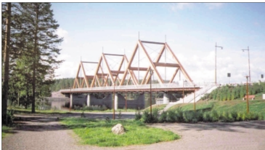
Fig 1. A glulam traffic bridge in Finland
