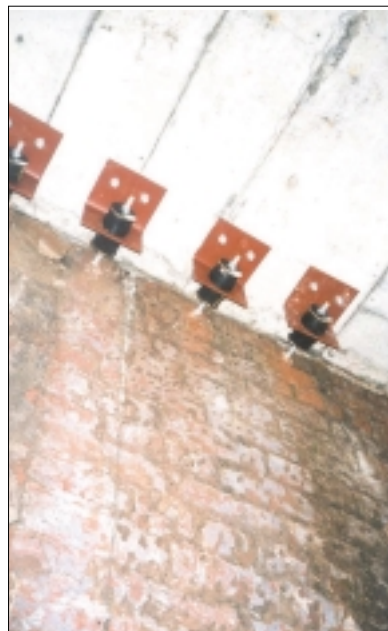
Right: The installation of acoustic bearings in the connections between the façades and the new structure at Oxford Circus, Manchester
