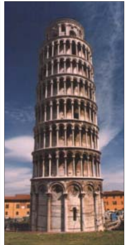
Fig 1. The leaning tower of Pisa
