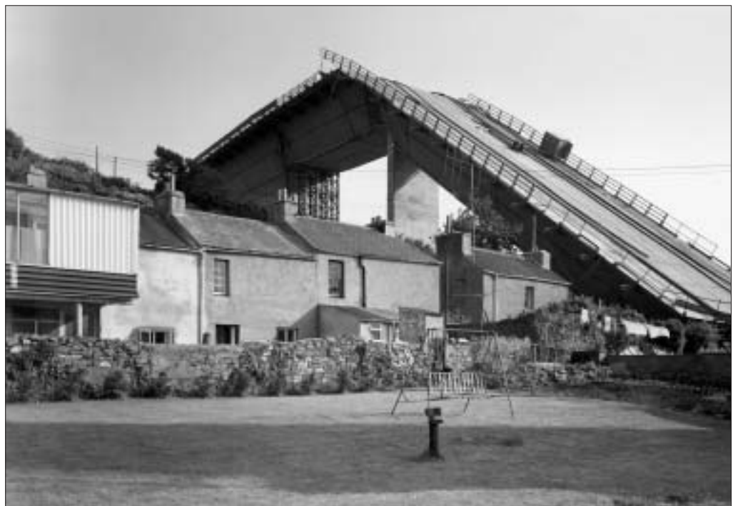
Fig 2. Milford Haven collapse
