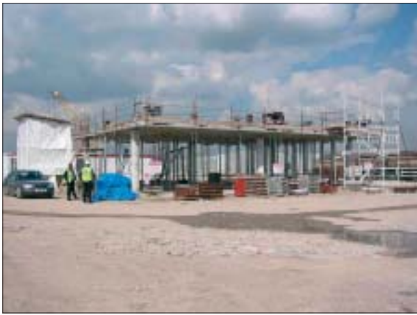
Fig 2. Post-tensioned slab at Laing O'Rourke's yard prior to hole cutting tests
