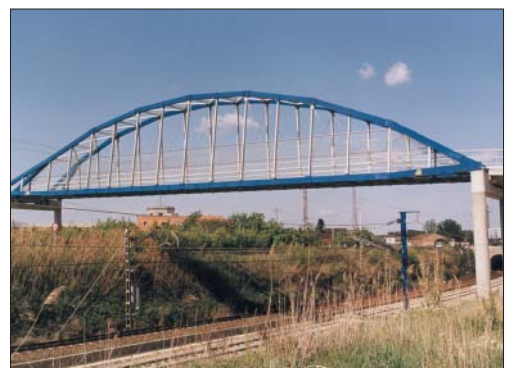
Below right: The composite pedestrian bridge in Lleida, Spain, is with its free span of 38m the longest of its kind in Europe. The bridge is made of structural profiles from Fiberline Composites (photo: courtesy Fiberline Composites)
