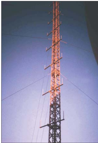
Pultruded FRP 50m mast supported by aramid guys (photo: courtesy Alan Dick & Co Ltd)
