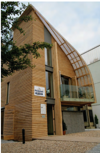
1 Kingspan Offsite Lighthouse built to the Code for Sustainable Homes at the BRE Innovation Park (Photo courtesy BRE)
