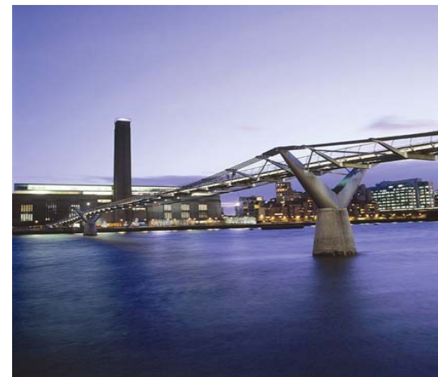
London Millennium Footbridge
