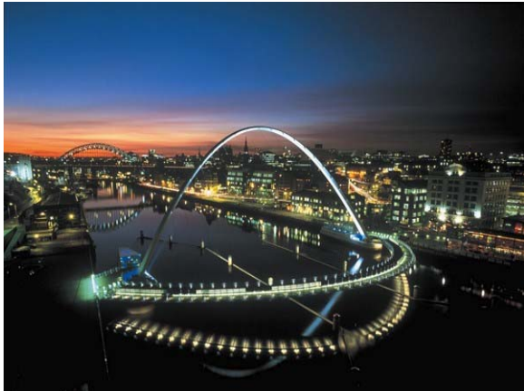
Gateshead Millennium Bridge
