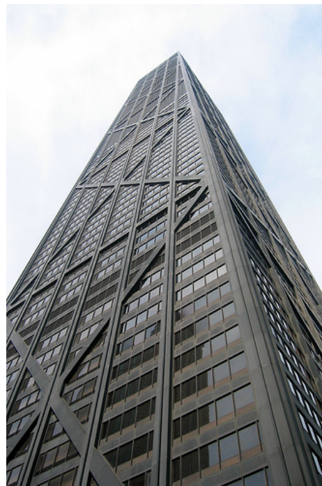
2. Fazlur Khan's revolutionary tubular bracing. Similar designs have been adopted on skyscrapers throughout the world
