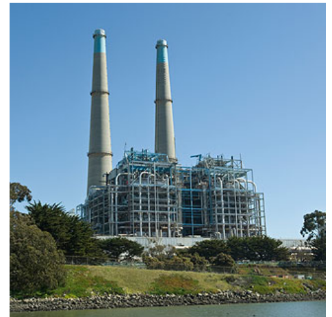
8. Moss Landing Power Station, California. Where Celtra are running their pilot scheme
