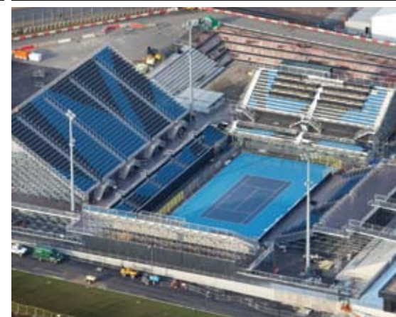
Figure 8 2012 Paralympic tennis stand (temporary structure)
