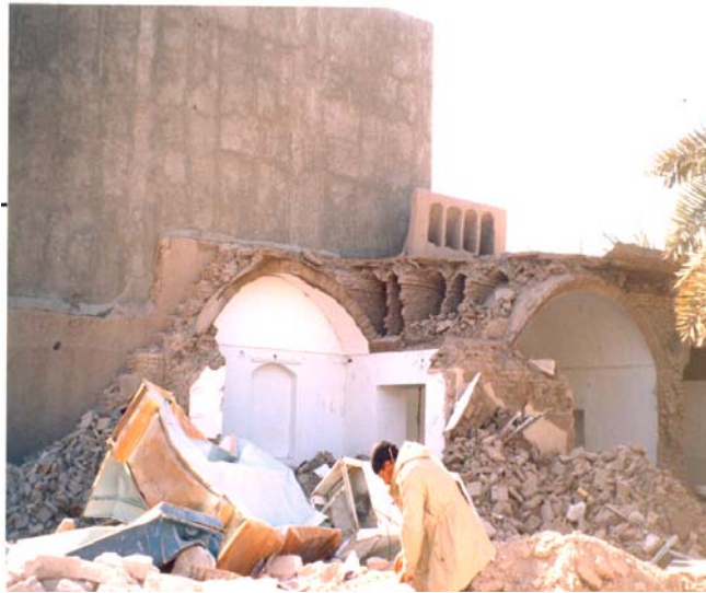
Photograph 3: This adobe's roof collapsed after the displacement and failure of its walls. Incidentally, the traditional form of air conditioning on the roof (wind-catchers) insulated the heat.
