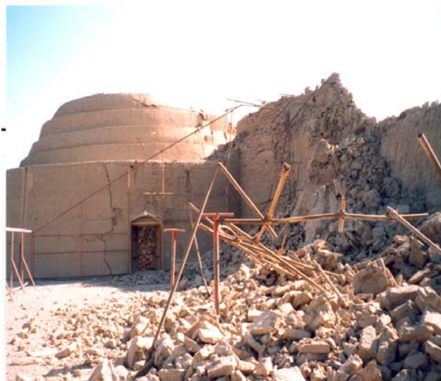
Photograph 28: Southern elevation of the Ice House, after the earthquake. The dome was reconstructed between 1974 and 2003, the original earthen walls survived the seismic forces (9EMS) with a vertical crack near the entrance in spite of the additional loading from the dome
