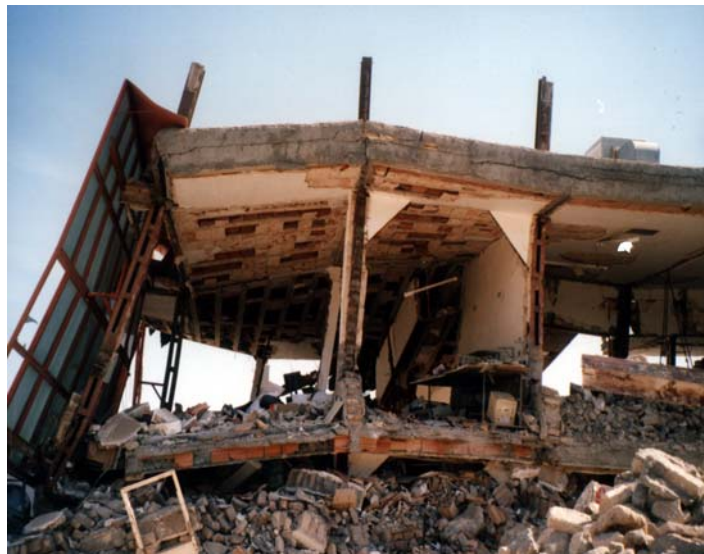
Photograph 16: The batten column at front elevation of this two storey commercial building buckled about its hollow axis.
