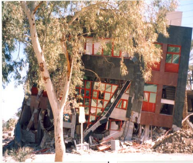
Photograph 11: Western elevation of Kimya building with the 3 rd and 4 th floors displaced about 4m towards west in to the pavement
