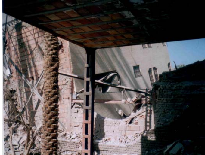
Photograph 15: View of south-east corner of Kimia building 4m displaced from inside the undamaged neighbouring building under construction where the floor has cross ribs every 2m and the battens on the columns are spaced at 300mm c-c compared to 500mm c-c in the next photograph
