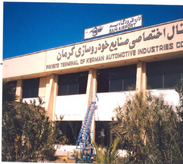
Photograph 30: The airport's control tower collapsed, non structural brick infill panels between the columns acted as shear walls when exposed to intensity of 8 EMS
