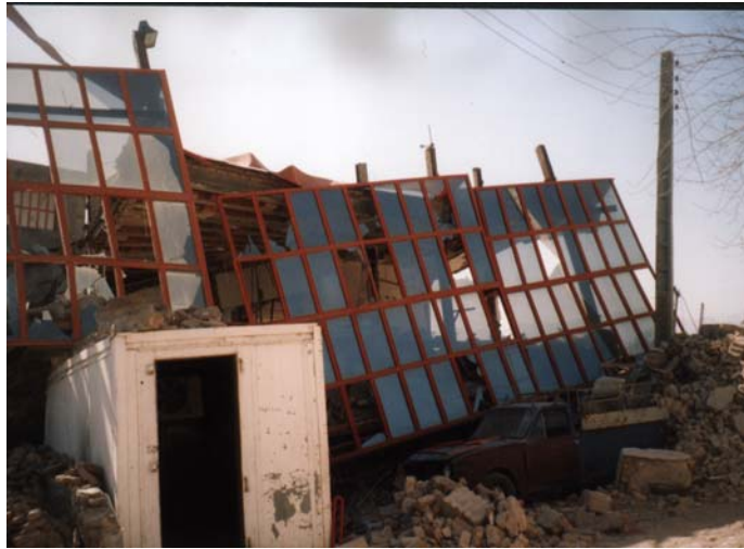
Photograph 17: The cladding of the building in the previous picture separated from the front elevation after the front batten columns buckled
