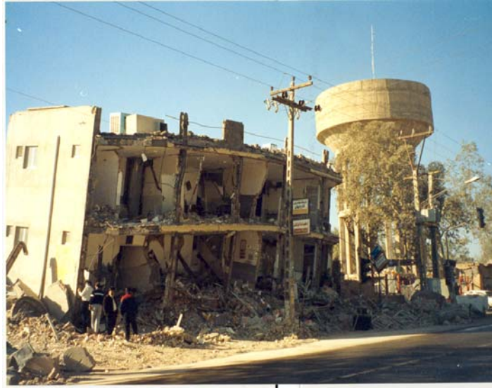
Photograph 19: Buildings surrounding the water tower were severely damaged.
