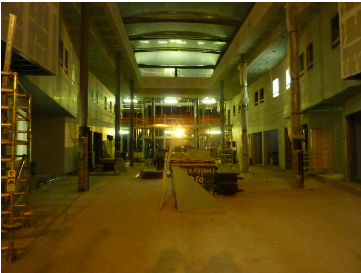
Main Corridor showing inflated roof
