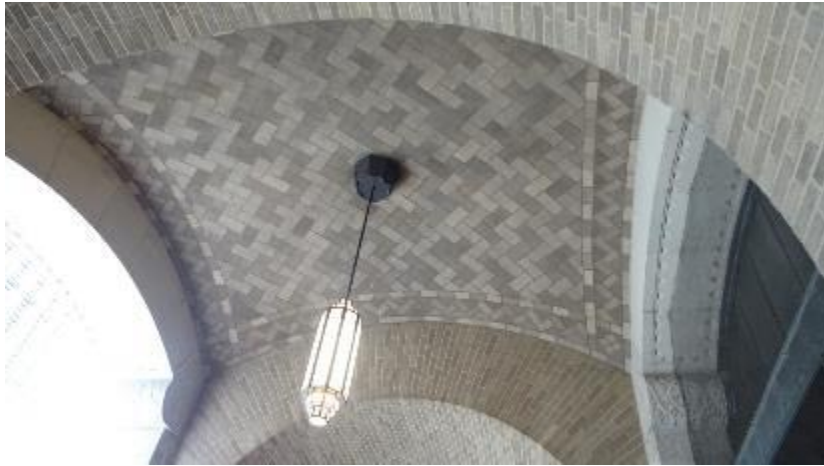
Figure 2.18 - Guastavino vaulted walkway in a building in Vesey Street New York City. This structure is directly opposite to the World Trade Centre and survived the impact from debris during the collapse of the twin towers in September 2001.
