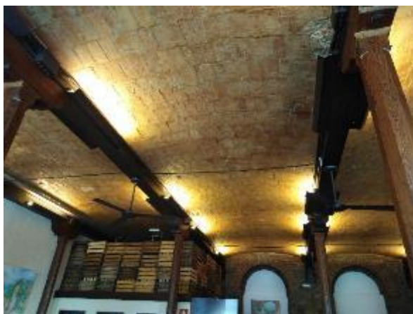
Figure 2.27 - Steel rods taking the horizontal thrust of Catalan vaults in a restaurant in Vilassar de Dalt.
