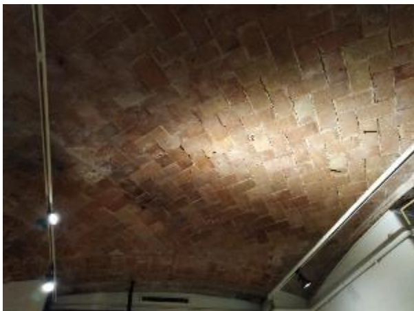
Figure 2.9 - Catalan vaulted roof of the Restaurant en Ville, Barcelona designed by Rafael Guastavino. The image on the left is an early example of the herringbone pattern being used in doubly curved Catalan vaults.
