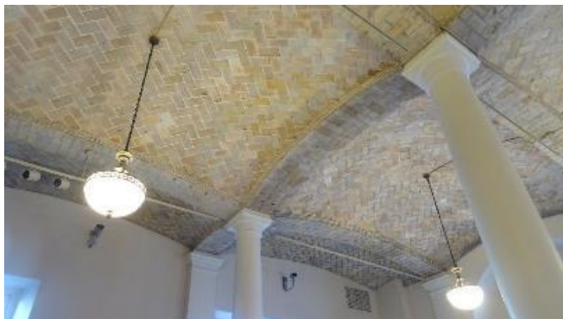
Figure 2.11 - Guastavino vaulted (Catalan vaulting) ceiling/ slab system in Boston Public Library.
