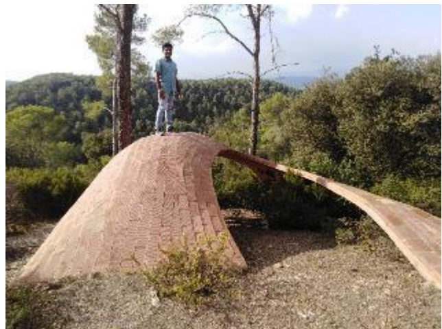
Figure 2.5 - Free-form Catalan vaulted structure built at Valldaura Labs, Barcelona
