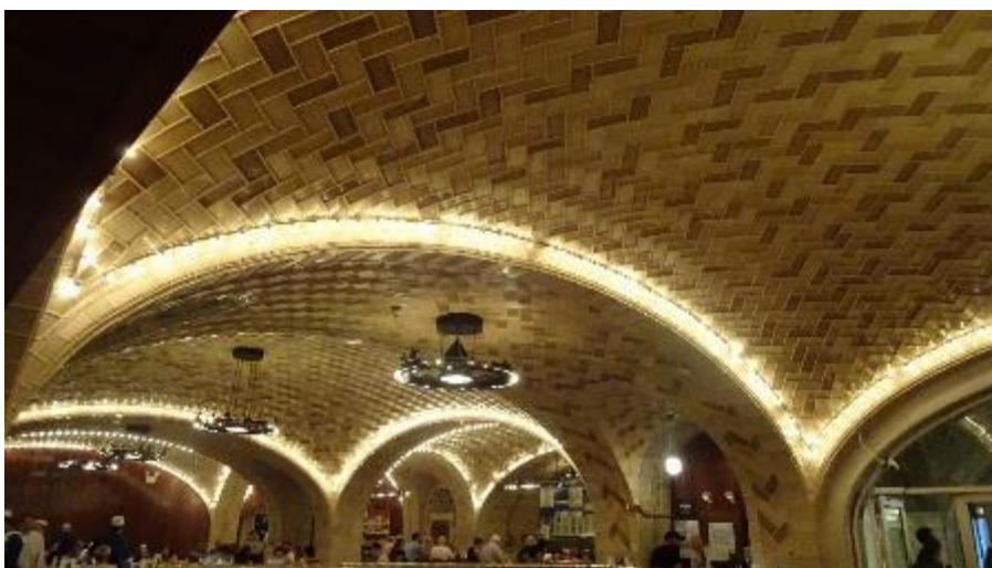
Figure 2.17 - Guastavino vaulted ceiling at the Oyster Bar in the Grand Central Station. This survived a major fire in 1997 with delamination of some tiles being the only damage caused.
