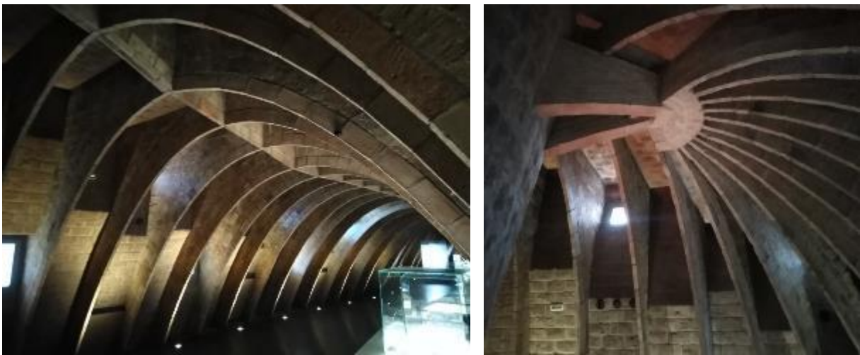
Figure 2.22 - Ribbed and vaulted roof structure at the attic of Casa Milà, designed by Antonio Gaudi.
