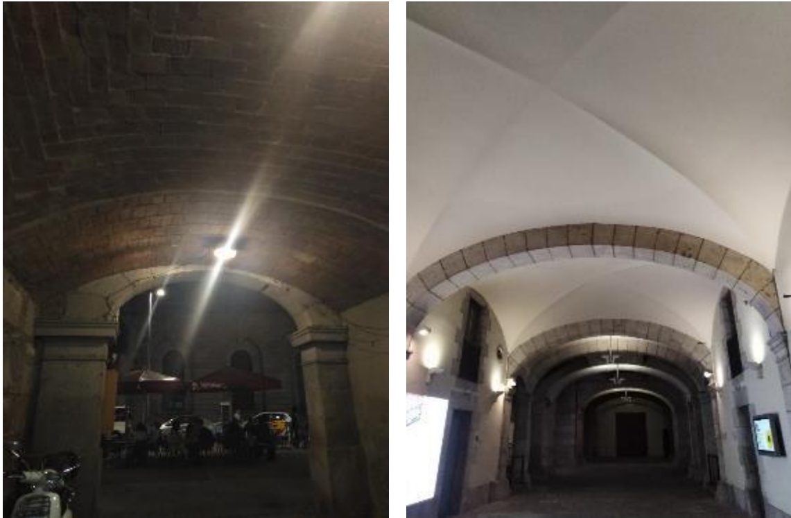
Figure 2.10 - Exposed and unexposed vaulted ceiling / floors around the city of Barcelona.
