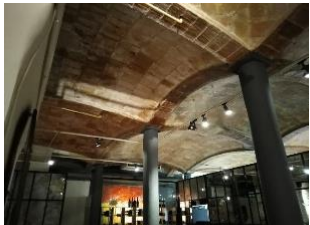
Figure 2.9 - Catalan vaulted roof of the Restaurant en Ville, Barcelona designed by Rafael Guastavino. The image on the left is an early example of the herringbone pattern being used in doubly curved Catalan vaults.
