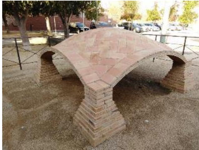
Figure 2.25 - A prototype of doubly curved Catalan vault built in front of Teatre La Massa in Vilassar de Dalt, Barcelona
