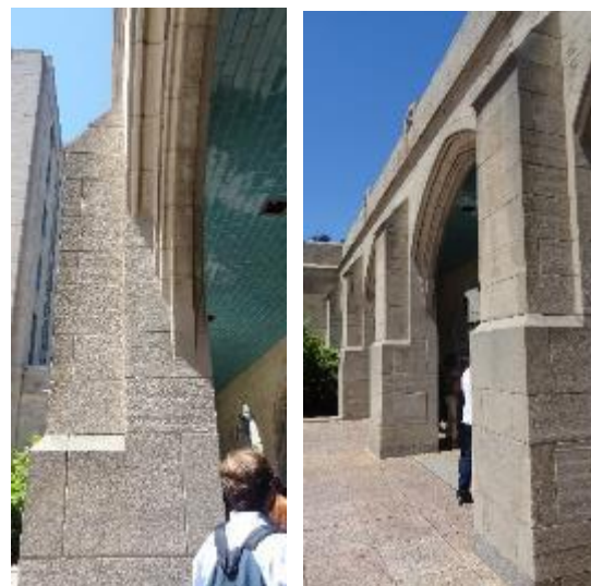
Figure 2.28 - Making use of buttressing to resist the horizontal thrust (in absence of tie rods) of Catalan vaulted structure, at University of Massachusetts.
