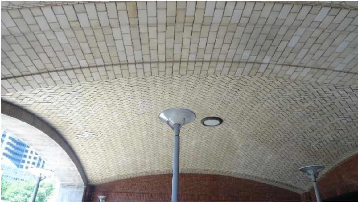
Figure 2.12 - Guastavino vaulted ceiling at the patio of the Boston Coast Guards office.
