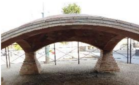
Figure 2.4 - Multiple layers of thin tiles in Catalan vaults.
