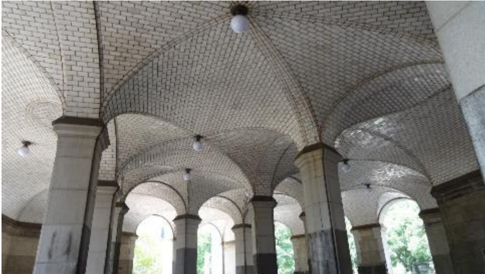
Figure 2.15 - Guastavino vaulted ceiling at New York Chamber Street City Hall Building.
