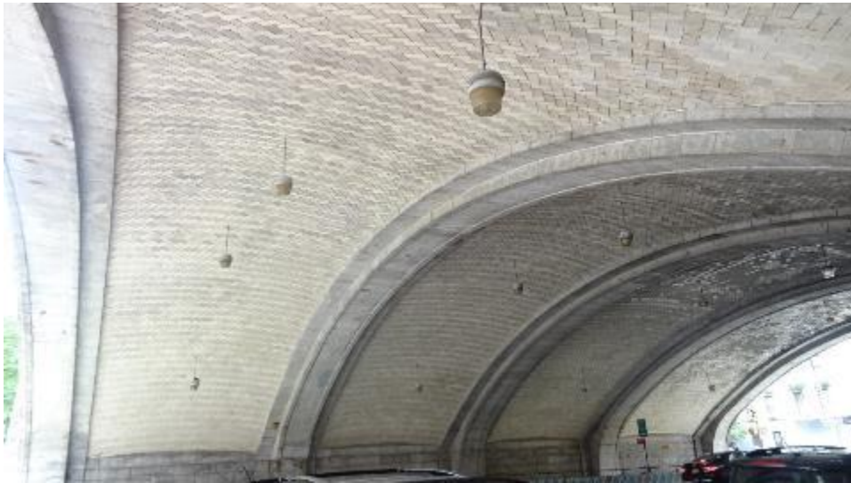
Figure 2.16 - Guastavino vaulting in the Queensboro Bridge, New York City.
