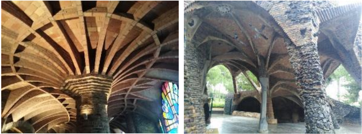
Figure 2.21 - Ribbed and vaulted roofs of Catalan tiles at the crypt in Colonia Güell, designed by Antonio Gaudi.
