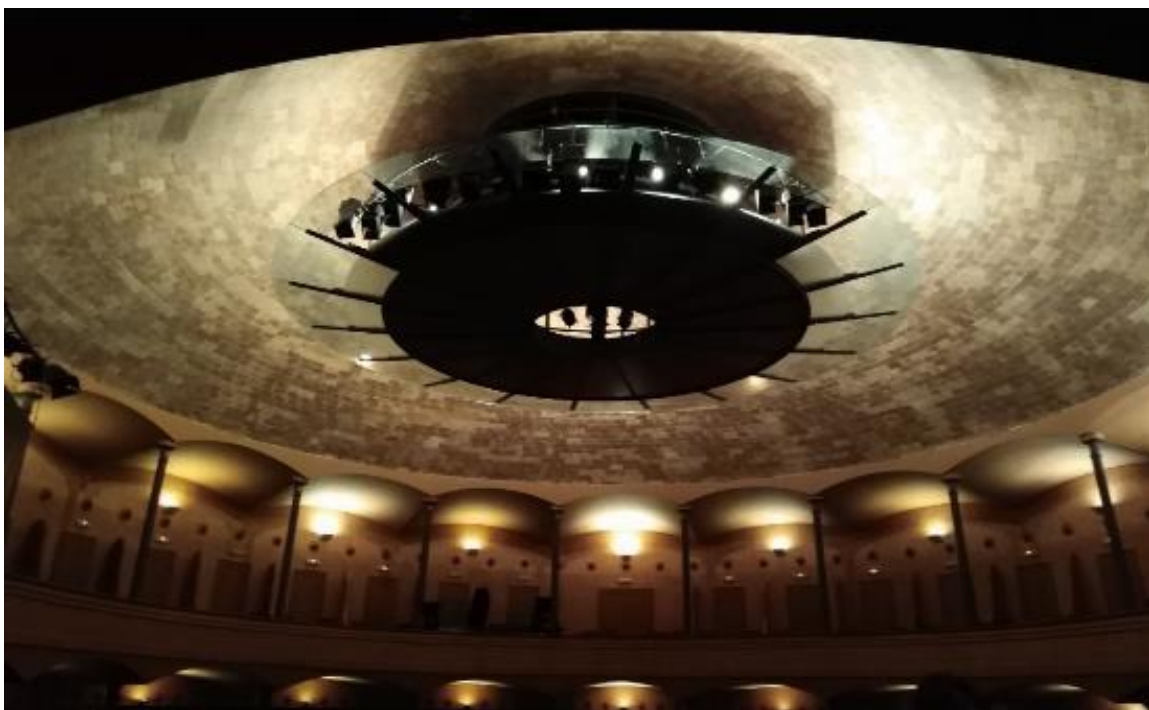
Figure 2.6 - The Catalan vaulted spherical dome of Teatre La Massa in Vilassar de Dalt, designed and built by Rafael Guastavino.
