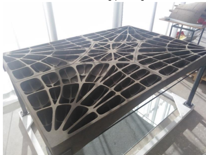
Figure 4.12 - 3D printed slab system developed at BRG.
