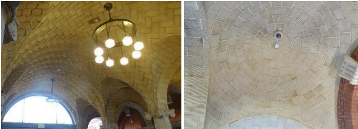
Figure 2.13 - Guastavino vaulted ceilings at the Fariborz Masseh hall at MIT.
