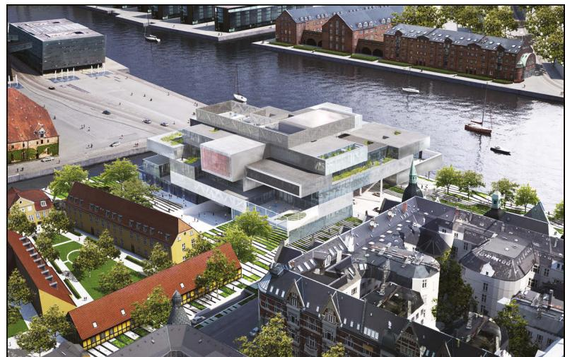
Bryghusprojektet, Copenhagen. Image courtesy of OMA. Arup carried out embodied carbon calculations as part of a broad response to the client's sustainability objectives. The team used those calculations to set a carbon target for the next stage of the design. This approach has ensured that the significant elements for this particular project have been identified and can now be targeted.
