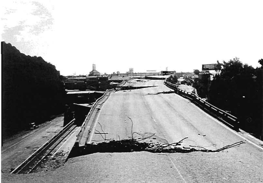
**Plate 5.1 : Cypress Street Viaduct - Looking South along collapsed deck**
