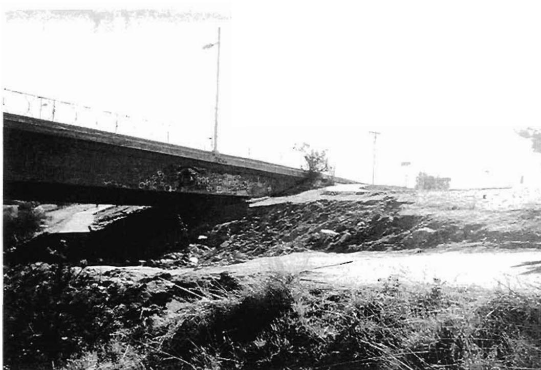
**Plate 5.12 : Laurel Street Bridge - Slumping of embankment**
