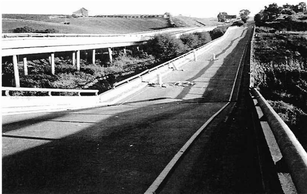
**Plate 5.23 : Struve Slough Bridge - Piles punched through deck slab**
