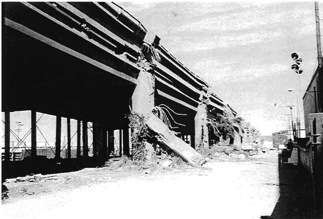
**Plate 5.2 : Cypress Street Viaduct - General view of collapsed viaduct**
