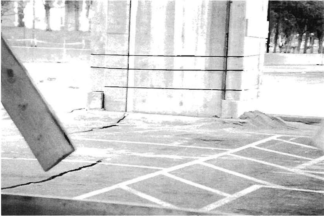
**Plate 7.6 : Liquefaction around pile cap on the Embarcadero**
