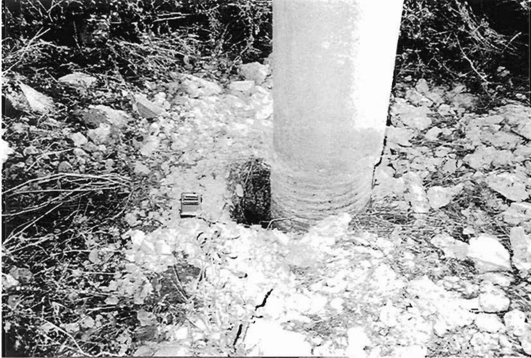
**Plate 5.24 : Struve Slough Bridge - Crushed concrete from pile/deck joint above postholing around pile**
