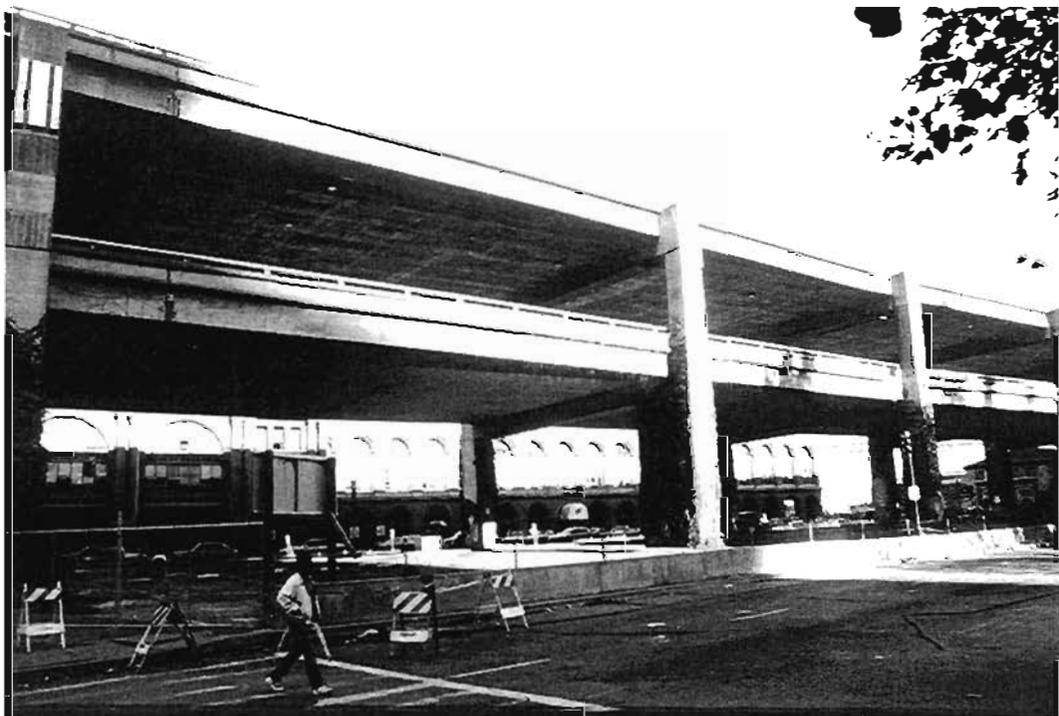
**Plate 5.6 : Embarcadero Viaduct - Cable restrainers (under metal covers at top left hand corner)**
