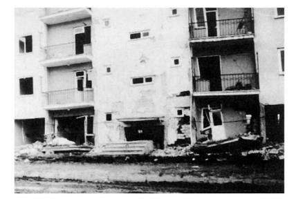
Plate 4.8 Bottom-top collapse, starting from ground floor level, with all the floors above surviving. Notice the detached entrance staircase.
