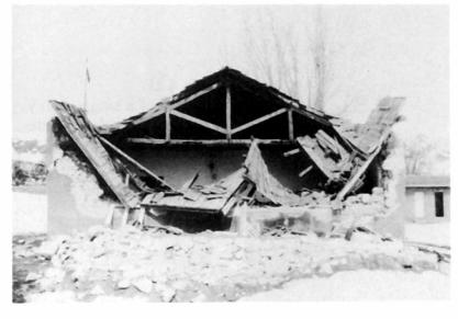
Plate 4.18 Roof collapse of a single storey stone masonry school building. *Location: Mecediyeh.*
