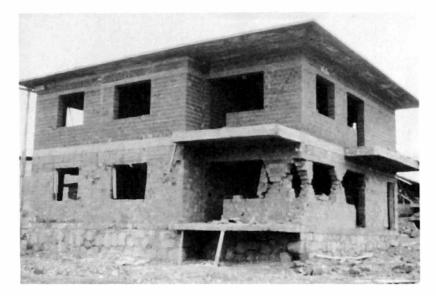
Plate 5.24 Cooperative Housing Estate, Uzumlu. House no. 21. Severe damage at the ground floor corner.
