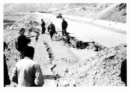
Plate 4.31 Failure of road embankment near Eksisu.
