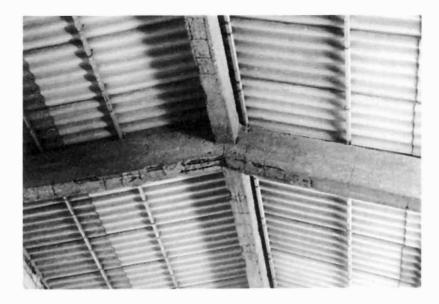
Roof of cattle shed at meat processing plant. Insufficient cover and poor compaction has resulted in corrosion of the reinforcement. Other sections of this roof collapsed completely (see Plate 4.22).
