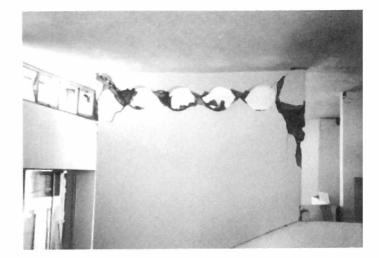
▲ Plate 5.19 City centre. Failure induced by openings in reinforced concrete wall. *Location 17*.
