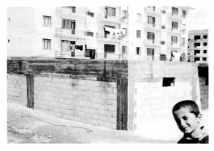
Plate 5.33 Concrete block infill at semi-basement level in apartment under construction. *Location 18*.
