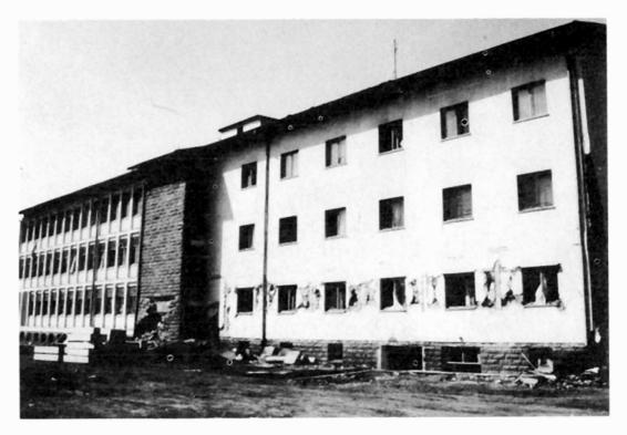
Operations clinic, state hospital, northern façade. Notice the identical location of damage to the infill walls at ground floor level. *Location 14*.
