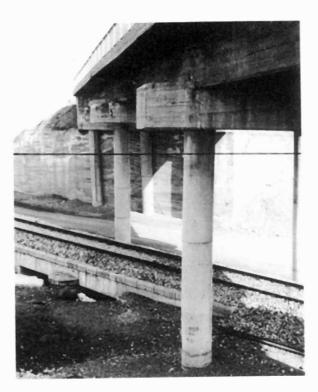
Badly damaged highway bridge on road to Kemah. Notice the lack of bearings between the crossheads and main beams. The nearest column is badly bent.
