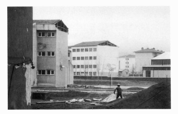
Plate 4.24 Failure of unrestrained gable ends. Location 10.
