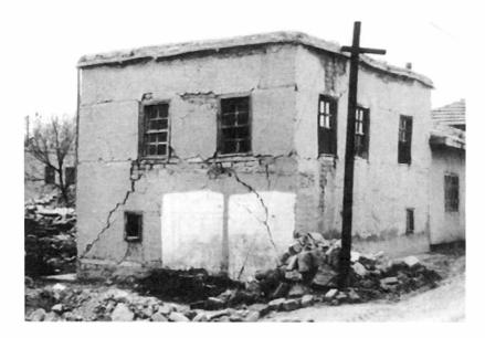
Plate 4.19 Traditional adobe house reinforced by timber hatils at the top and bottom of the windows. *Location: Altinbasak.*
