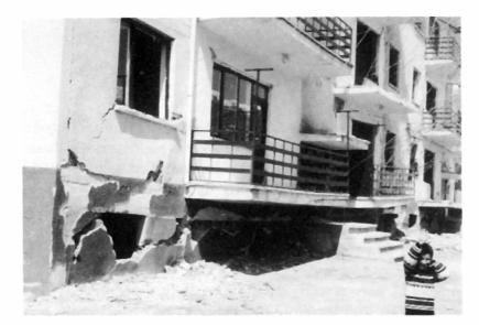
Plate 5.31 Weak storey failure in recent apartment block. Location 18.
