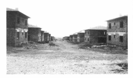
General view of the Cooperative Housing Estate, Uzumlu, looking southwards from the top of the estate. Notice that the first few houses, whose roofs are already finished, are completely undamaged. The significant slope of the site is also visible. The collapsed buildings are at the bottom of the estate, presumably in deeper soil.
