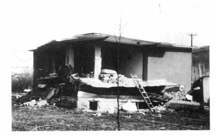
Plate 4.16 Collapsed two storey RC frame with basement and ground floor used for storage, without most of the infill. Location: Çukurkuyu.
