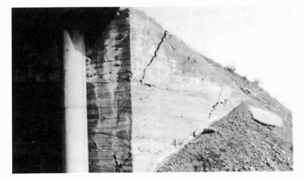
Plate 4.27 Severe cracking of embankment wall of the same bridge.
