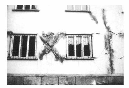
Plate 4.7 Poorly repaired structure, the original damage probably caused by 1983 earthquake. *Location 4*.
