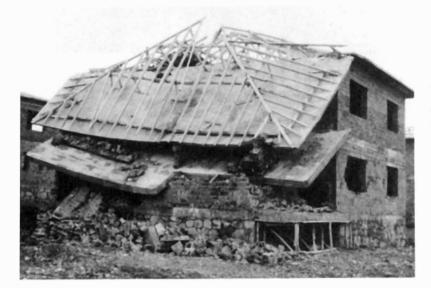
Plate 5.26 Cooperative Housing Estate, Uzumlu. House no. 14. Collapse of both floors (only in the western part).
