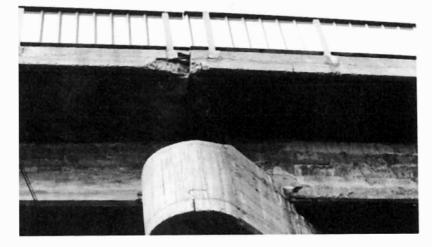
Plate 4.28 Detail of column head of the same bridge, showing poor construction quality and damage due to pounding between adjacent deck segments.
