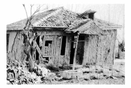
Severely damaged himis house. Two single storey concrete block masonry houses next to it collapsed. *Location: Calabzur*.
