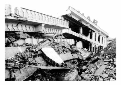
Bottom-top collapse of four storey RC frame with double basement. The structure has split at a movement joint, with the near half suffering a complete pancake collapse, while in the other half the top two storeys have survived. Location 5.
