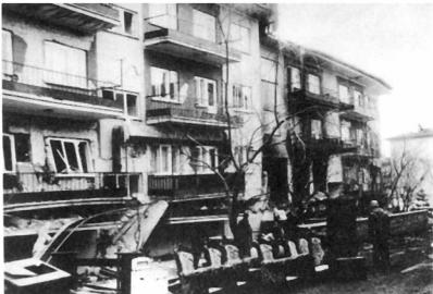
Plate 4.10 Mid-storey collapse of a five storey apartment building.
