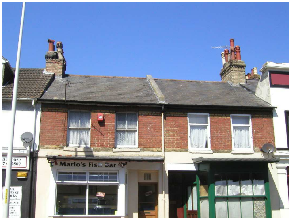
Figure 4: Similar chimneys damaged to different extents at two ends of same building on Black Bull Road.
