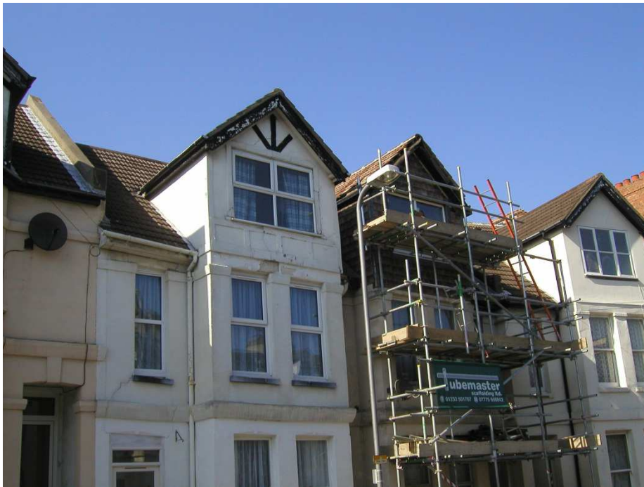
Figure 10: Broadmead Road. Structural cracking and cracking of render in the façade of a three storey house.
