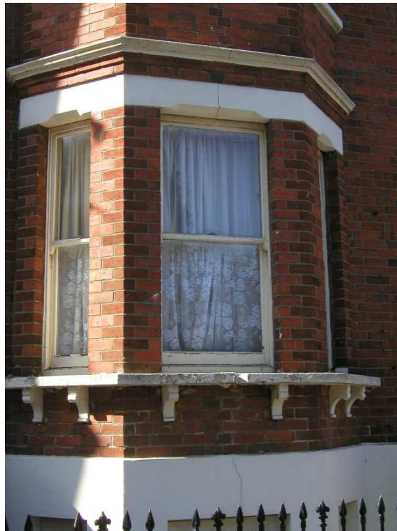
Figure 11: Broadmead Road. Vertical cracks in lintels, window sill and wall.
