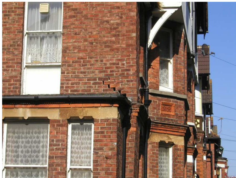
Figure 12: Broadmead Road. Large crack in the external wall of a house.
