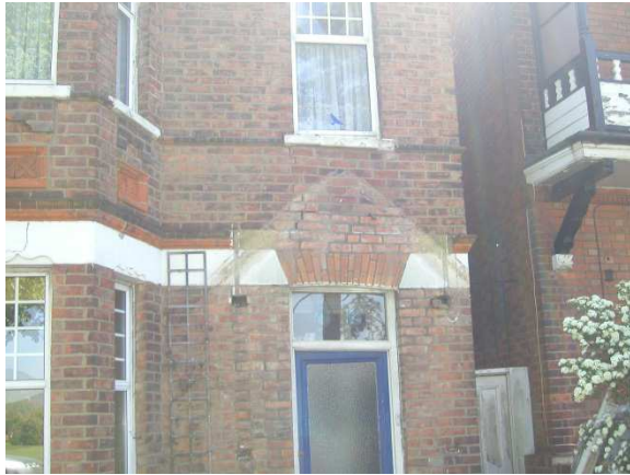
Figure 9: Light structural damage in a house on Radnor Park Road. First floor window sill is tilted, structural vertical crack to door, crack in ground floor lintel, detachment of wooden portico and significant chimney damage.
