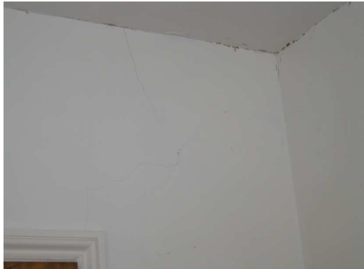
Figure: 8. Examples of hairline cracks in plaster observed within a house on Linden Road (right). External view of the property (left).
