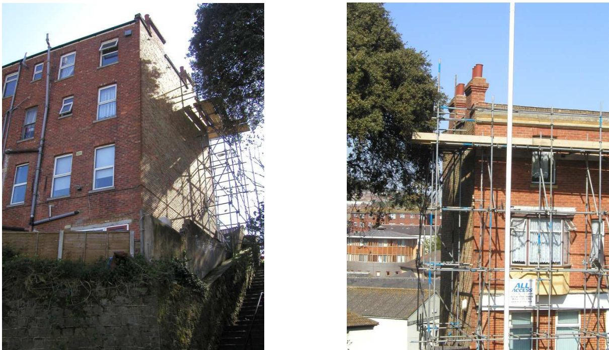
Figure 16: Moderately damaged building on Grace Hill.
