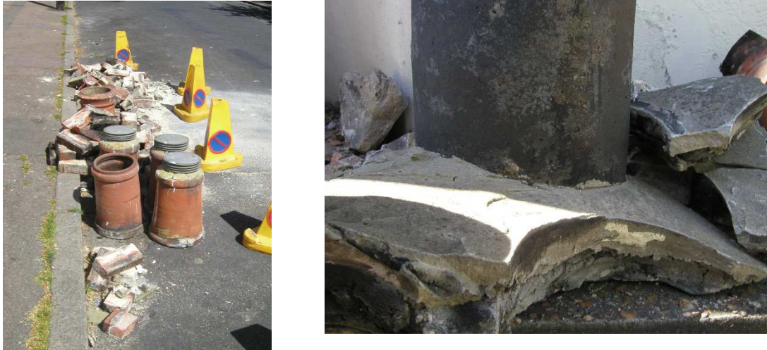
Figure 3: Examples of typical clay chimney pots (left) and the mortar build-up for chimney pots (right).
