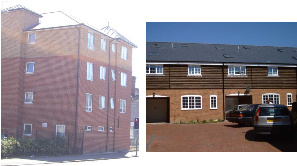
Figure 17: Examples of modern brick buildings with no damage. (left: building located at the junction of Park Farm road and Pavilion road, right: Pavilion Road).
