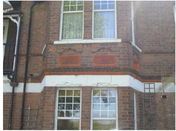
Figure 9: Light structural damage in a house on Radnor Park Road. First floor window sill is tilted, structural vertical crack to door, crack in ground floor lintel, detachment of wooden portico and significant chimney damage.
