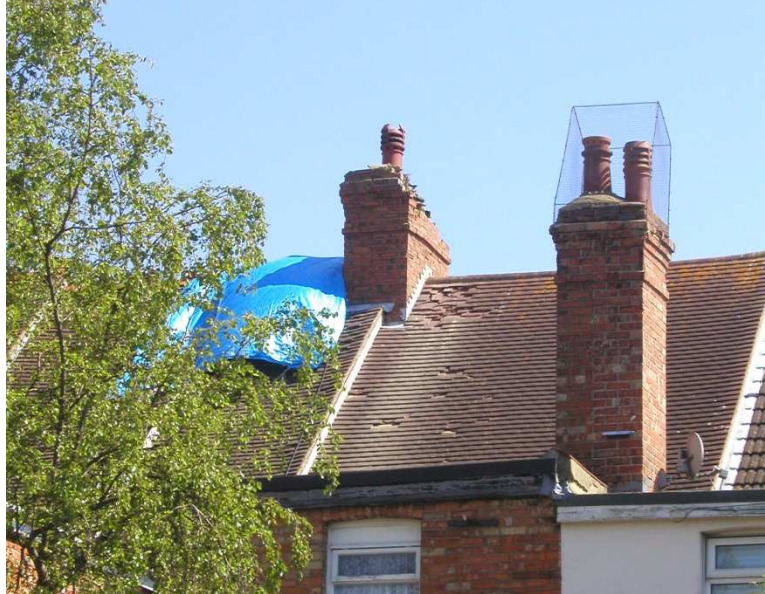
Figure 5: Park Farm Road. Chimney damage causing secondary damage to the roof.
