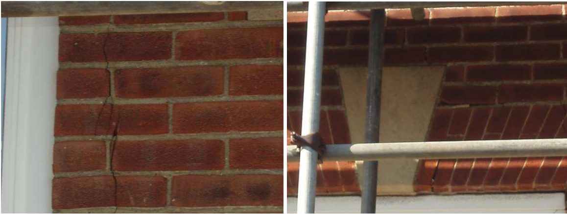
Figure 15: Cracks in western façade of Harvey Grammar School. Photos care of Neena Saith and Torolf Hamm of Risk Management Solutions.
