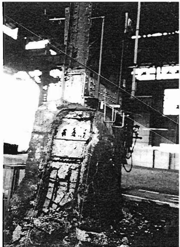
Plate 4.175: As 4.174 but severely corroded
