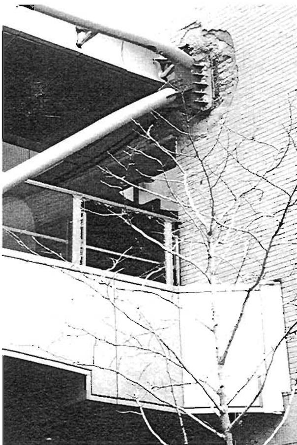
Plate 4.145: Connection damage between new buildings
