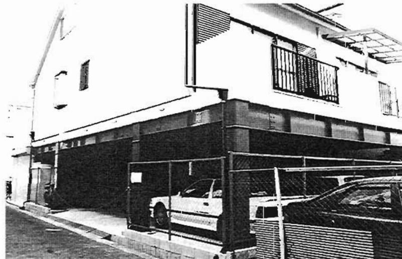
Plate 4.104: House with ground floor moment resisting frame
