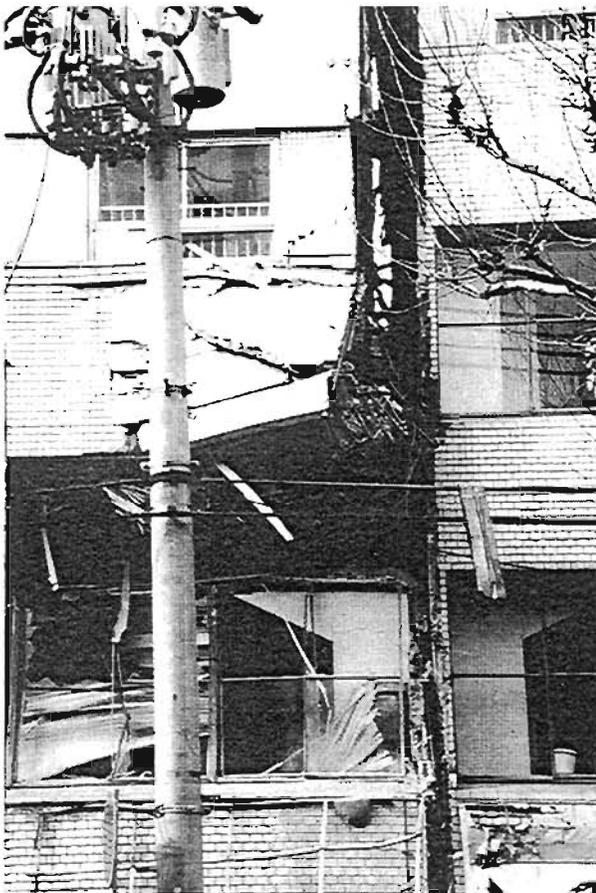
Plate 4.156: Column damage due to buffeting
