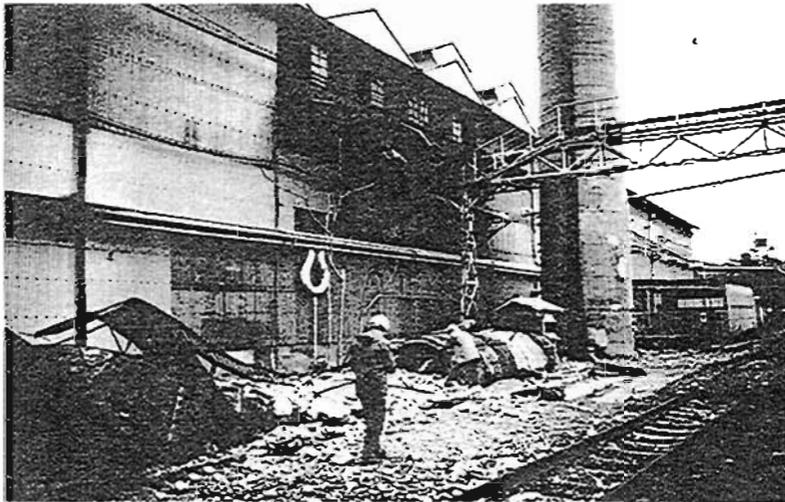
Plate 7.33 RC stack at old steelworks, top section fallen
