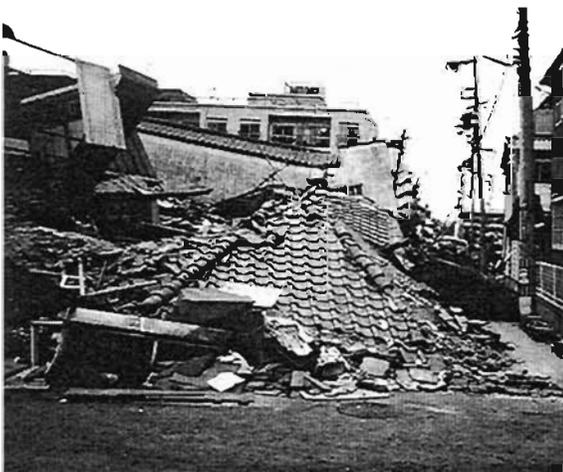
Plate 4.99: Collapse with roof intact
