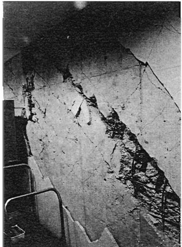
Plate 4.37: Shattered shear wall
