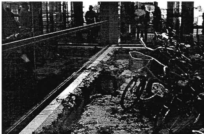
Plate 8.6: Liquefaction settlement observed at the KCAT Ferry Terminal, Port Island
