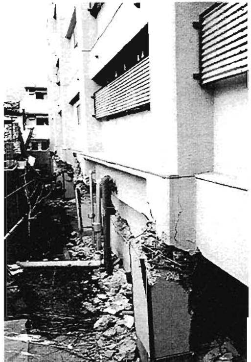
Plate 4.58: Severed shear wall
