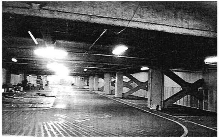
Plate 4.132: Internal bracing of the Diamaru
