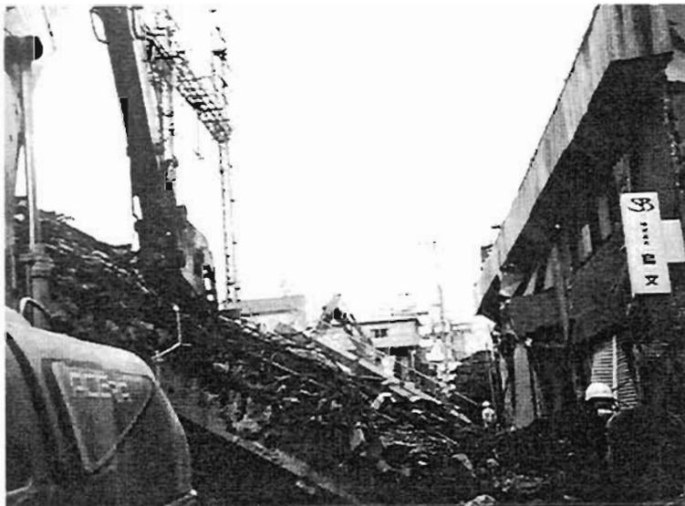
Plate 4.159: Collapse of viaduct span due to building restraint
