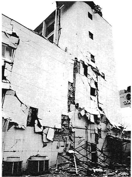
Plate 4.40: Damage at root of tower
