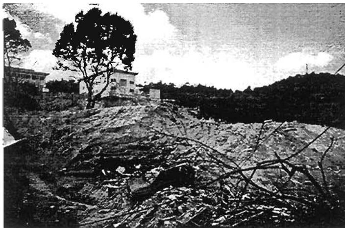
Plate 8.39: Earthquake induced landslide observed at Nikawa, Nishinomiya
