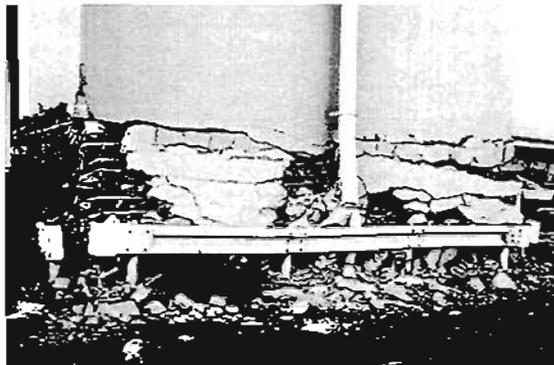
**Plate 6.41** Pier on East Approach to the Maya Ohashi Bridge on the Harbour Highway close-up of pier in centre of Plate 6.40 - this is the second pier from the east main pier, and suffered severe damage in accommodating the distortion at the main bridge pier.
