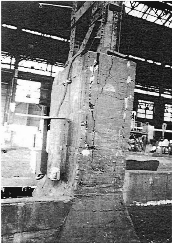
Plate 4.174: Cracked encased base of lattice column
