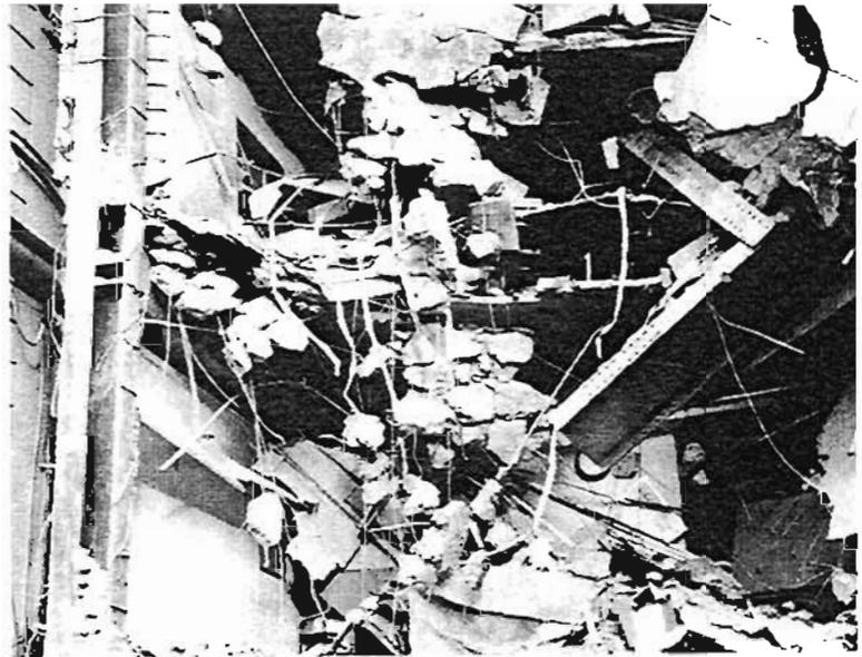
Plate 4.75: Building with failed welds at beam/column connections
