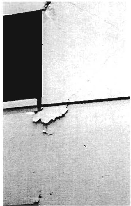
Plate 4.123: Cracking at ends of connecting
