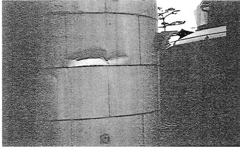
Plate 7.16 Buckling in tank wall
