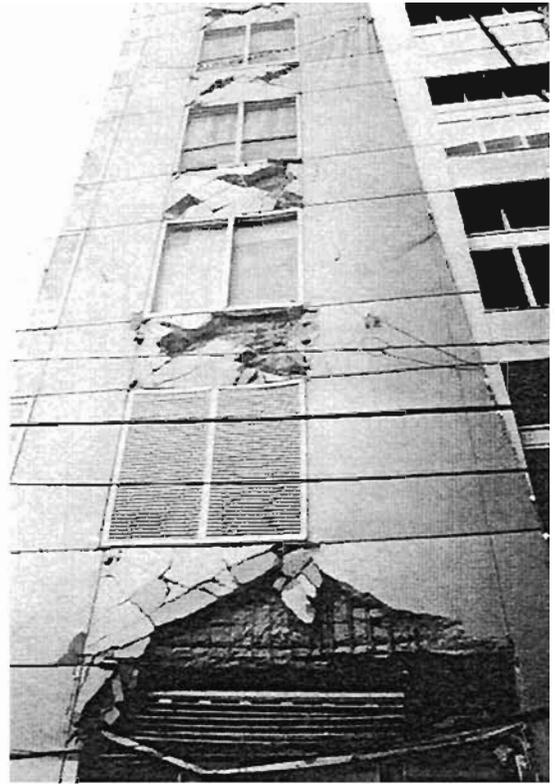
Plate 4.36: Damaged connection beams
