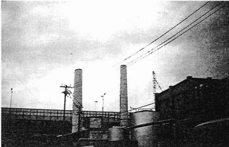
Plate 7.35 Two RC stacks, top sections fallen
