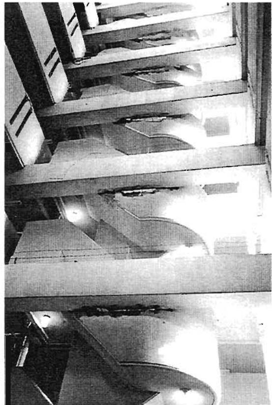
Plate 4.55: Spalling between staircase and stair well cross beam
