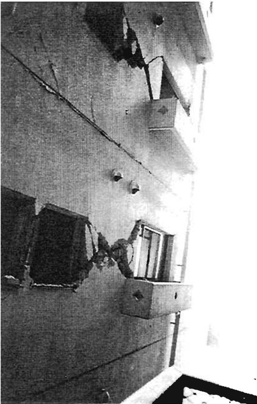
Plate 4.54: X-cracking in perforated shear walls
