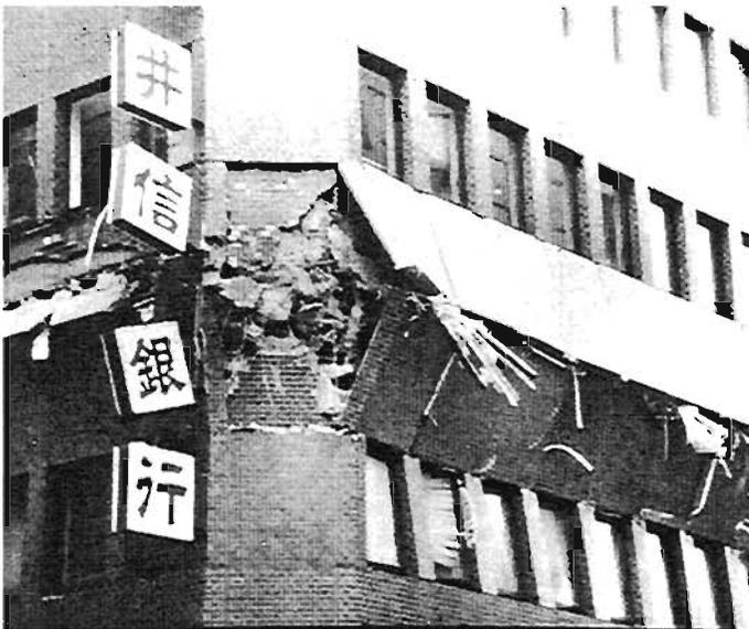
Plate 4.8: Bulging facade at corner where building dropped
