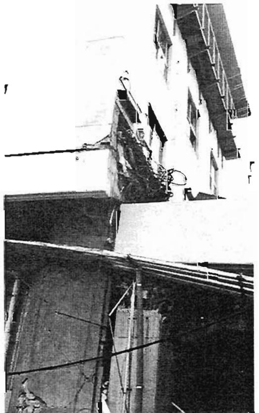
Plate 4.162: First floor column damage due to impact across expansion joint
