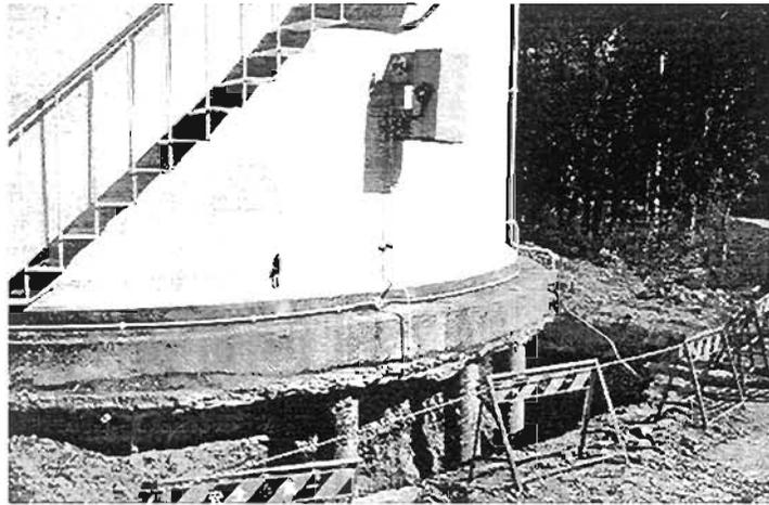
Plate 8.22: Excavated piles under a water tank at the Higashinada Power Station (Photo by C. Bolton)
