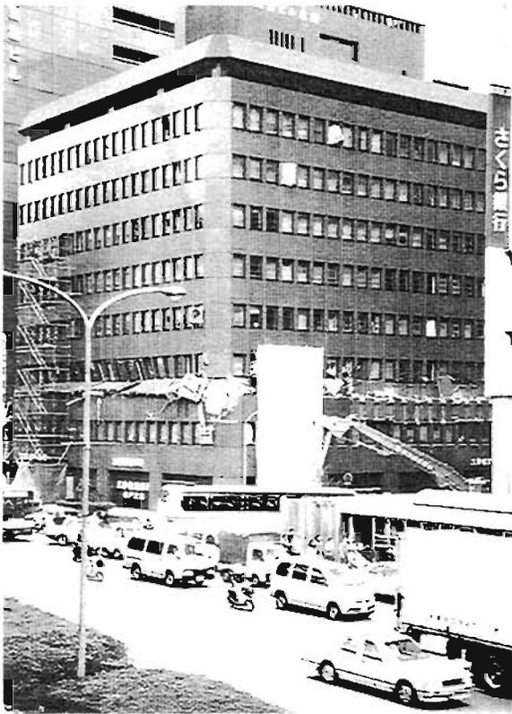
Plate 4.7: RC Building with collapse in 3rd storey
