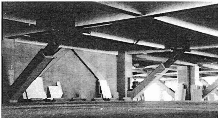
Plate 4.119: Internal bracing
