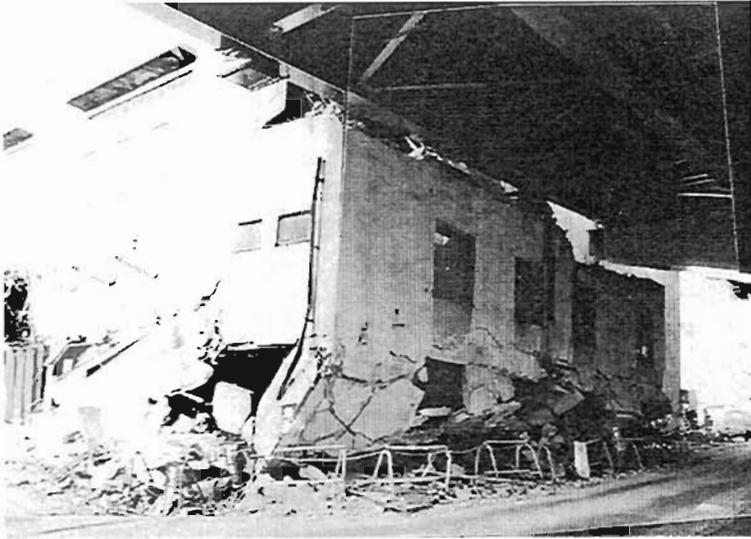
Plate 4.158: Substation collapsed against viaduct damaging viaduct
