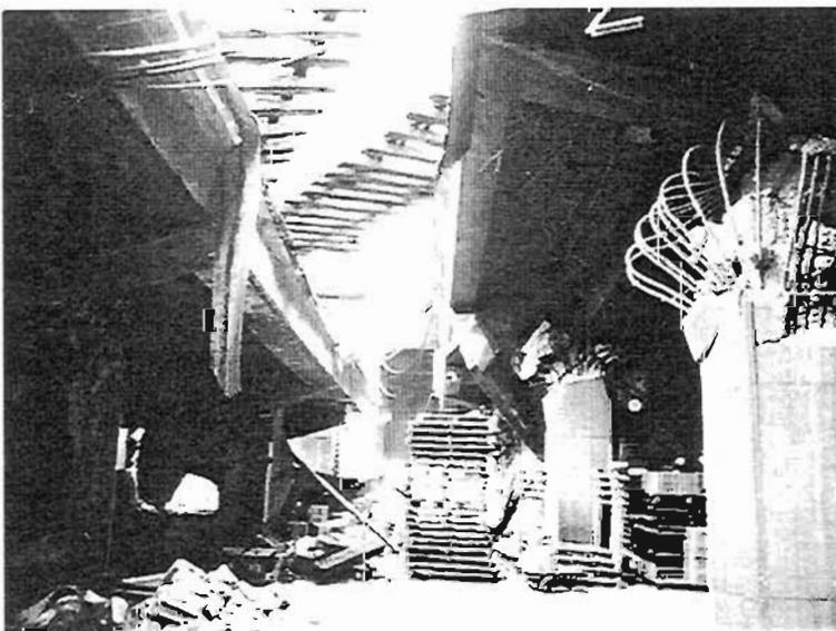
Plate 4.161: Collapsed infill slab due to buffeting between viaduct and warehouse
