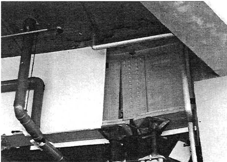
Plate 4.95: Rotated joint with rotation concentrated at span connection
