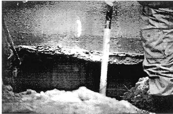
Plate 8.23: Hairline cracks observed in the piles of the water tank (photo by C. Bolton)
