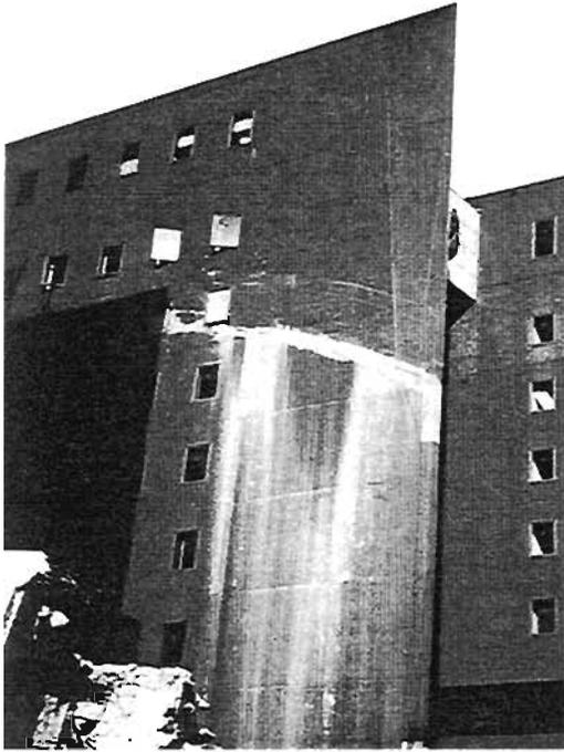
Plate 4.29: Substantial perforated shear wall building
