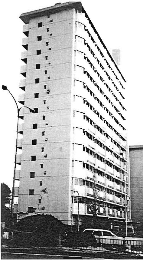
Plate 4.32: Shear wall compression failure with consequential shear fracture along vertical axis
