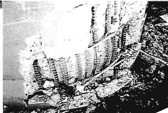
**Plate 6.30** Hanshin Expressway, Kobe: Large diameter column with small confining bars. Ends of bars hooked, but with tails not long enough to anchor into core concrete.
