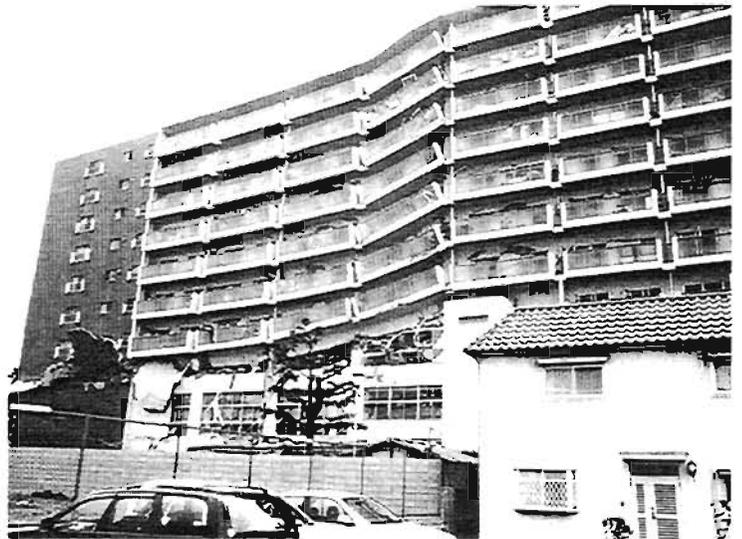
Plate 4.21: Partial storey collapse due to shear wall failure one end of building
