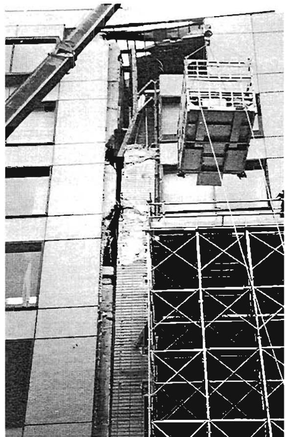
Plate 4.157: Buffeting damage in top storey
