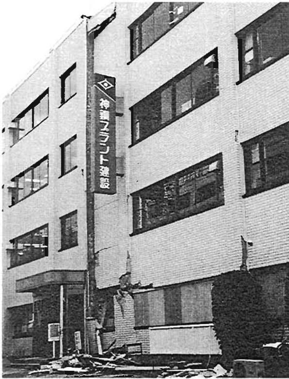
Plate 4.154: Impact damage between buildings of same height
