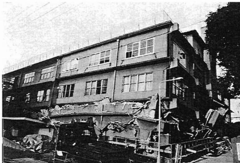
Plate 4.110: Precast concrete building with partial collapse induced by link bridge
