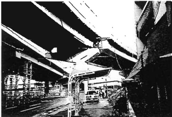
**Plate 6.9** Hanshin Expressway to the west of Kobe centre: Large sideways shift towards south of curved deck, same interchange as Plate 6.8
