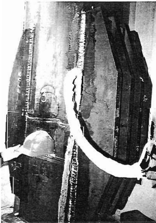
Plate 4.78: Fin strengthening at column fractures
