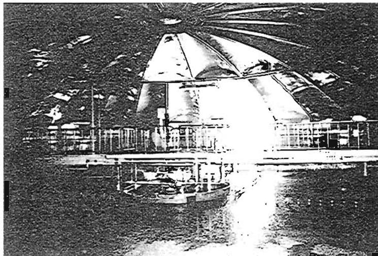
Plate 7.15 Glassfibre panel roof, internal view
