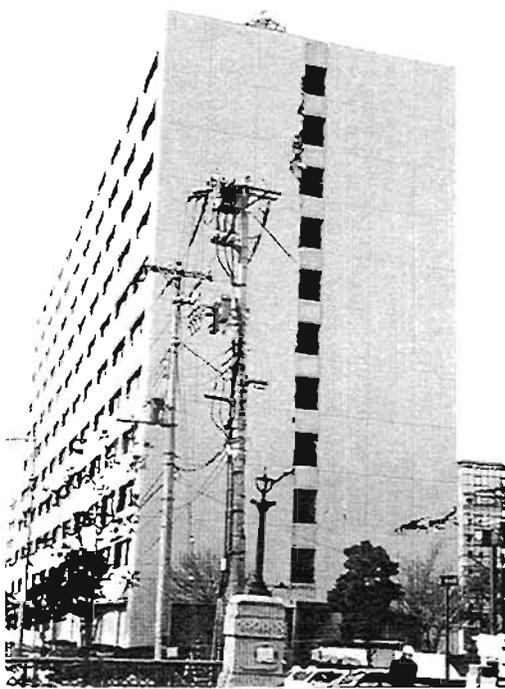
Plate 4.27: Coupled shear wall building
