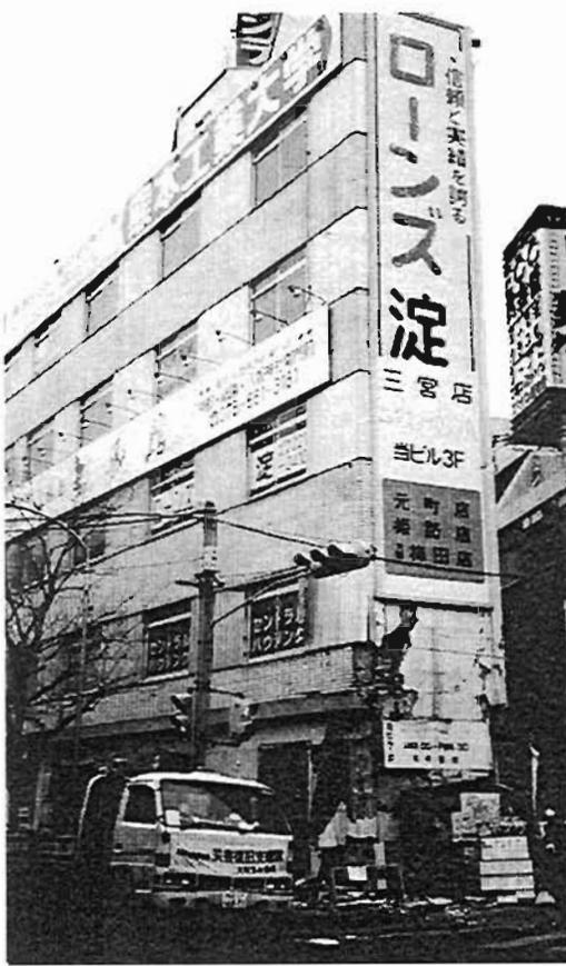
Plate 4.44: Damage at end of heavily tapered building
