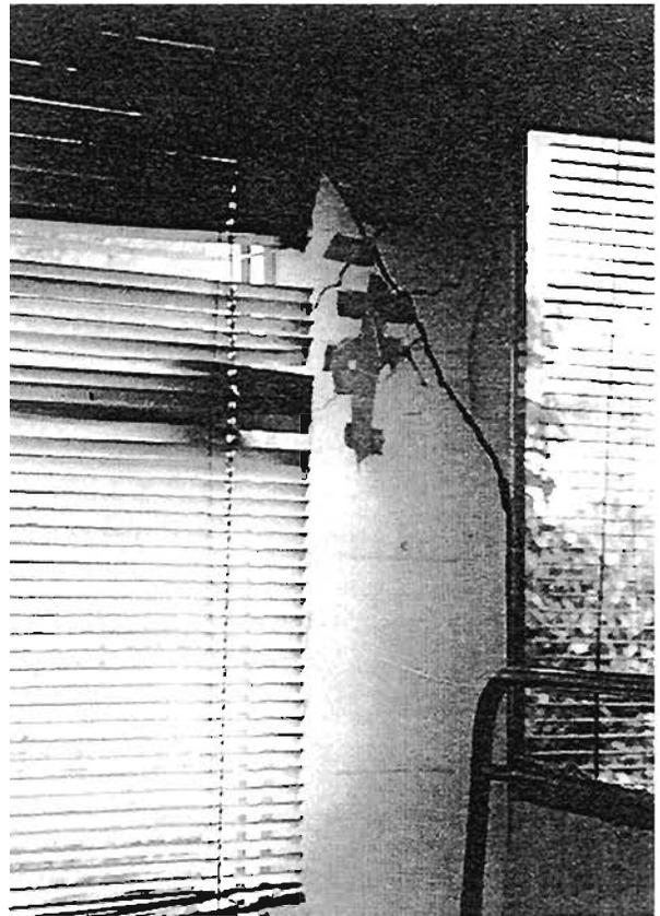
Plate 4.3: Internal RC column damage
