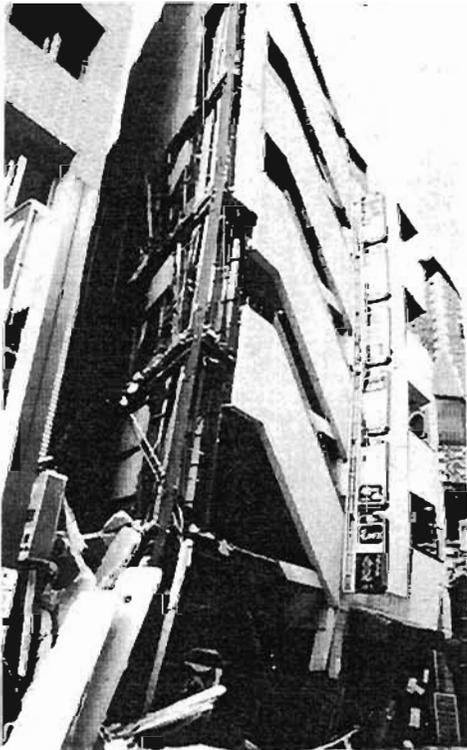
Plate 4.70: Sway after apparent failure
