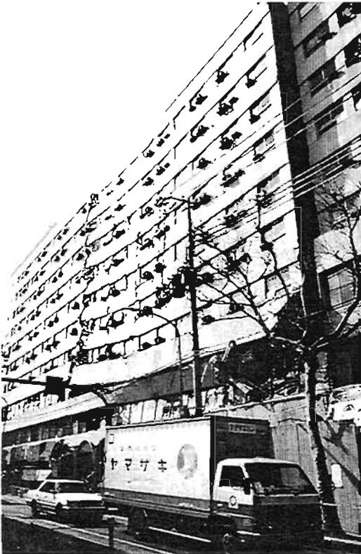
Plate 4.20: Partial storey collapse due to buffering
