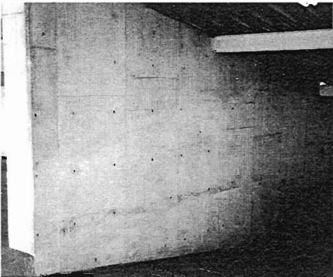
Plate 4.128: Repaired cracks in transverse wall
