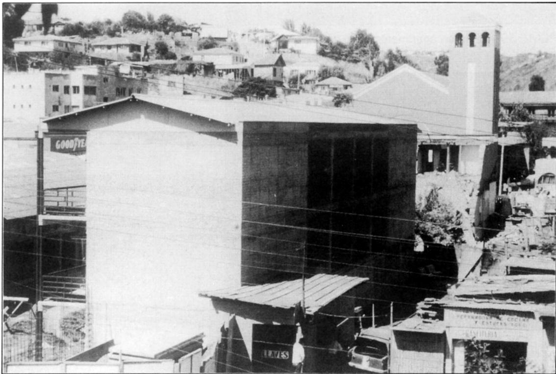
PLATE 5.6 Undamaged infill frame building on sloping ground, San Antonio
