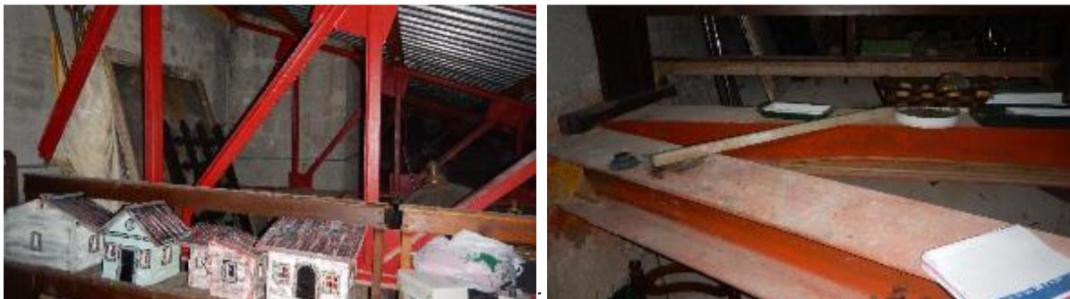
Figure 6-12 Portico steel structure: a) horizontal bracing and b) roof trusses.
