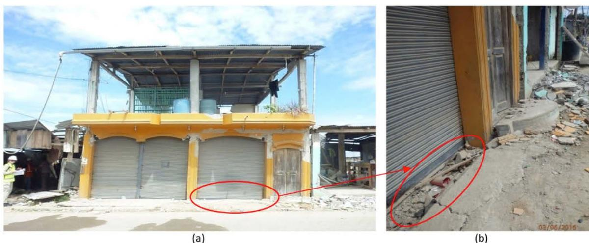
Figure 4-12 Settlement of building in Chamanga (a) increased settlement from left to right of structure (b) settlement relative to road and step.
