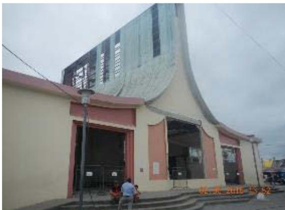
Figure 6-39 Pedernales Cathedral, with damage to the roof and masonry façade.
