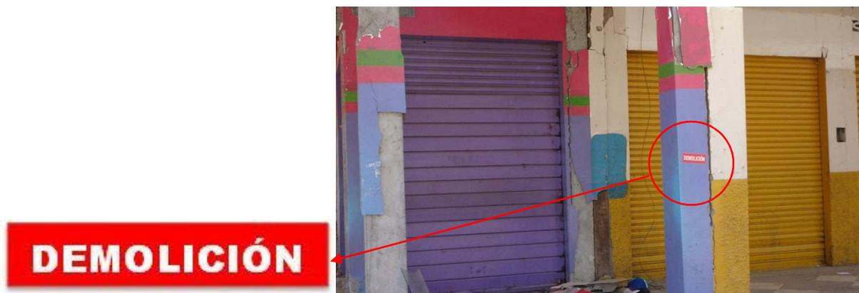
Figure 6-48 Placard for demolition.
