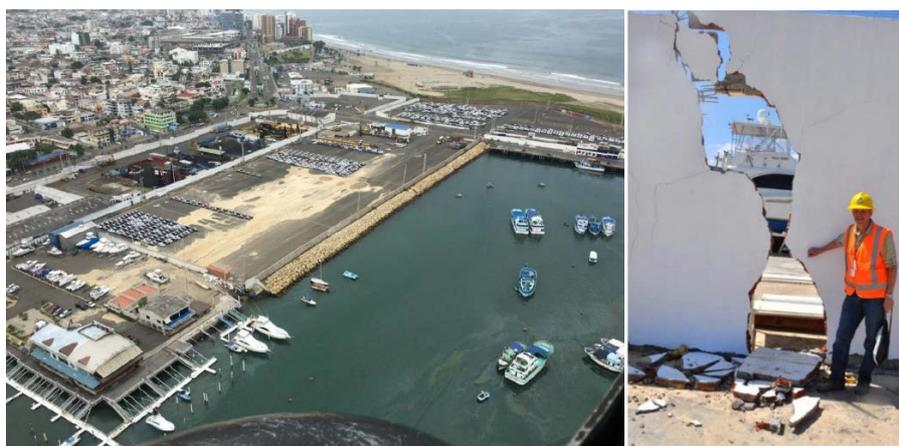
Figure 7-20 Manta Port damage (left: aerial photograph showing extent of liquefaction damage at surface; right: port wall damage, showing for scale K. Rollins, at GPS 0o56'29.6"N, 80o43'27.4"E – from GEER, 2016).
