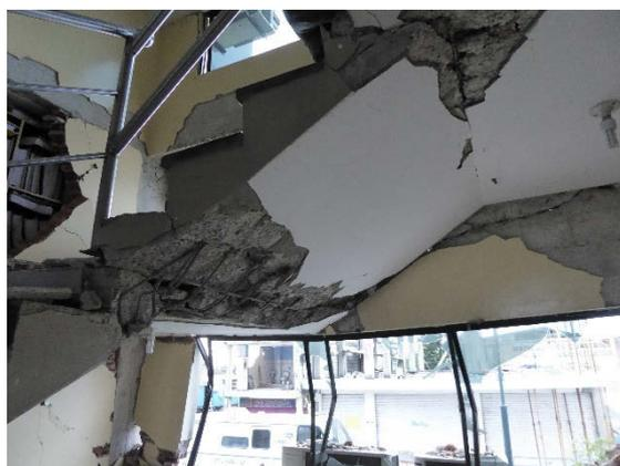
Figure 6-43 Moderate damage to RC staircase.
