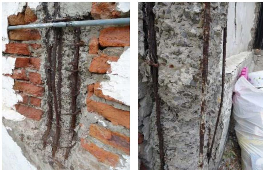
Figure 6-13 Insufficient cover to rebar – note 100% section loss to some of the links.
