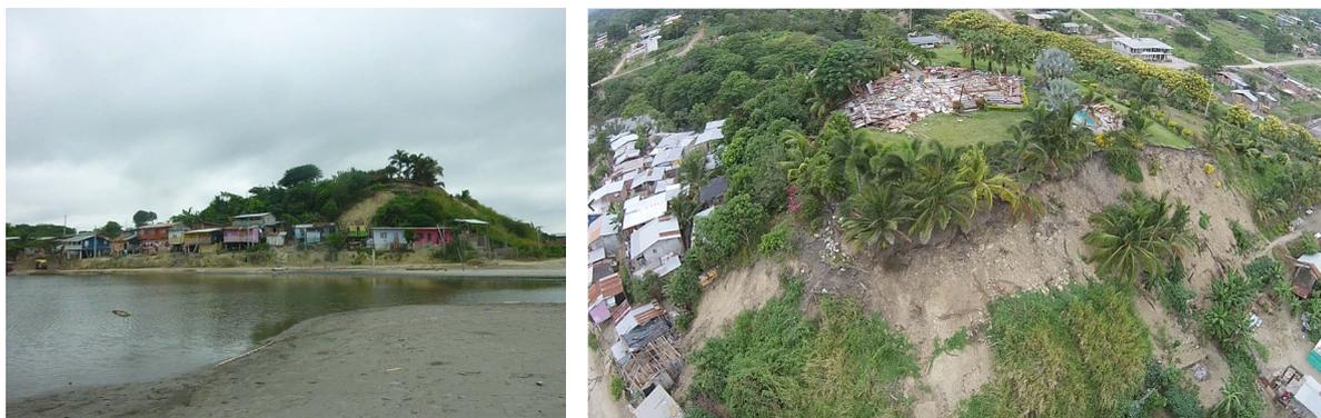
Figure 4-27 Informal settlement damage South of Pedernales due to slope failure (drone image of the head of the slope on the right).
