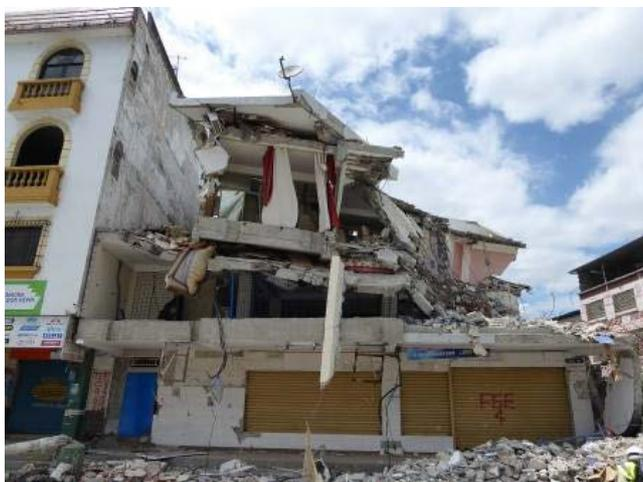
Figure 6-6 Collapsed building, showing failure of façade and frame.
