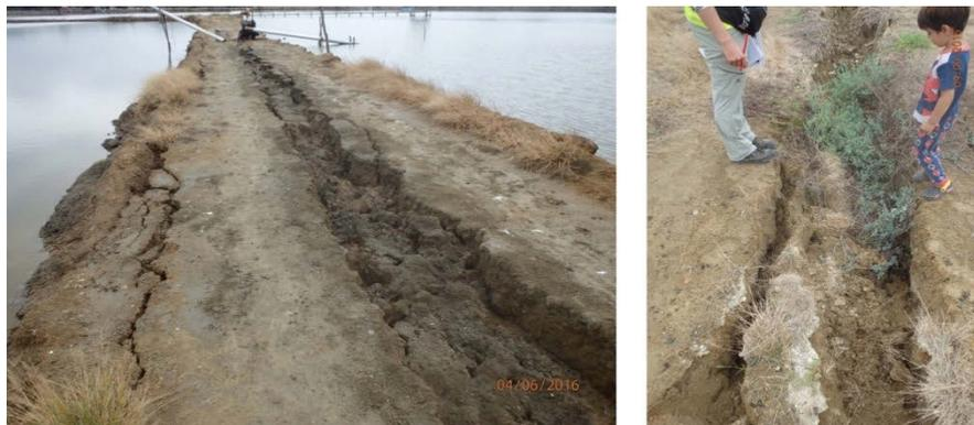
Figure 4-7 Liquefaction induced damage to shrimp farm dykes in Chone River estuary.
