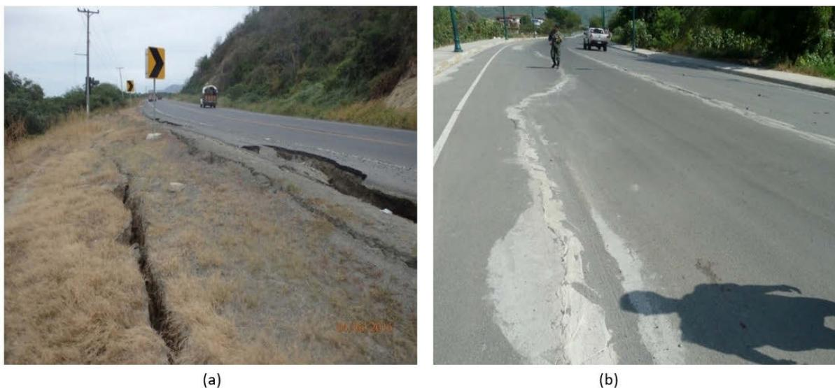
Figure 7-3 Damage to roads due to liquefaction induced lateral spreading (a) Chone river estuary near San Vicente, (b) Portoviejo, close to the Rio Portoviejo.
