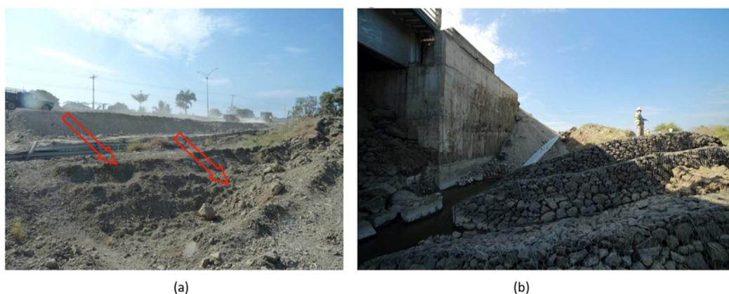
Figure 4-6 Damage to south-west of Mejía Bridge (a) lateral spreading of embankment, (b) sliding and rotation of gabions.
