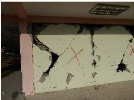
Figure 6-29 In-plane shear cracking of masonry infill walls.
