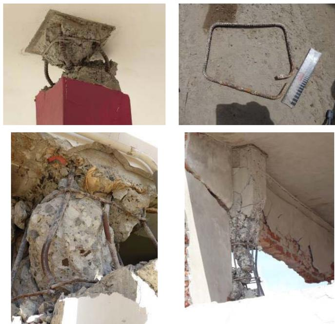
Figure 6-8 Inadequate design and detailing for shear – insufficient link spacing, poor link detailing and plain links used.
