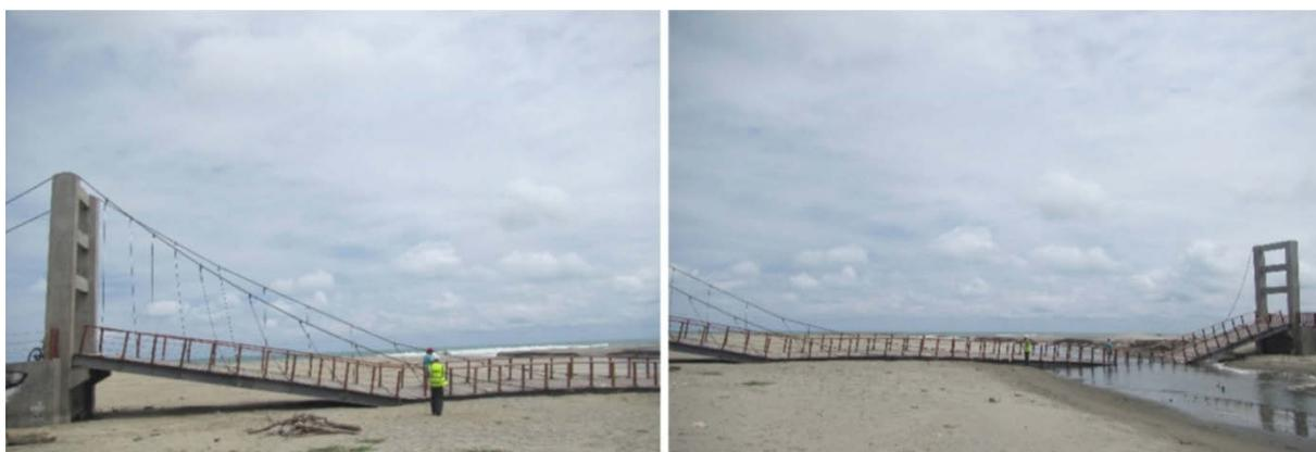
Figure 7-14 Collapsed footbridge in Canoa.
