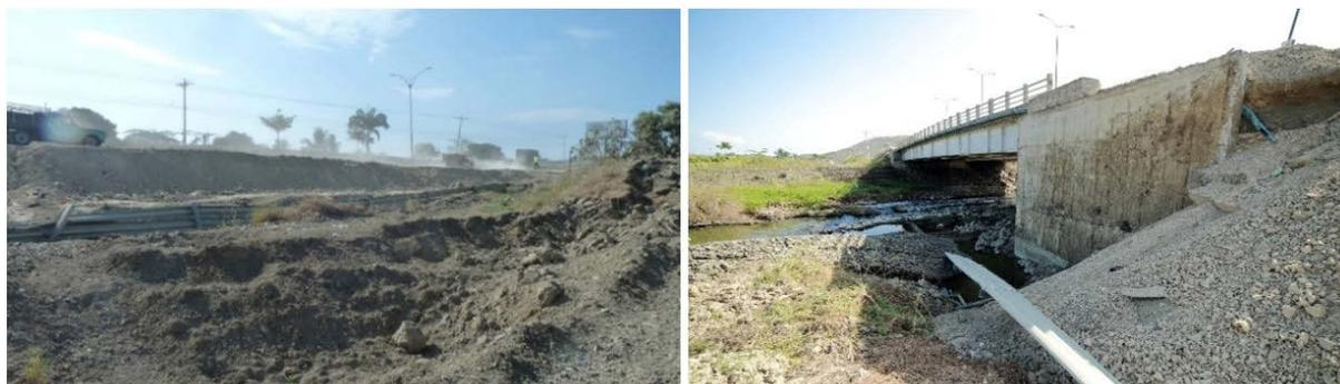
Figure 7-7 Mejía bridge, embankment (left) and gabion wall (right) failure.
