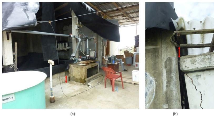
Figure 4-10 Relative uplift of structure with underground storage tanks in Pedernales, showing locations of measured relative settlement.
