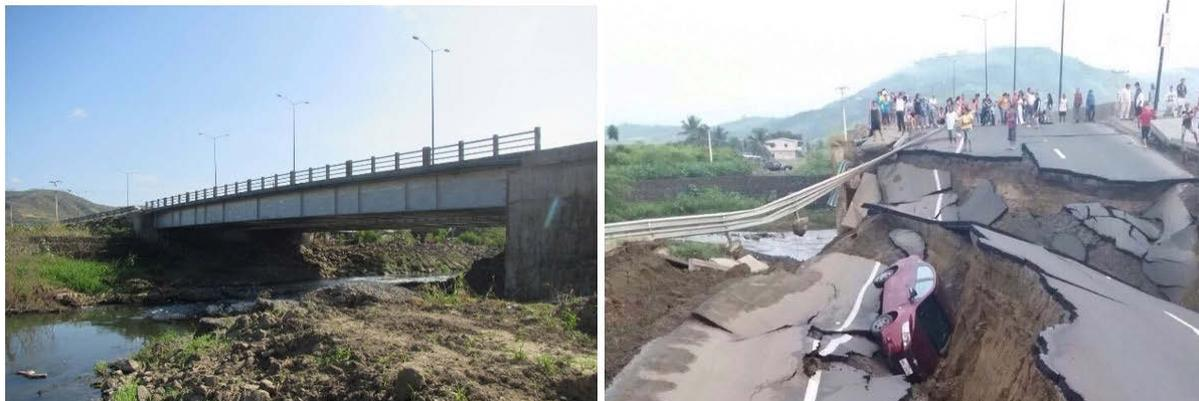
Figure 7-5 Mejía bridge – Highway 39A Portoviejo – Rocafuerte (-0.9899N; -80.4697E). Gabion walls provided on this side of the bridge only. Left – from EEFIT mission; Right - from EERI (2016), posted on twitter just after the main shock (<http://www.eqclearinghouse.org/>).
