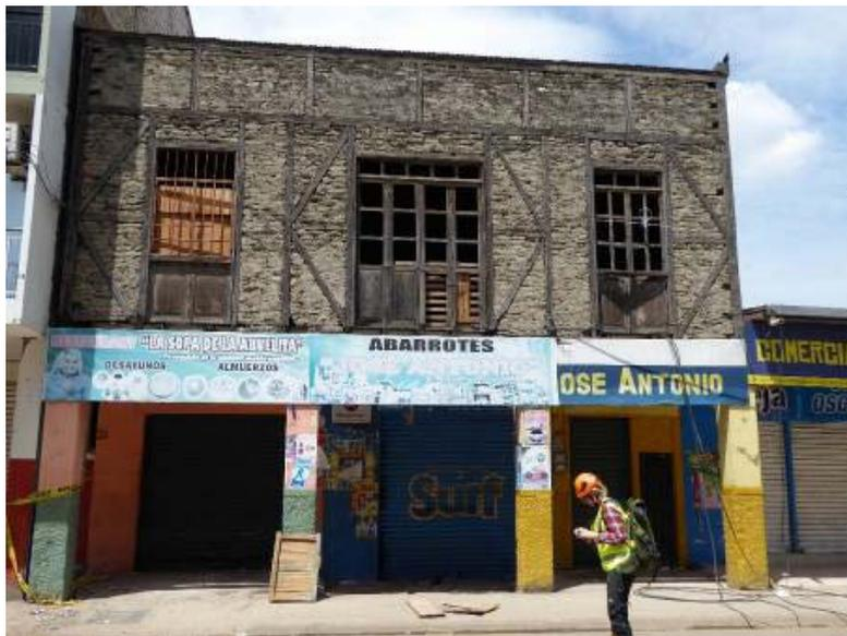
Figure 6-4 Timber frame with masonry infill.
