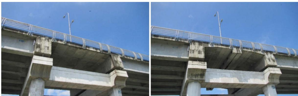
Figure 7-11 Los Caras bridge, continuous connection between main spans (left) and movement joint between main spans (right).
