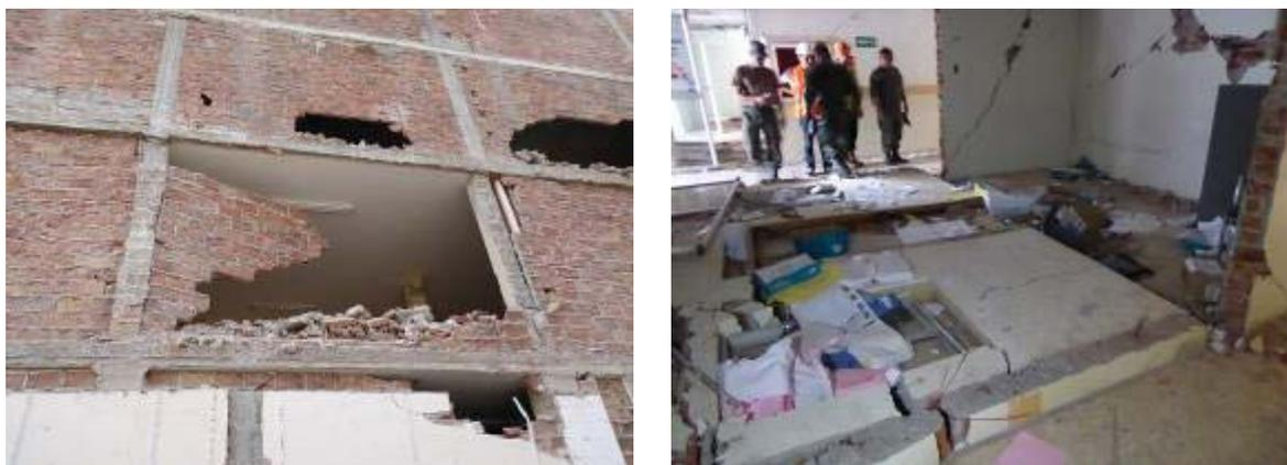
Figure 6-7 Inadequate masonry infill wall design and construction.
