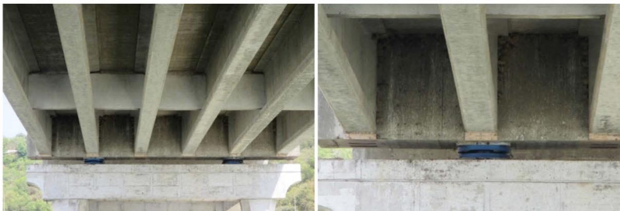
Figure 7-12 Los Caras bridge, location of seismic isolators (left) and close-up view of seismic isolator (right).
