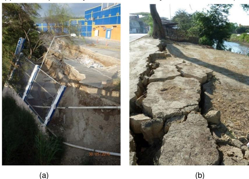
Figure 4-3 Lateral spreading in Portoviejo (a) liquefaction of fill below VelBoni carpark (b) tension cracking due to liquefaction of a lower layer.
