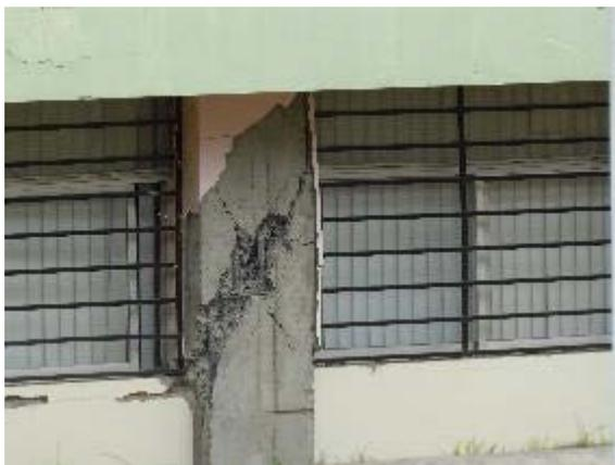
Figure 6-27 Shear cracking due to short column effect.
