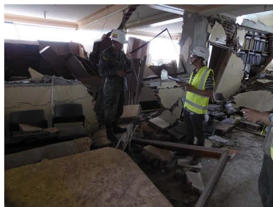
Figure 6-44 Heavy non-structural damage to internal and external masonry wall panels.
