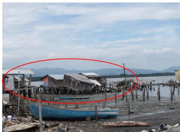
Figure 4-11 Collapse of structures on timber piles in Chamanga.
