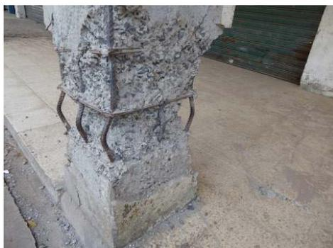
Figure 6-15 Inadequate design of plastic hinges.
