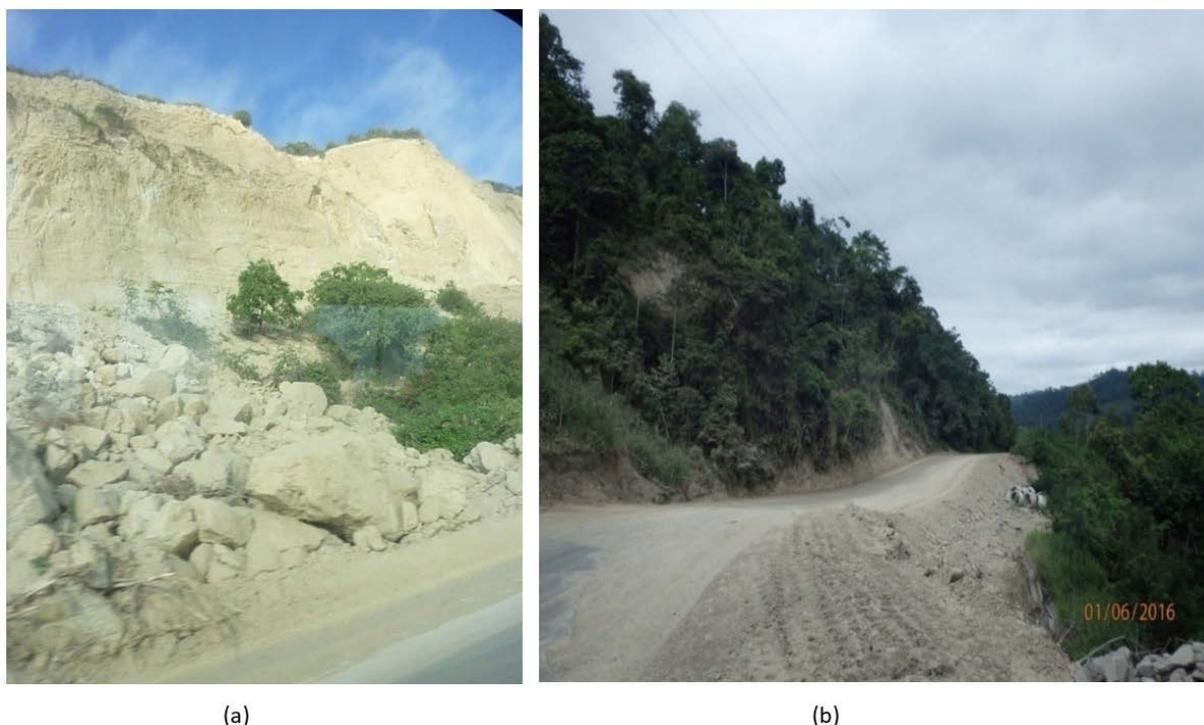
Figure 7-1 Landslide damage to roads (a) on the Highway 15, near Canoa (b) on rural road near San Isidro.
