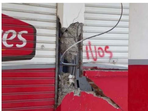
Figure 6-12 Short columns at a shop front – note the local crushing of the masonry lining up with an imaginary compression strut and local shear failure of the column.
