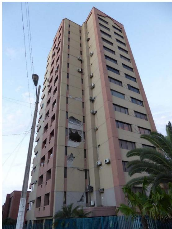
Figure 6-2 Reinforced concrete frame with masonry infill walls – engineered high-rise.
