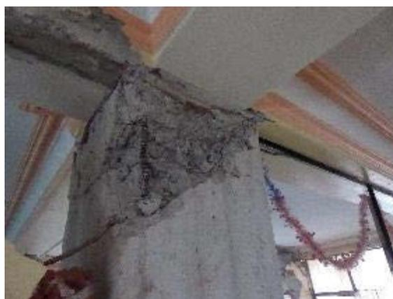
Figure 6-42 Local damage to head of RC column.
