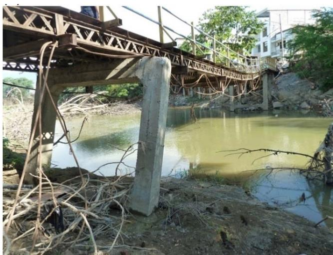
Figure 7-17 Structural damage due to lateral spreading along Rio Portoviejo observed on the rotation and lateral displacement of foundations of the Puente Chile in Pedernales.
