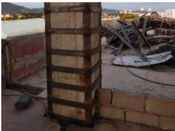
Figure 6-33 Steel plate retrofit to reinforced concrete column.
