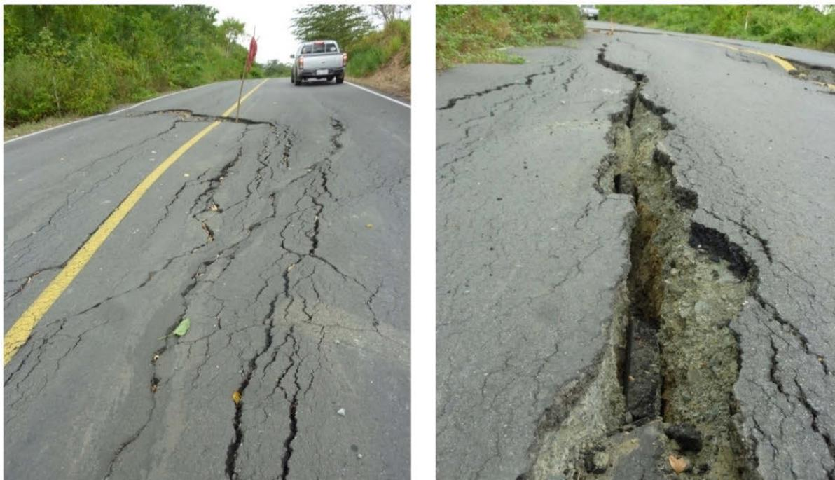
Figure 7-2 Examples of cracking on roads near San Isidro.
