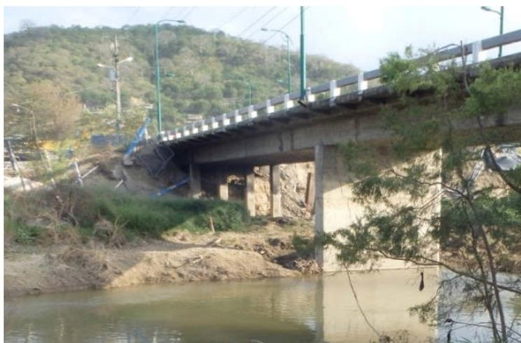
Figure 7-18 Movement of soil from around the Velasco Ibarra bridge foundations.
