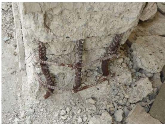
Figure 6-17 Poor quality concrete.
