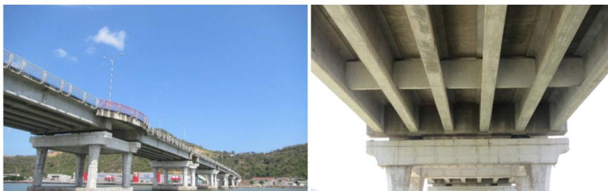
Figure 7-10 Los Caras bridge, 45m-long decks supported by 4-column piers (left) and deck's prestressed concrete beams showing also seismic isolators (right).
