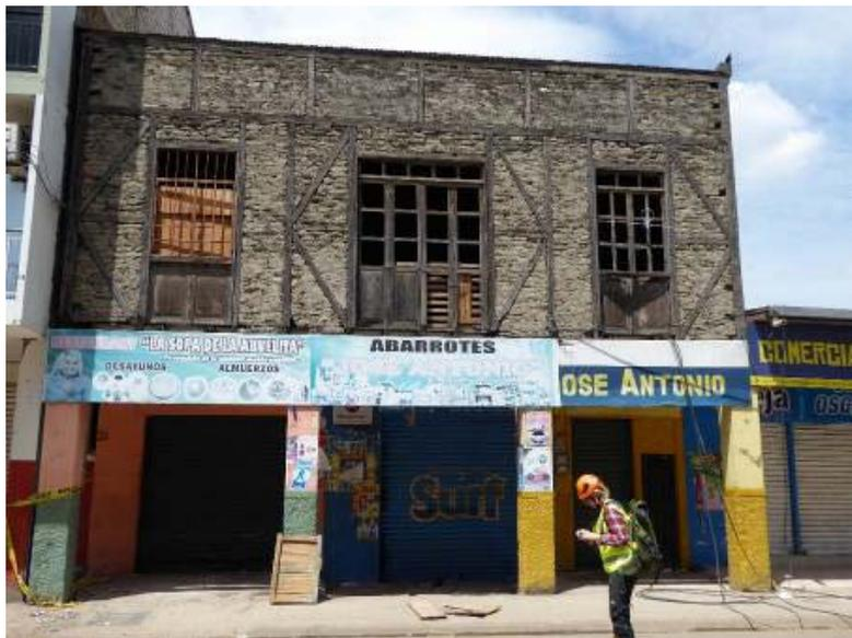
Figure 6-4 Timber frame with masonry infill.
