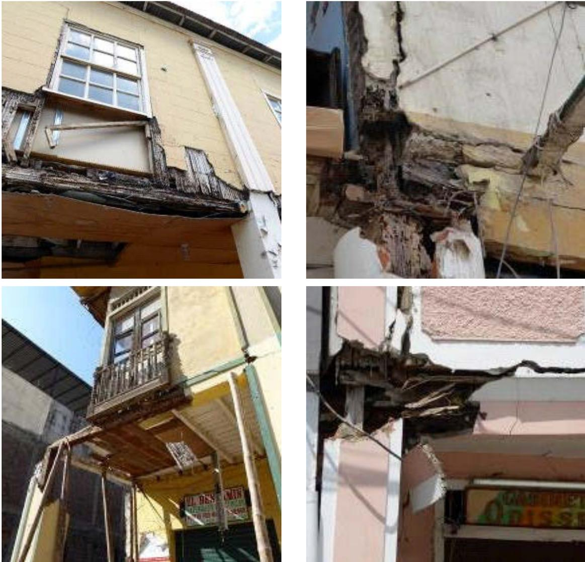
Figure 6-18 Examples of rot and insect damage.
