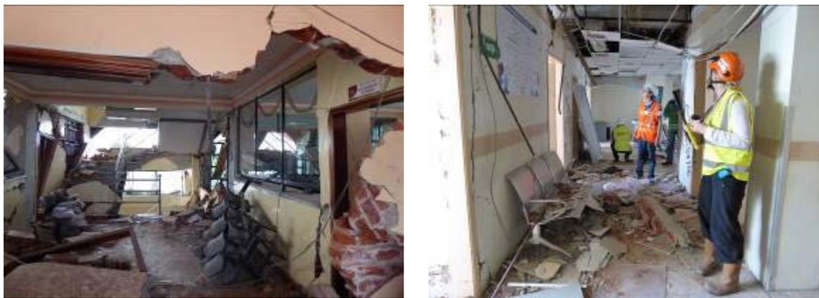
Figure 6-16 Inadequate securing of non-structural elements – the image on the right depicts a hospital corridor.
