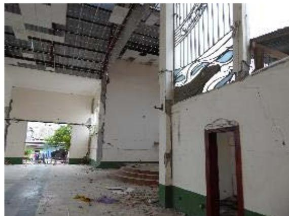
Figure 6-40 Internal damage to ceiling tiles and masonry walls.
