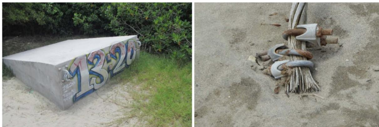
Figure 7-15 Footbridge in Canoa, right end anchorage block (left) and suspension cable end that failed at anchorage (right).
