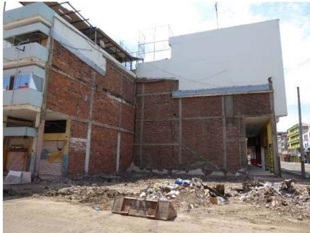
Figure 6-1 Reinforced concrete frame with masonry infill walls – non-engineered low-rise.
