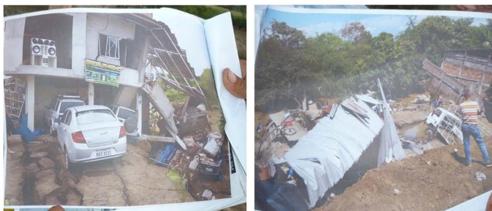
Figure 4-5 Collapse of structures along Rio Portoviejo due to liquefaction induced lateral spreading.
