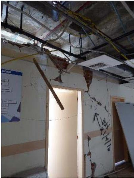
Figure 6-37 Significant damage to false ceiling and fittings.
