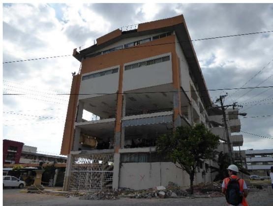
Figure 6-28 Complete out-of-plane failure of masonry perimeter infill walls.
