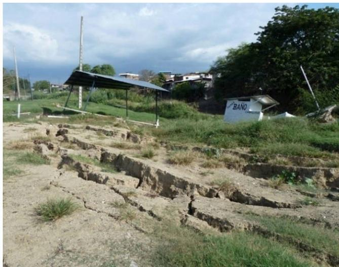
Figure 4-4 Structural damage due to lateral spreading along Rio Portoviejo consisting in the rotation and settlement of structures at sports pitch.
