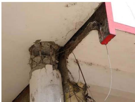
Figure 6-14 Pounding of a column head by a slab of an adjacent building.
