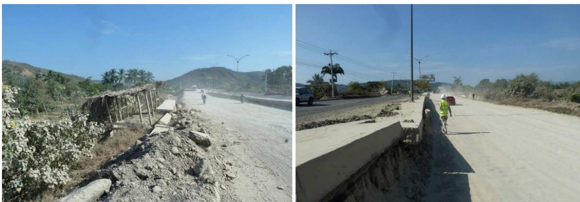
Figure 7-6 Mejía bridge, differential settlement between the two separate sections as seen from the bridge's approach.
