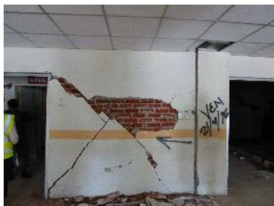
Figure 6-36 In-plane shear cracks.
