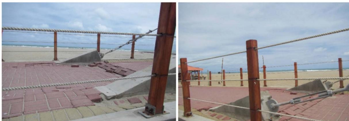
Figure 7-16 Footbridge in Canoa, left end anchor points experienced uplift.
