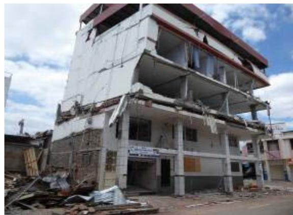
Figure 6-10 Exposed reinforcement with possible inadequate lap lengths for future construction, and an upper storey soft/weak storey failure.
