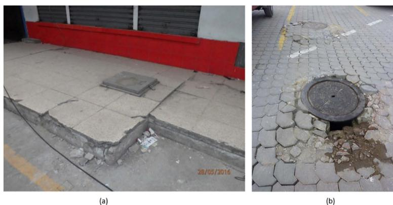
Figure 4-9 Protrusion of manholes in Manta (a) and Pedernales (b).
