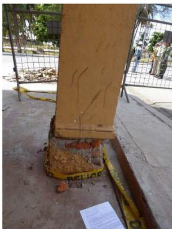
Figure 6-19 Lack of positive connection between frame and masonry upstand, leading to sliding of column laterally.
