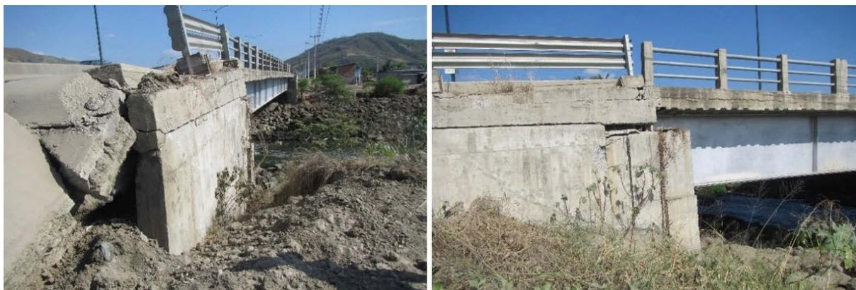
Figure 7-8 Mejía bridge, damage in abutment.
