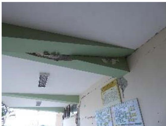
Figure 6-30 Pounding at movement joint.
