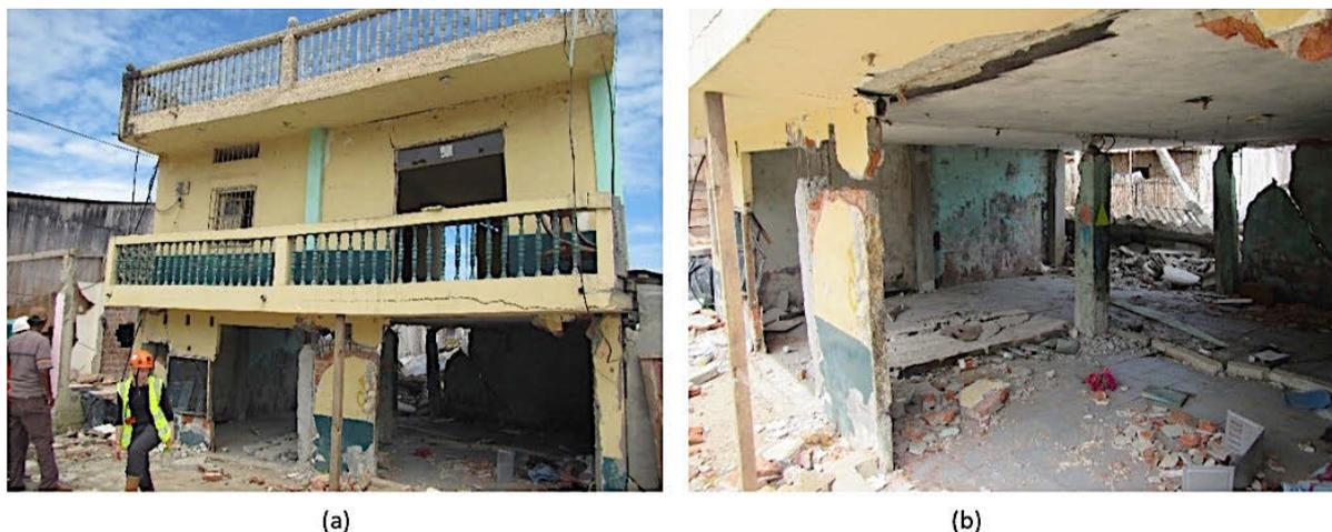
Figure 4-13 Damage due to differential settlement of building in Chamanga (a) concrete cracking due to differential settlement, (b) detail of structural damage to building.
