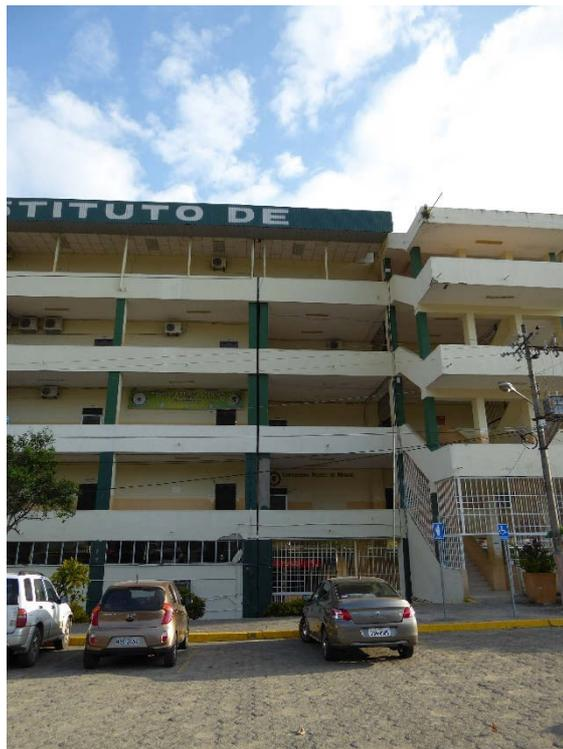
Figure 6-32 Permanent lateral drift of buildings relative to one another of approximately 50mm (follow movement joint below “DE”).
