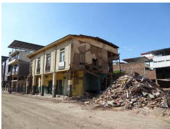
Figure 6-20 Possible damage due to debris from adjacent buildings.
