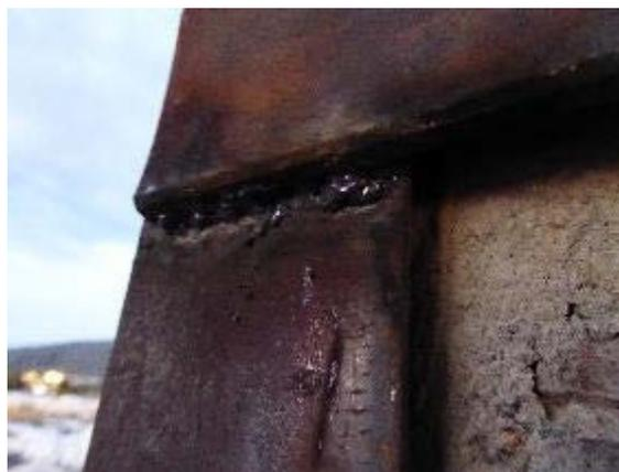
Figure 6-34 Site welded steel plate.
