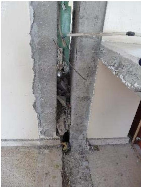
Figure 6-31 Movement joint filled with rubble (prior to event).
