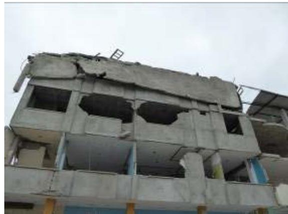
Figure 6-9 Weak and soft storey failures.
