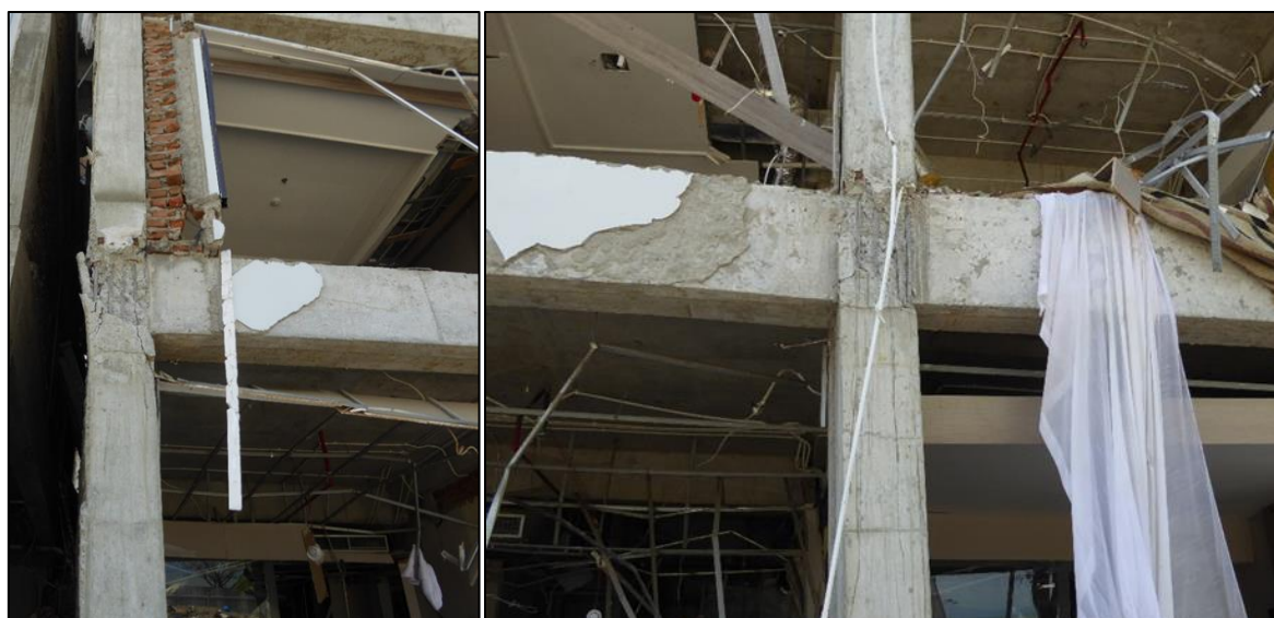
Figure 7.46 – Mercure Hotel – Images of cover spalling in RC frame joints in the second storey of the structure
