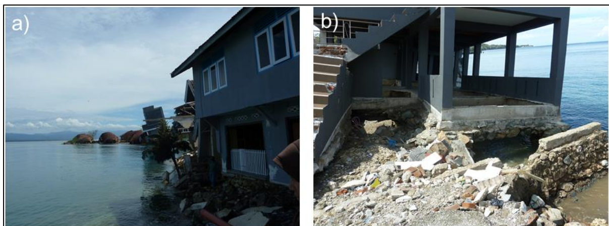
Figure 5.23.- Photographs of Donggala Port, looking a) South East across the estuary towards the partially collapsed metal rooved storage houses b) detail beneath the concrete structure seen tilted on the South edge of the bay, showing evidence of soil having been displaced from beneath the structure.
