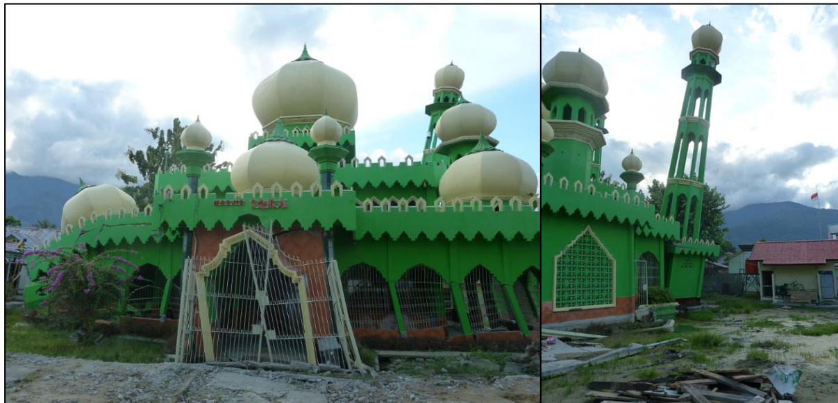
Figure 5.6 – Left: Front of Masjid Iqra. Right: Masjid Iqra in Lasoso. Severe liquefaction-induced damage and tilting of minaret due to liquefaction beneath base.
