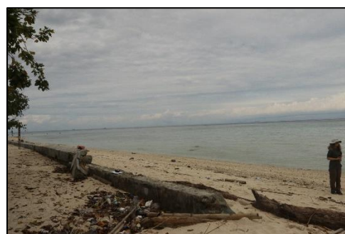
Figure 7.54 - Rudimentary seawall. Left - Sketch of layout and section. Right - Damaged sections with tree trunks closing the gap.
