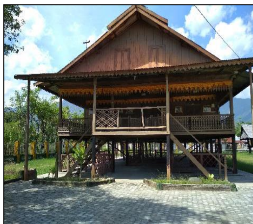
Figure 7.4 - Performance of timber stilt houses in Palu and Dongqala, Central Sulawesi: Left – The palace of the Princes of Palu. This structure was affected by ground shaking but not tsunami inundation and was undamaged. Right - The remaining concrete foundations of the timber stilt houses in the Labuan Bajo Fisherman Village, shown in red circle. Collapsed stilt houses can be seen in the background.
