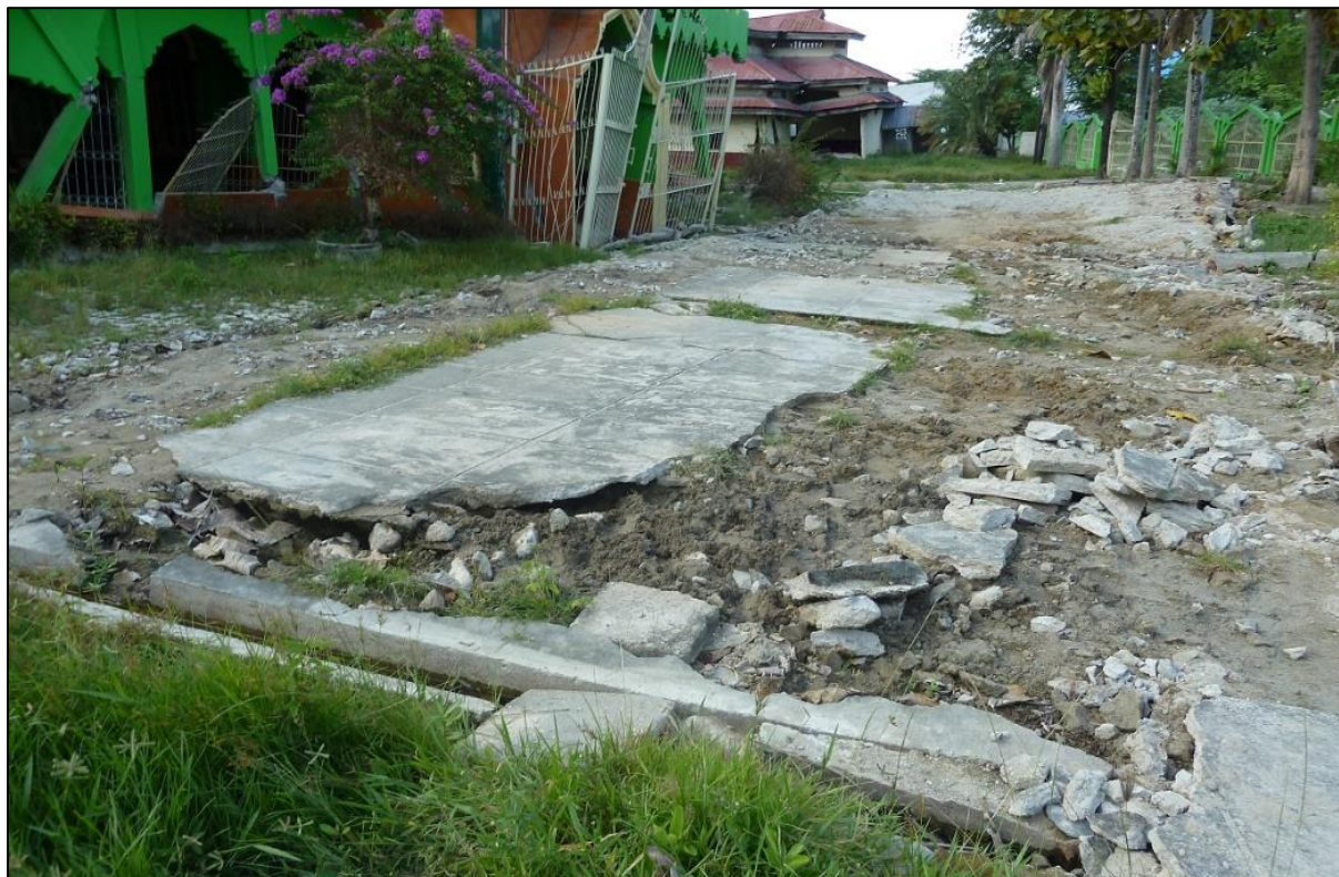
Figure 5.7 -. Masjid Iqra. Failure of garden paving above sandy soil, and ejecta in background.
