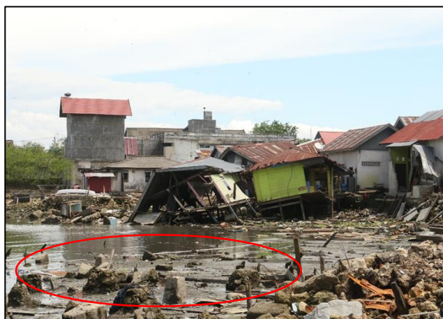
Figure 7.4 - Performance of timber stilt houses in Palu and Dongqala, Central Sulawesi: Left – The palace of the Princes of Palu. This structure was affected by ground shaking but not tsunami inundation and was undamaged. Right - The remaining concrete foundations of the timber stilt houses in the Labuan Bajo Fisherman Village, shown in red circle. Collapsed stilt houses can be seen in the background.
