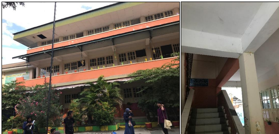
Figure 7.32 - MTS Alkhairaat Pusa Palu School. Left – 3-storey RC frame building that sustained minor damage to infill panels. Right – Typical sizes of beams and columns in RC frame schools.
