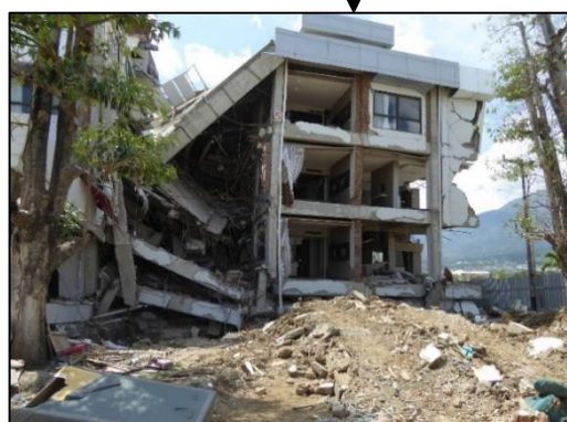
Figure 7.45 – Mercure Hotel, which suffered soft-storey failure of ground floor. Top – Image of the hotel before the earthquake, Source: Tripadvisor.com. Bottom – Pictures of the Hotel after the earthquake, showing the soft-storey failure of the ground storey of the structure.
