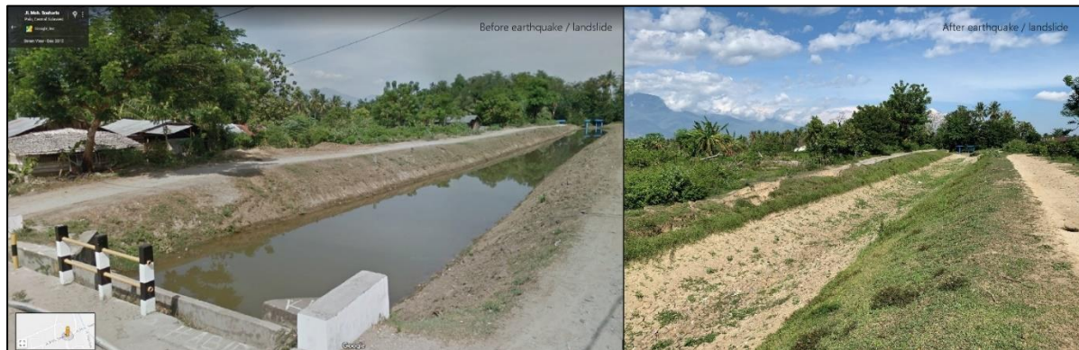
Figure 4.10 – Far northern end of the Bendung Iriqasi Gumbasa irrigation channel above the head of the Petobo Landslide before (left) and after (right) the earthquake.
