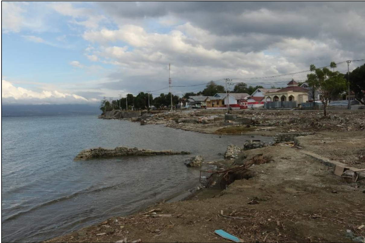
Figure 6.16 - Damage in Labuhan Bajo.
