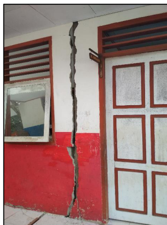
Figure 7.8 - Typical earthquake damage observed in infilled timber frame construction. Left - Out-of-plane failure of infill panels. Right - Separation of infill from frame due to differential settlement of foundations.
