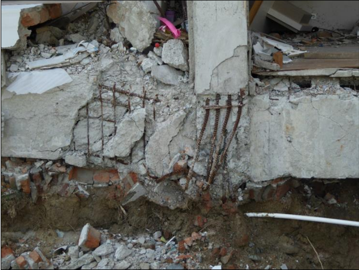
Figure 7.47 – Mercure Hotel – Detail of a joint within the first floor of the building (now at ground level following soft-storey collapse of ground floor).
