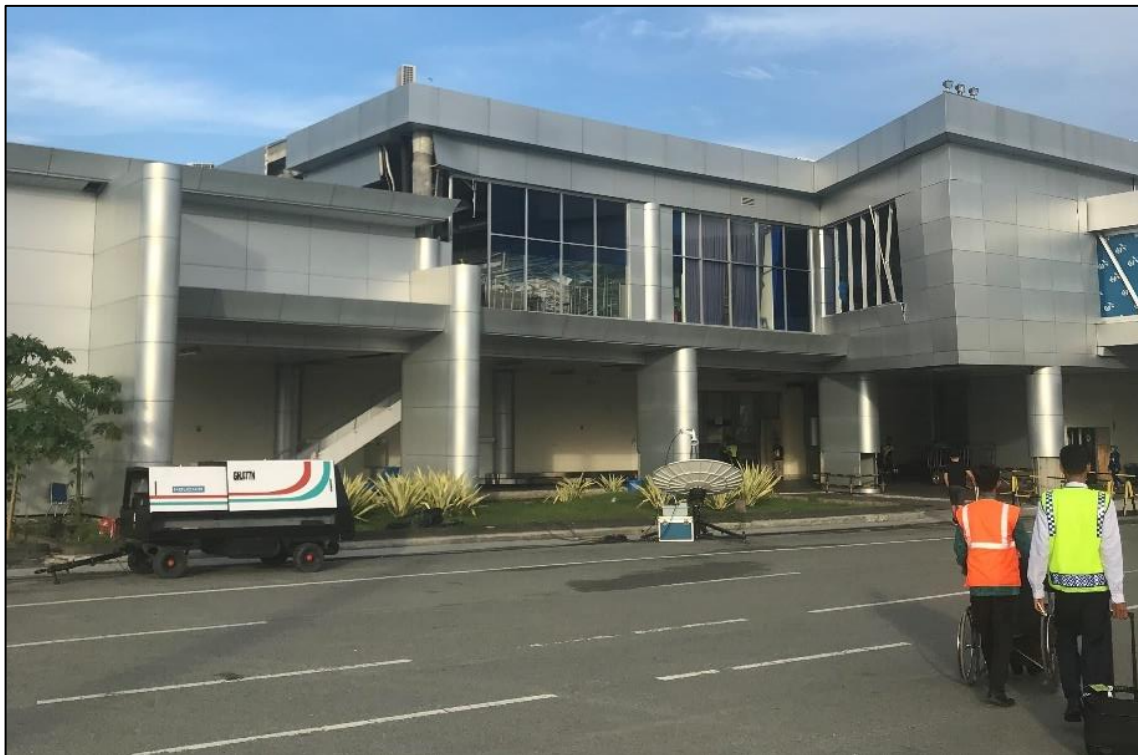
Figure 7.50 - View of Palu Airport passenger building from the runway. Damage to the infill walls at the ground floor is observed. A stack of fallen ceiling cladding can be seen in upper storey window.
