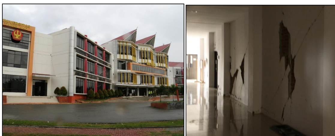
Figure 7.19 - Tadulako University Rektorat (DET2): exterior view (left); damage to internal infill panels (right)
