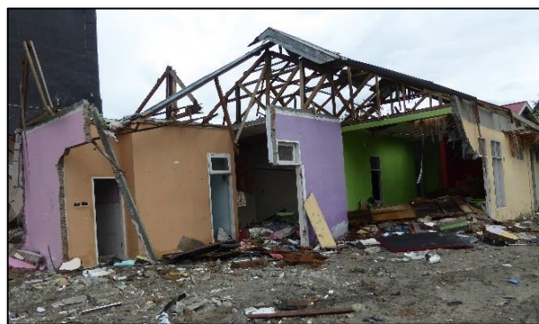
Figure 7.10 – Heavily damaged CM houses in Palu bay area along the Jl. Rajamoili road, about 100m from coastline. The walls of this house were directly hit by the tsunami inundation.
