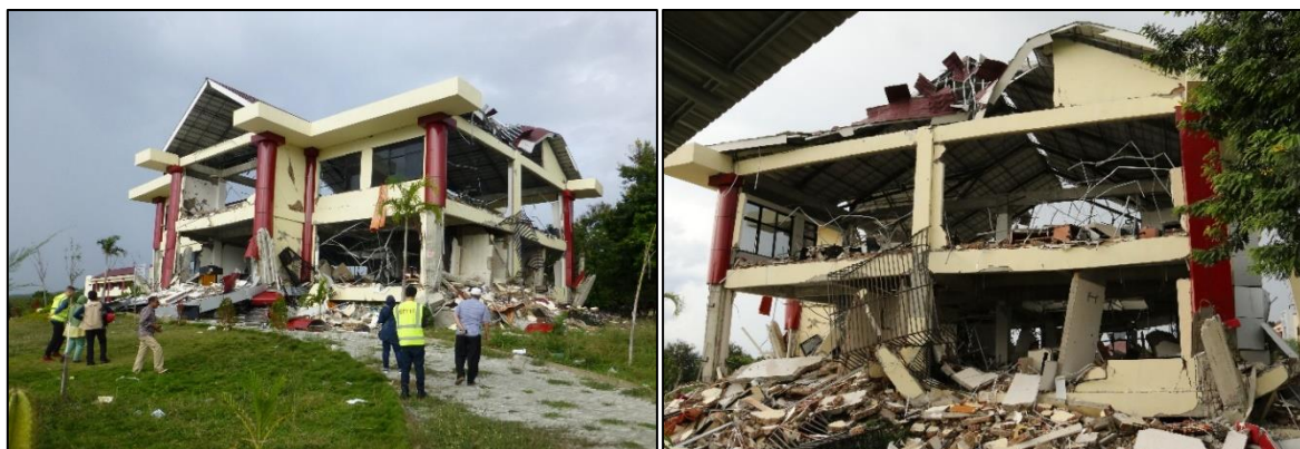
Figure 7.20 - Tadulako Univerity collapsed 3-storey building of the Faculty of Social and Political Sciences. Left – front view. Right – back view.
