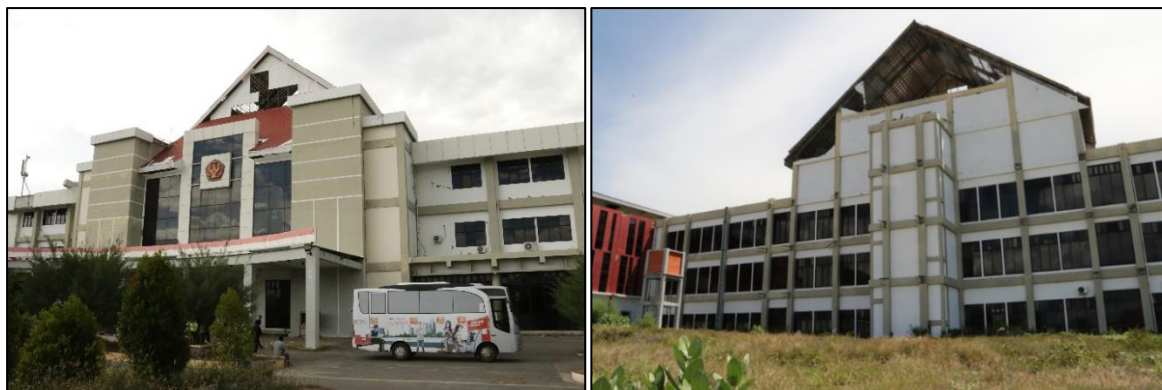
Figure 7.36 - Tadulako University Hospital Building A. Left – Front view. Right – rear view, showing damage to gable.
