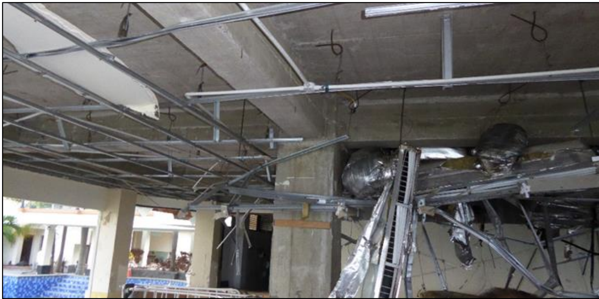
Figure 7.49 - Swiss Belhotel - damage to internal fittings at the ground storey of the shoreward side of the hotel. No structural damage observed in the main RC structure.
