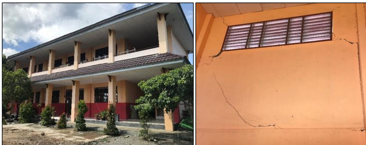
Figure 7.33 - SD Negeri Pengawu School in Palu (Building A in Fig. 7.24c). Left – 2-storey RC school building that sustained moderate damage to infill panels. Right – Damage to the infill walls
