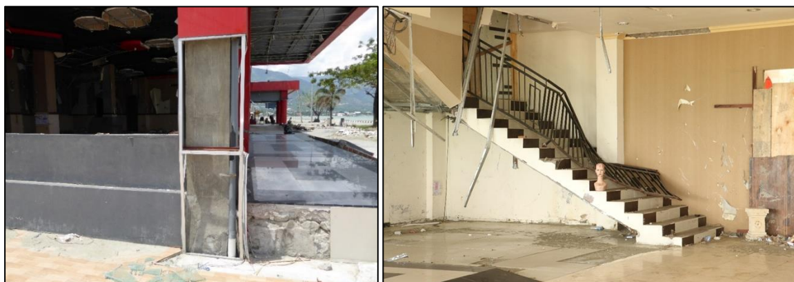
Figure 7.43 – Grand Duta Hotel, Left – image of intact column at ground floor. Right – Image of staircase inside the ground floor of the hotel. The staircase railing was damaged when it was hit by a large desk moved by the tsunami inundation.
