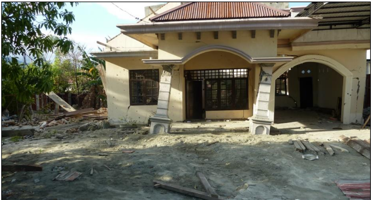
Figure 5.5. - Damage to a one-storey building in Lasoso due to differential settlement induced by liquefaction. Sandy ejecta in garden.
