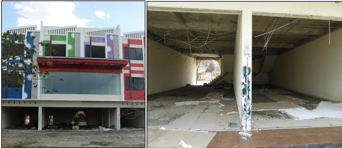
Figure 7.44 – Three –storey RC building near the Grand Duta Hotel. This structure was inundated by the tsunami at its ground floor, but sustained no structural damage, just non-structural damage to sea front windows and to back walls and to fittings at ground-floor level.
