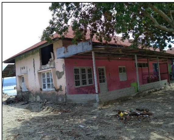
Figure 7.6 - Examples of infilled timber frame construction in Labuan Bajo. Left - Timber framed house with wire-reinforced mortar. Right - Two storey timber framed house with mortar infill.
