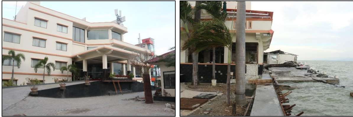
Figure 7.48 - Swiss Belhotel (Left) Undamaged front facade facing away from the bay (Right) Loss of confined masonry one-storey buildings to the shoreward side of the hotel
