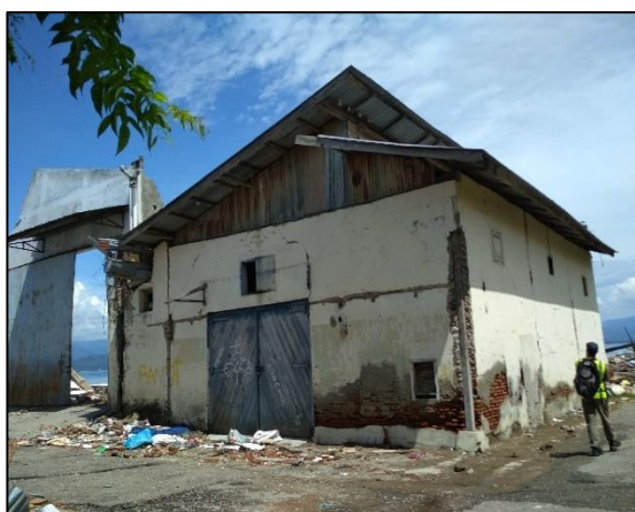
Figure 7.7 - Examples of infilled timber frame construction. Left - Timber framed warehouse with masonry infill in Labuan Bajo (left). Right - Elementary school at Wani, timber frame construction with mortar infill.
