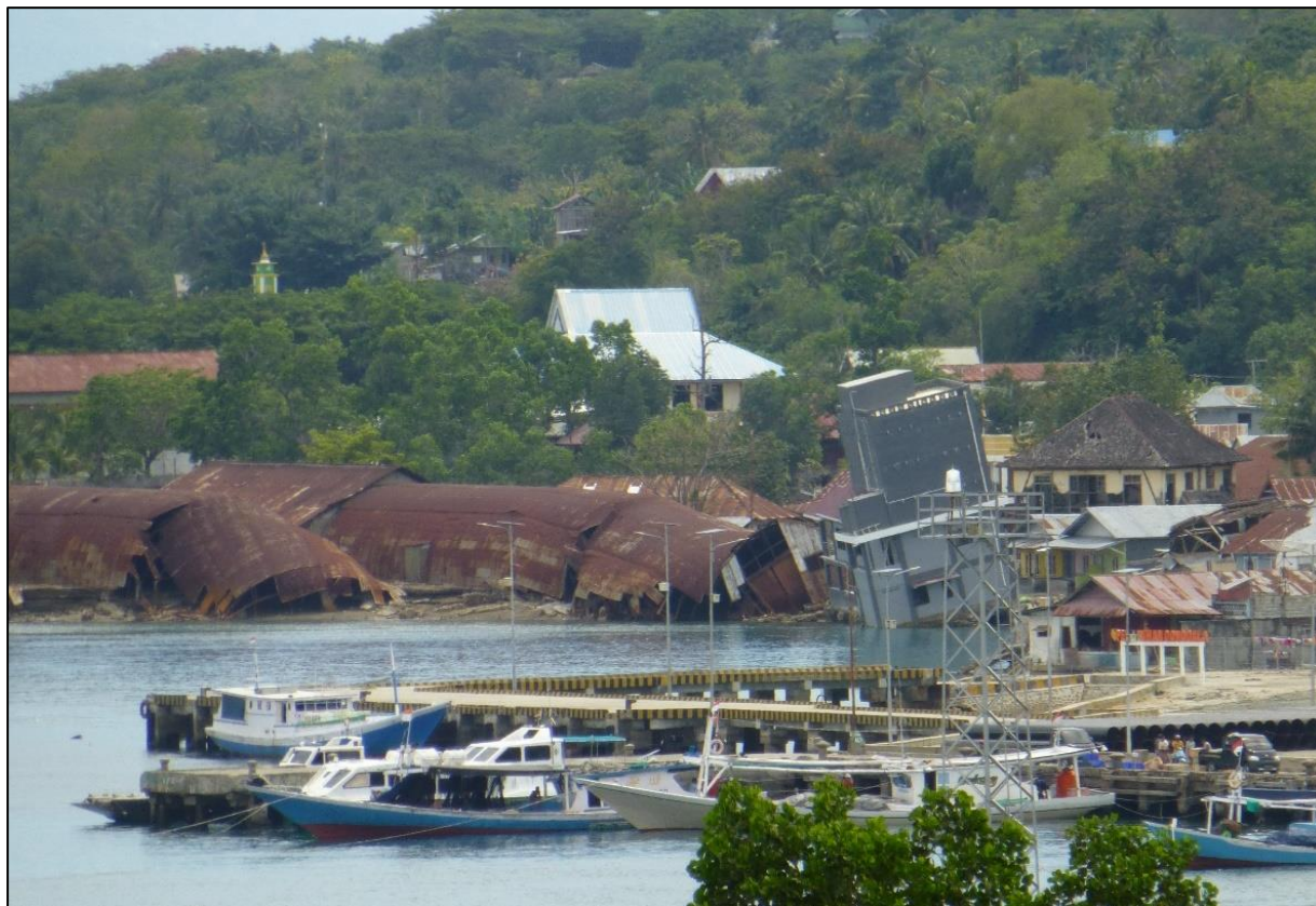
Figure 7.59 - Damage to old port of Donggala
