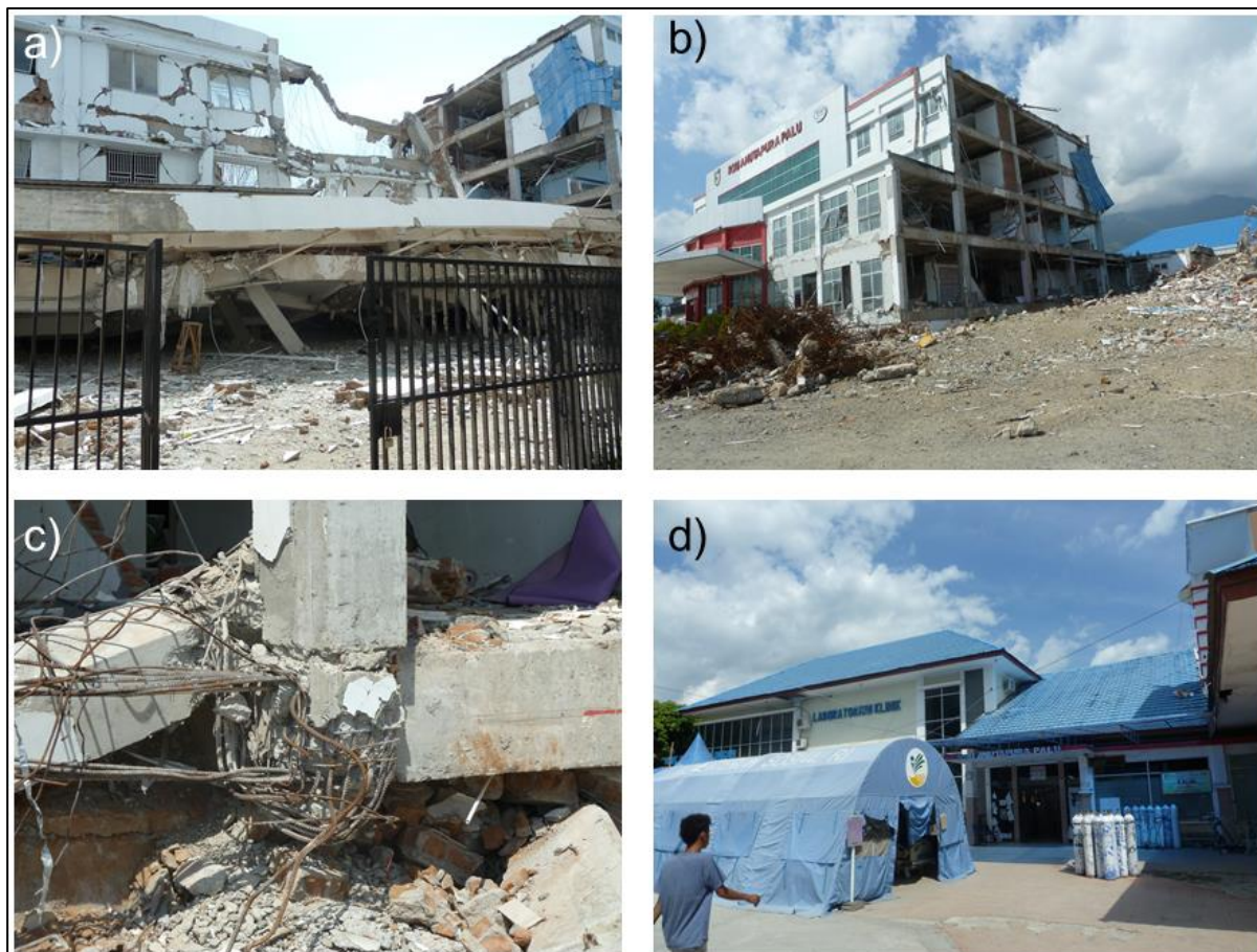
Figure 7.40 - Damage at Anutapura Hospital a) soft story collapse of four story RC frame structure; b) RC frame of remaining structure visible following removal of collapsed debris; c) column=beam joint reinforcement exposed in collapsed structure; d) low-rise hospital structures were relatively undamaged and remained operational.
