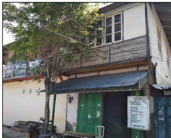
Figure 7.6 - Examples of infilled timber frame construction in Labuan Bajo. Left - Timber framed house with wire-reinforced mortar. Right - Two storey timber framed house with mortar infill.
