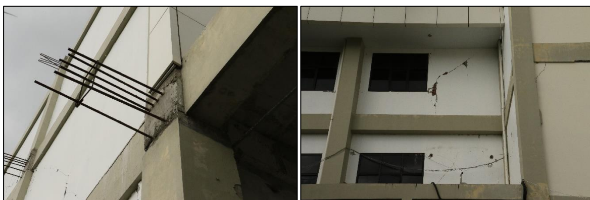
Figure 7.37 - Tadulako University Hospital Building A. Left – Beam reinforcement detailing. Right – damage to brick masonry infills.
