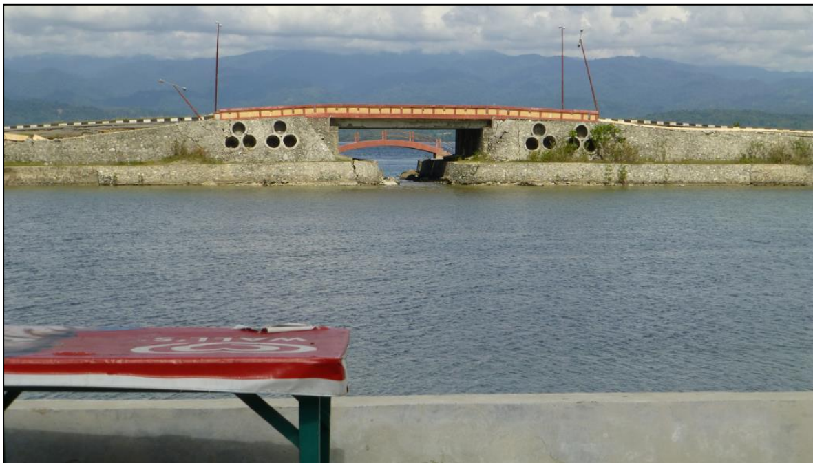
Figure 5.16 - View across dolphin enclosure to sea road. Slight damage to bridge abutments consistent with soil displacements, though bridge remains operational.
