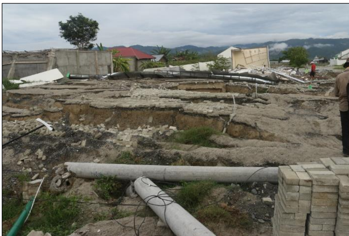
Figure 5.12 - Differential settlement and ground disturbance in Sigi. Pipework in foreground appears to be new rather than uplifted.
