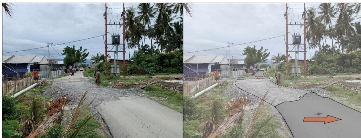
Figure 3.4 – Offset road due to strike-slip fault displacement.
