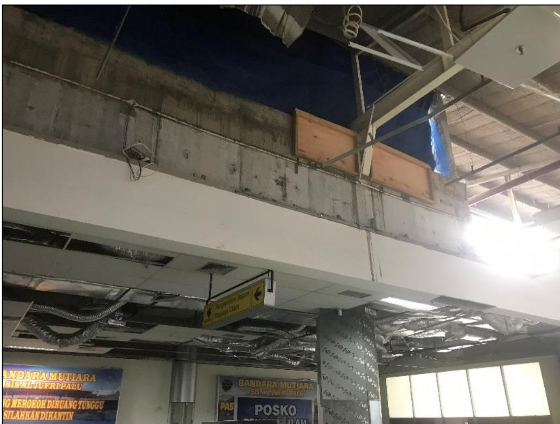
Figure 7.51 - Picture of missing ceiling cladding and damaged fixtures, inside Palu Airport passenger building.
