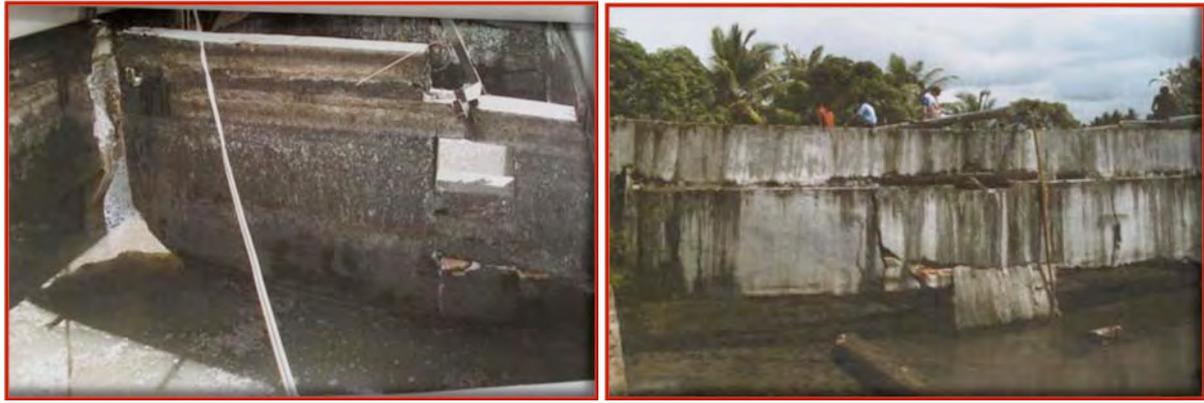
Figure 41. Damage to the reservoir where poisonous materials are removed before disposal of residual waters (photos provided by the plant manager).
