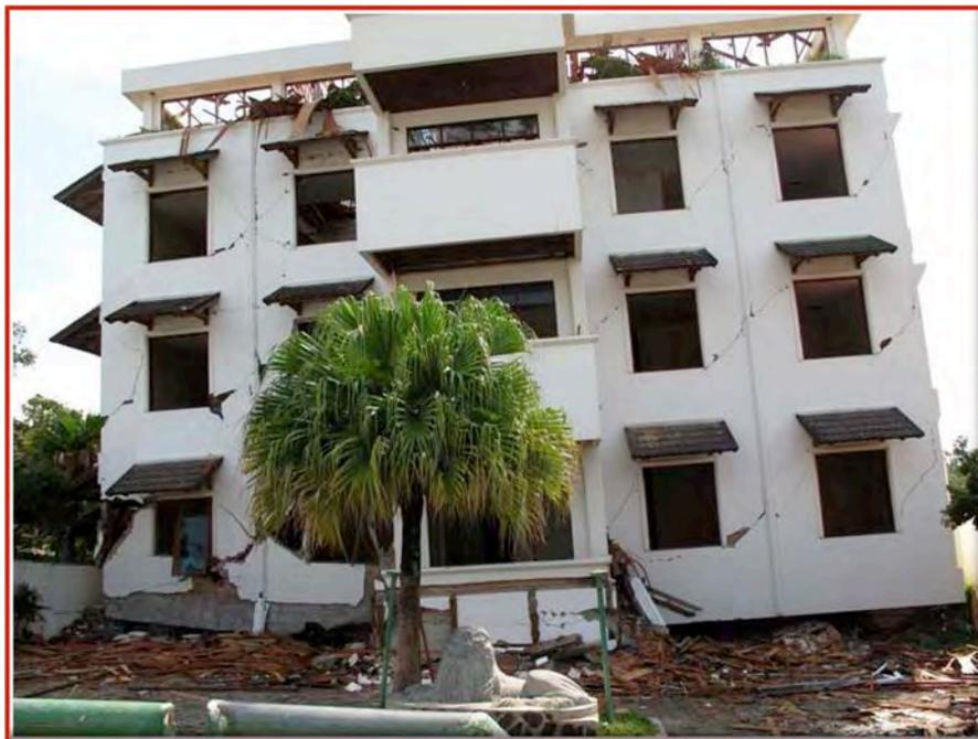
Figure 26. Examples of Soft-storey Hotel Failures.
