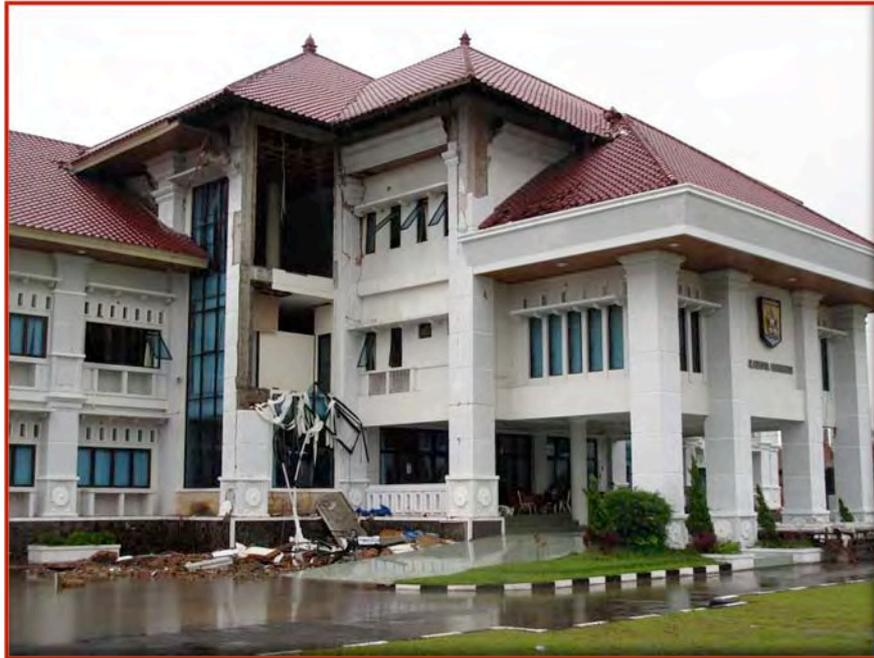
Figure 37. Governmental building in Pariaman city. In spite of the irregular geometry of the building, the observed damage was limited to the two infill walls.
