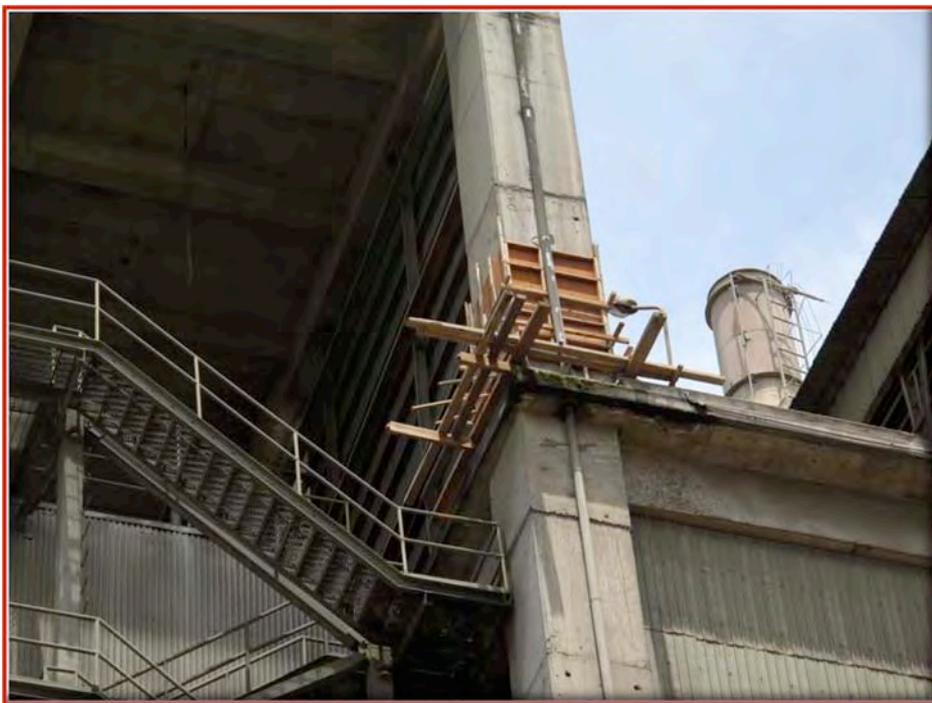
Figure 39. A minor problem with a RC column in the cement factory where part of the face concrete was damaged and then repaired. This did not represent a structural problem.
