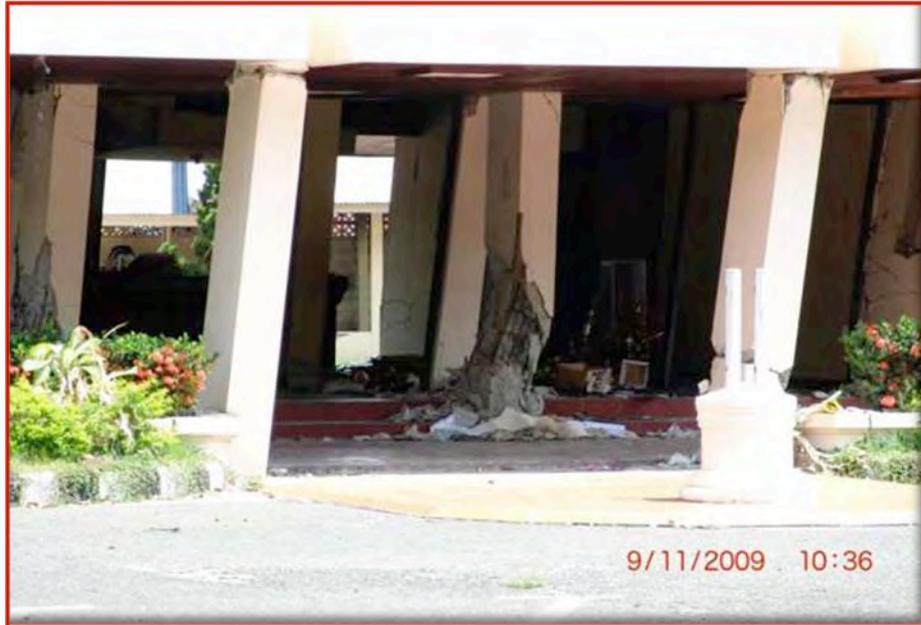
Figure 35. Soft storey failure of a governmental building in Padang, with the bottom photograph showing the failure of the column in the area indicated in the upper photograph.
