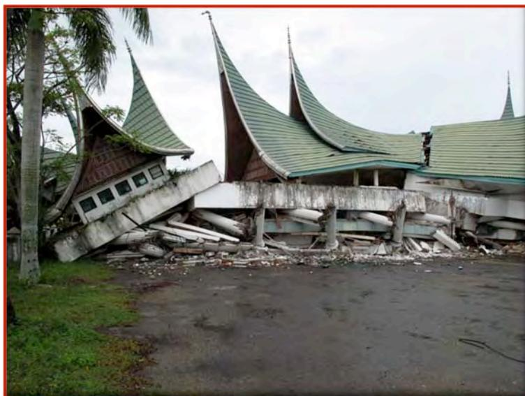
Figure 36. Examples of soft storey failures in governmental buildings in Padang.
