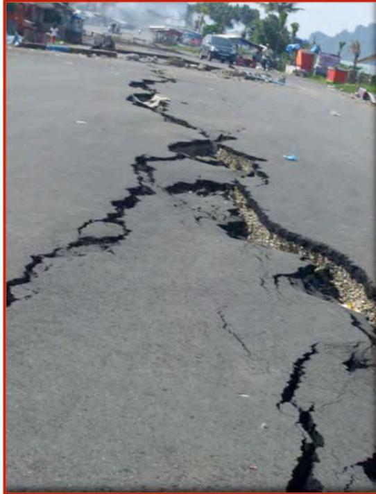
Figure 55. Tension cracks propagating parallel to the longitudinal axis of the road.
