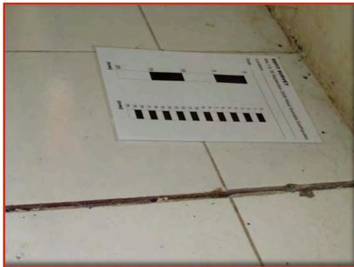
Figure 58. Crack on floor tiles of classroom due to differential settlement.
