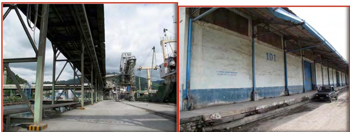
Figure 42. No structural damage was observed in any of the port facilities. Left: light steel structure. Right: warehouse of RC moment resistant frames with infill walls.
