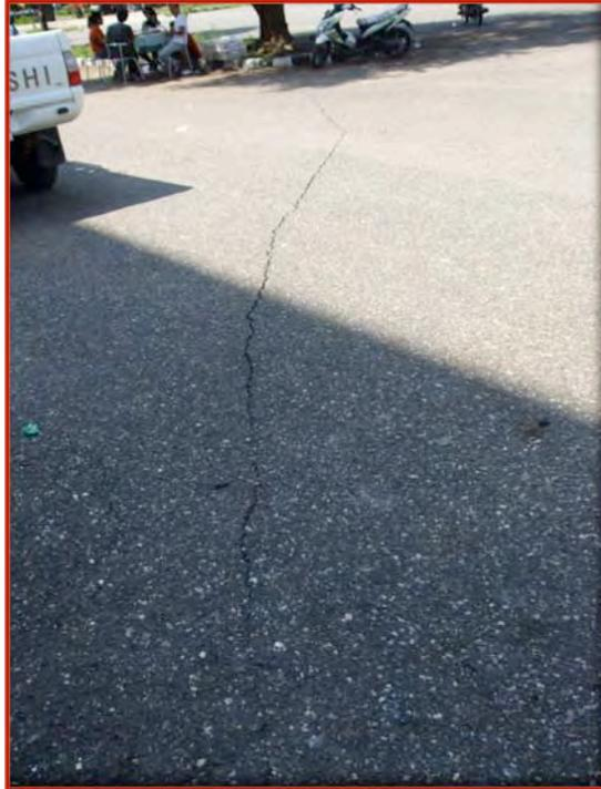
Figure 57. Road cracks parallel to the plane of fault rupture.
