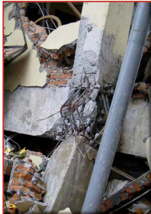
Figure 28. Evidence of soft-storey failure, light-fixture and chair at ground level (left) and lack of transverse reinforcement in beam-column connection (right).
