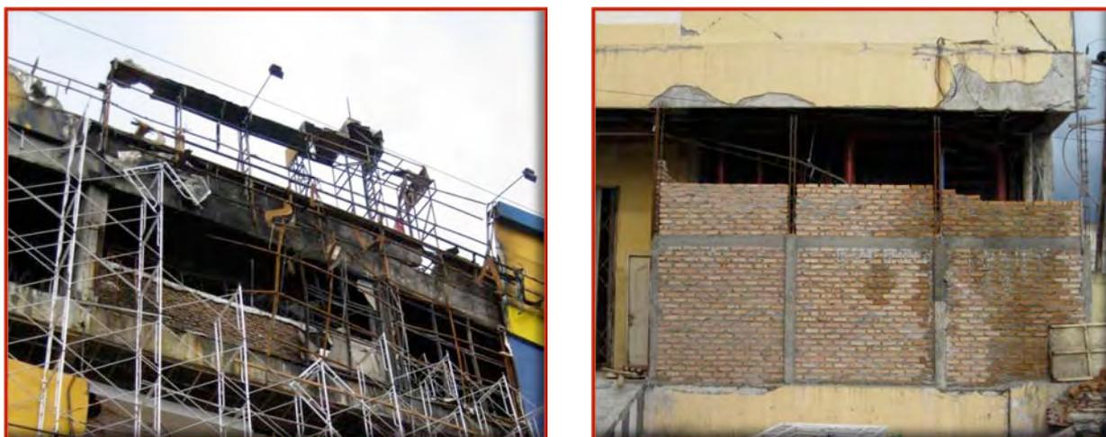
Figure 34. Ramayana Shopping Centre: fire damage (left) and new masonry construction (right).
