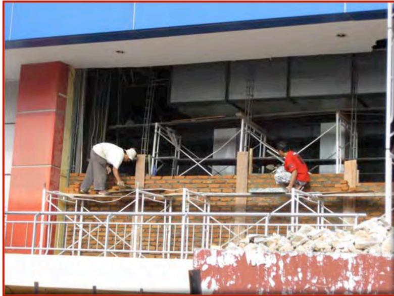
Figure 16. Labourers Rebuilding the Walls of the Ramayana Shopping Centre, Padang.
