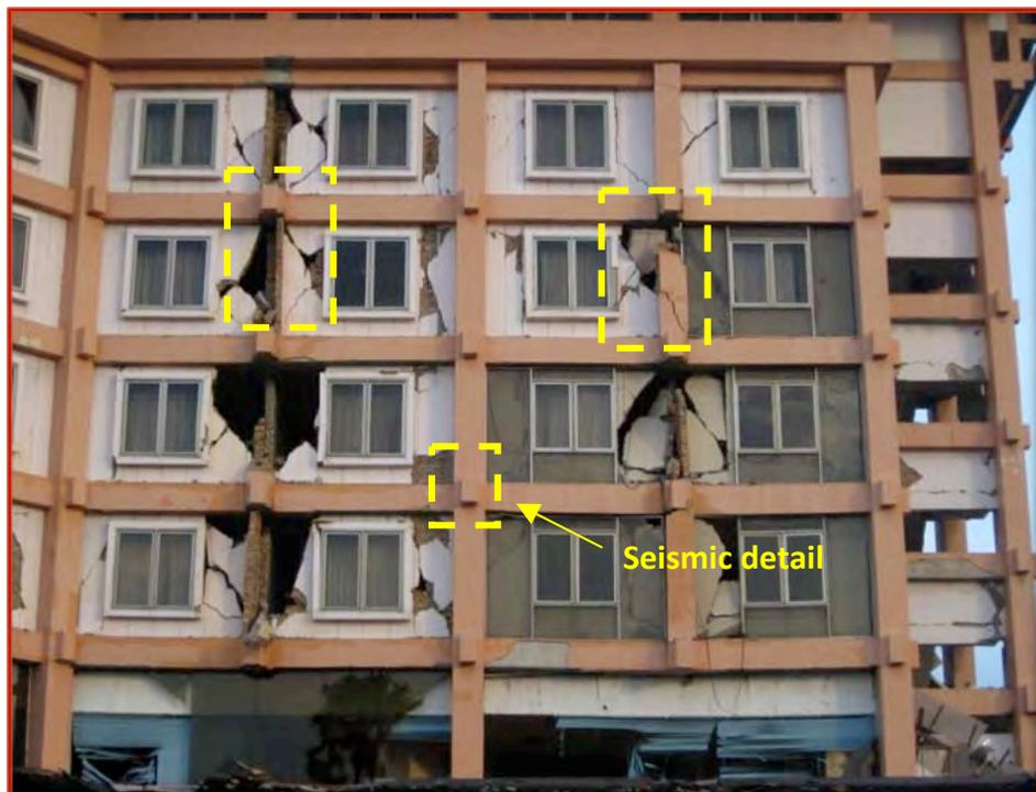
Figure 30. Bumiminang Hotel, shear cracking and damage to false masonry columns.
