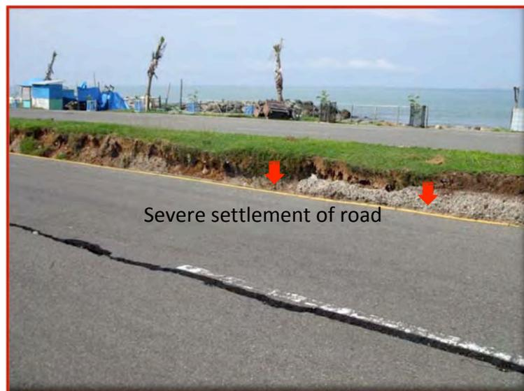
Figure 54. Settlement and cracks on road parallel to the coastline.
