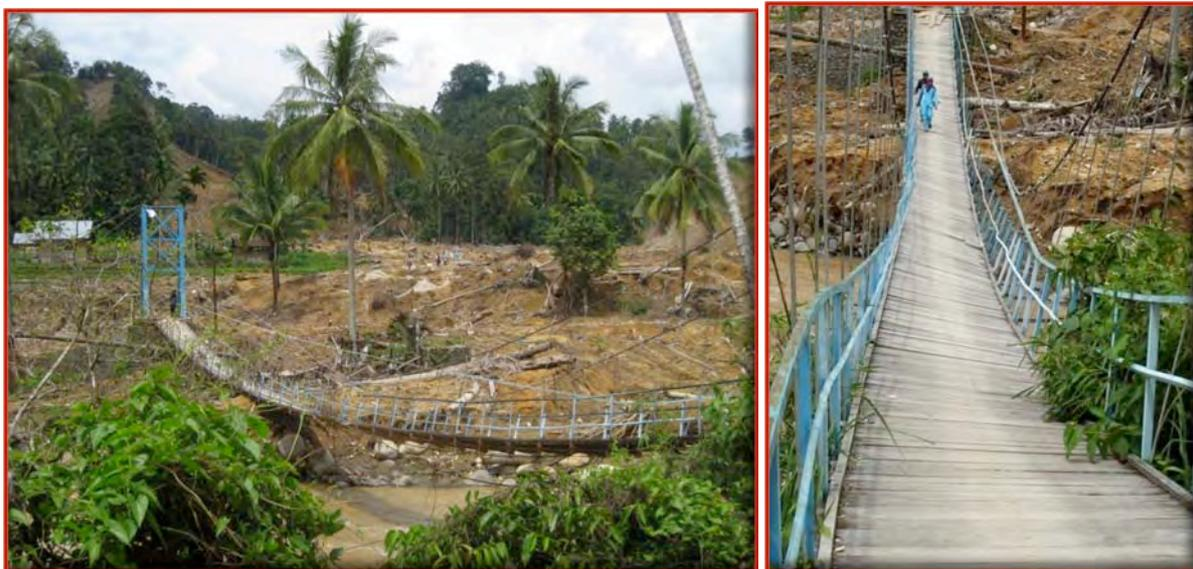
Figure 70. Damaged pedestrian bridge still frequently used by residents.
