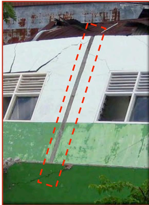
Figure 46. Location of wall to wall joint – no connection between orthogonal walls.
