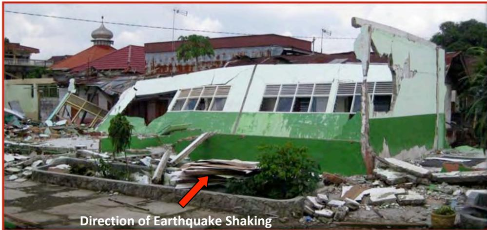
Figure 44. SDN 24 Ujung Gurun Elementary School in Padang – collapsed building.
