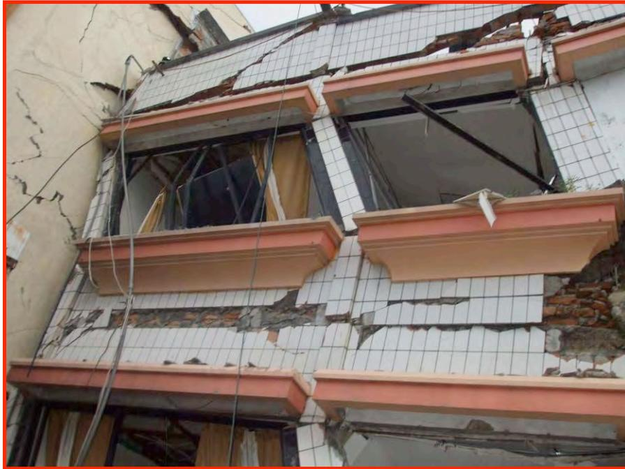
Figure 25. Plastic hinging at column ends of reinforced structure.
