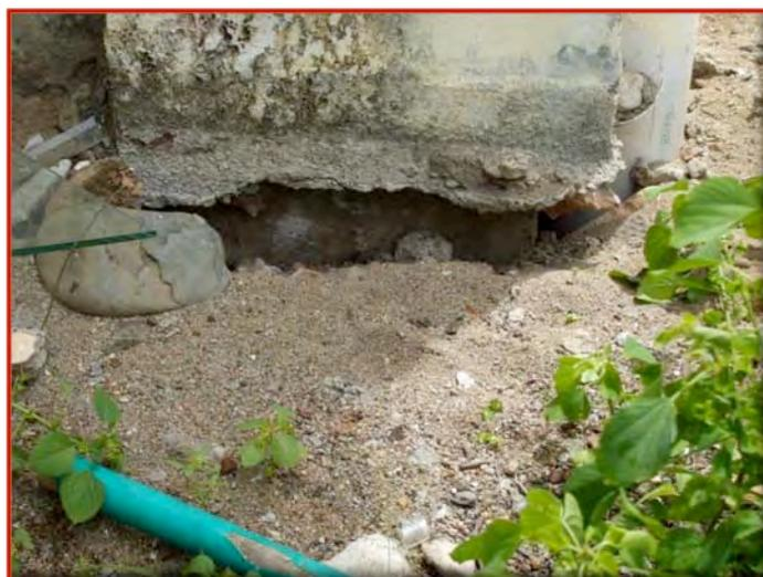
Figure 59. Settlement of soil around a column of a university building.
