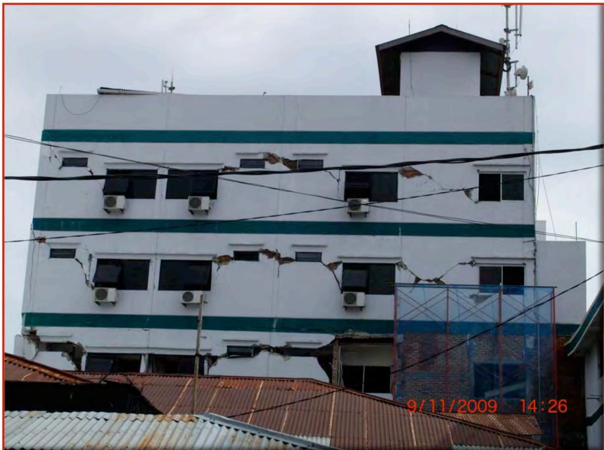
Figure 51. Bunda Medical Centre showing extensive cracking of non-structural masonry.
