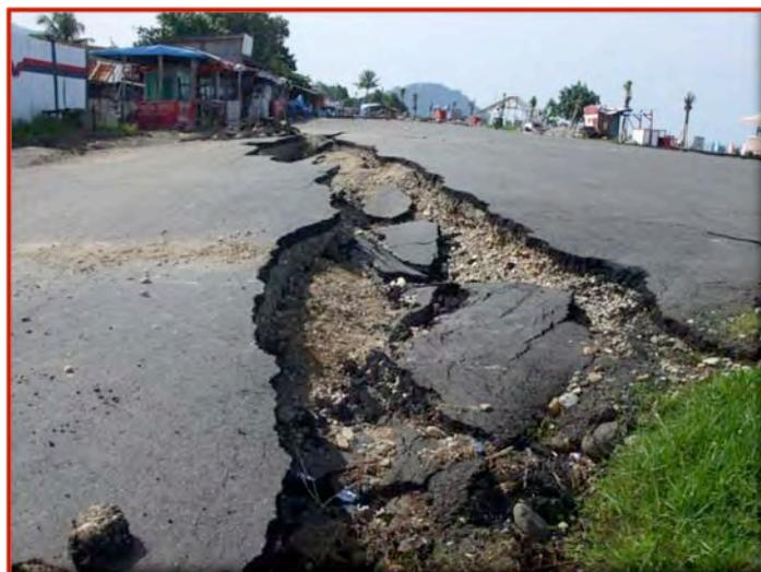
Figure 56. Severe failure of road at the crest of the embankment.
