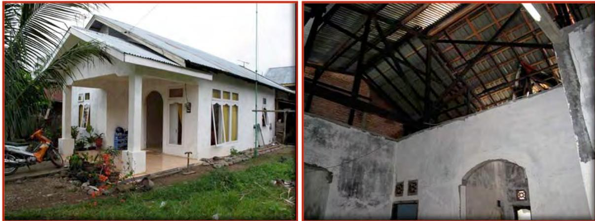
Figure 18. Left: Typical one storey house made of confined masonry (photo taken in Padang). Right: typical configuration of residential roofs.
