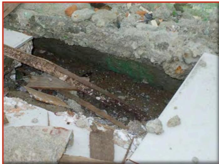
Figure 61. Wall collapse due to insufficient embedment of strip foundation.
