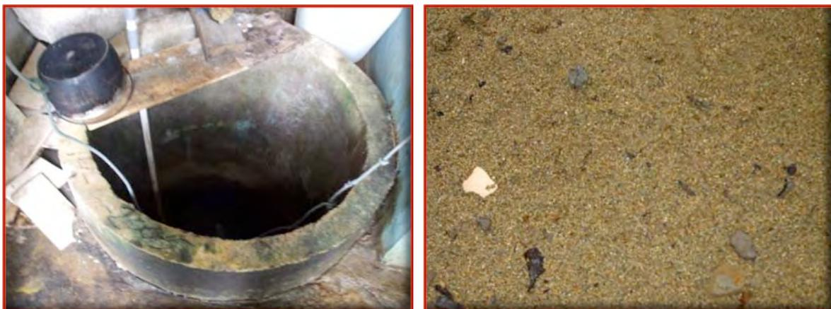
Figure 73. The well (left) that was blocked with sand (right) due to liquefaction.
