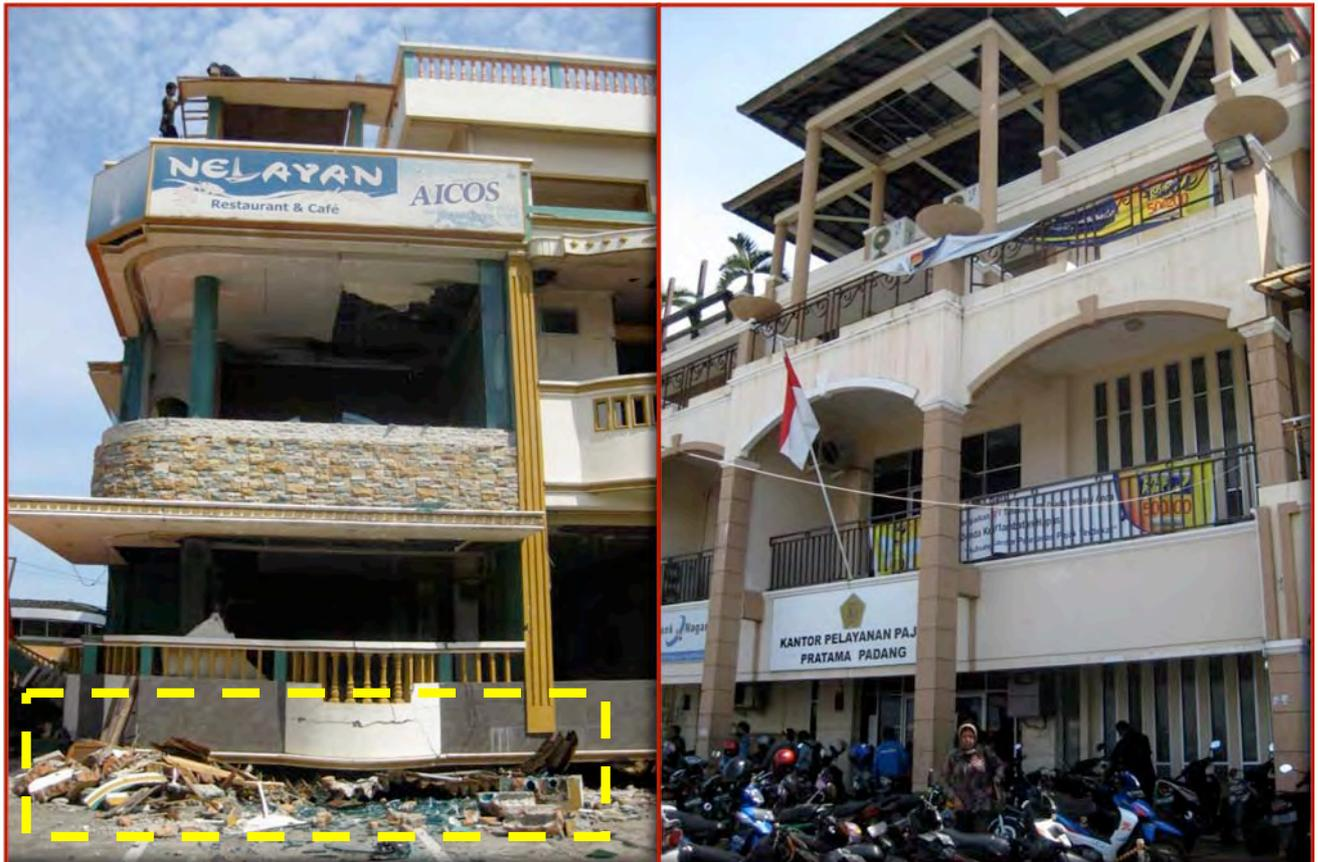
Figure 31. Small Shopping Centres; Left: soft-storey failure, Right: Minimal damage.
