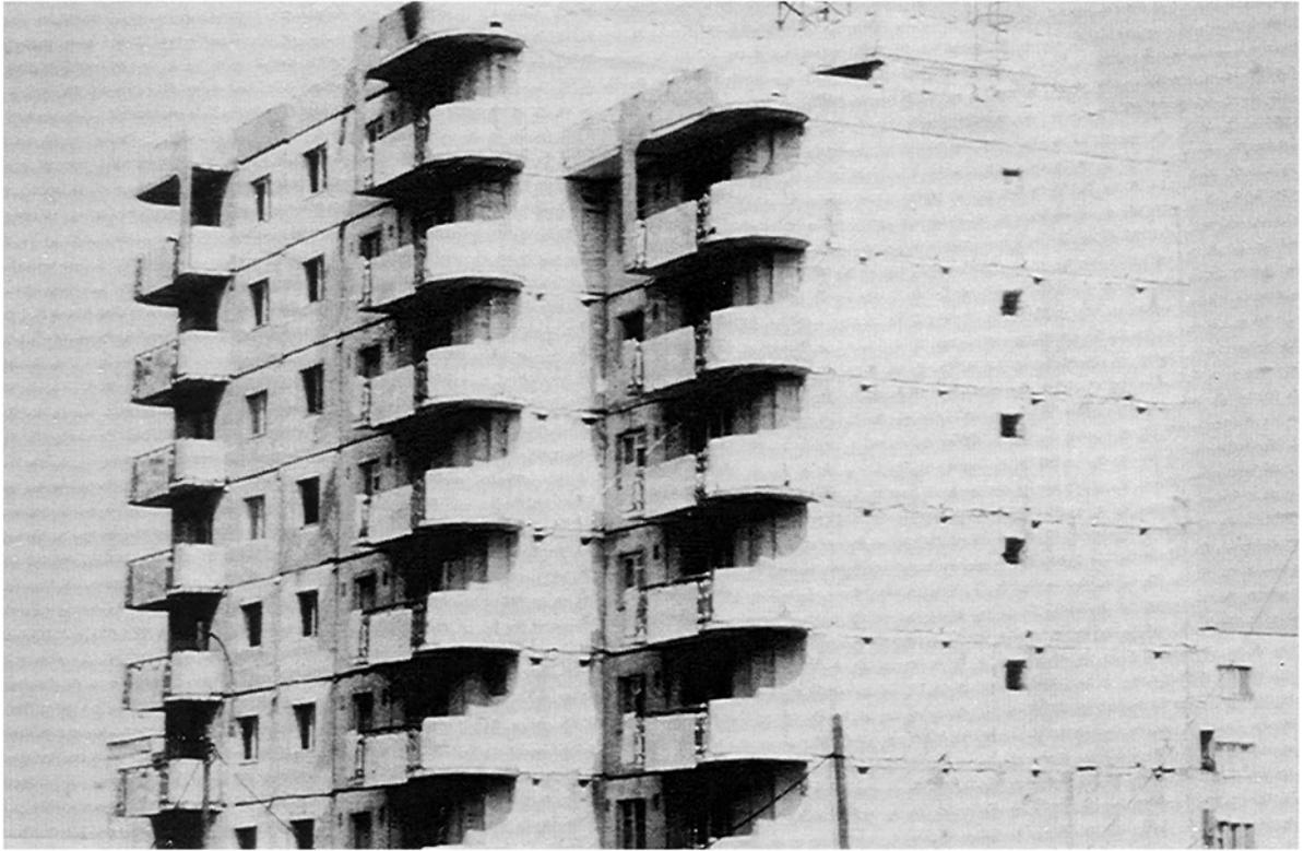
Plate 18: RC large panel construction before plastering. Notice the poor details in the connections.
