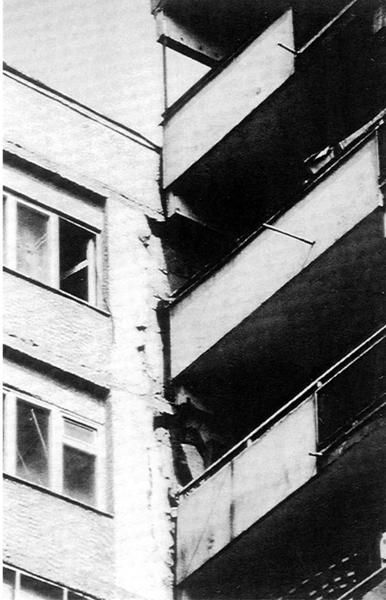
Plate 28: Close view of the damage due to pounding between the two structural parts of different shape and height.
