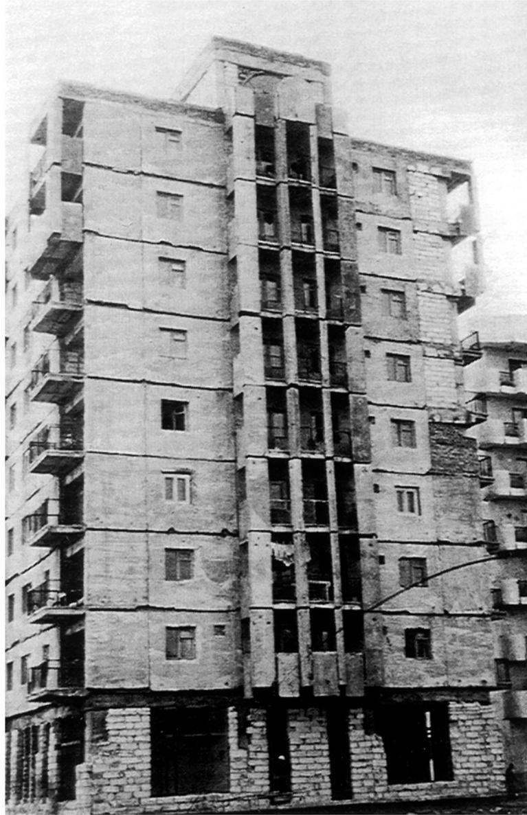
Plate 14: Similar RC frame building in final stage, before plaster is applied (Location: Focsani)
