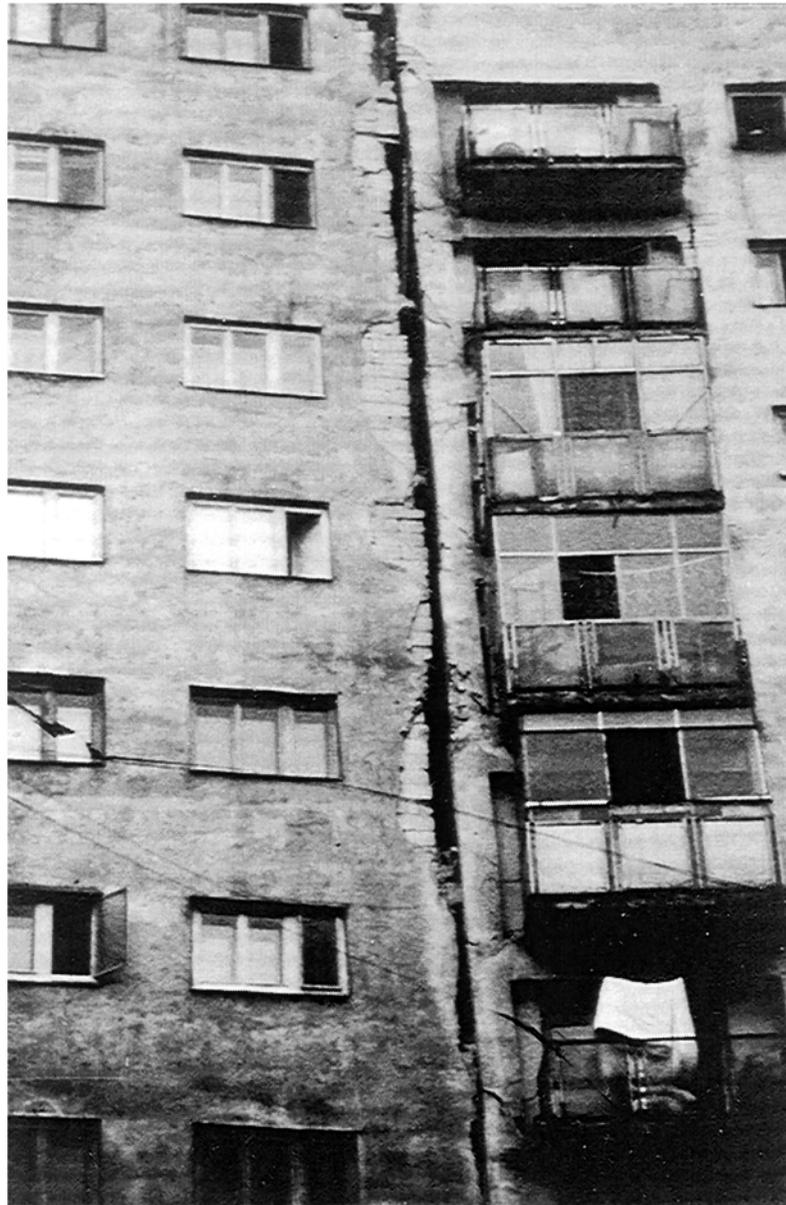
Plate 4: Colentina district, damage down the seismic gap line, due to pounding.
