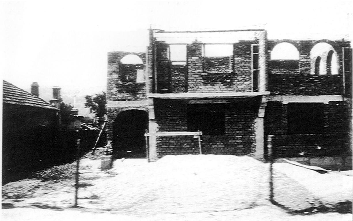
**Plate 11: Two storey reinforced brick masonry house. Notice the reinforcing bars in the top floor and columns in the ground floor.**
