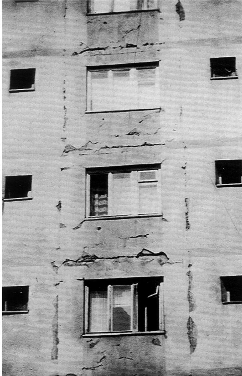
Plate 25: Widespread cracks around the panel perimeter (Location: Ploiesti survey)
