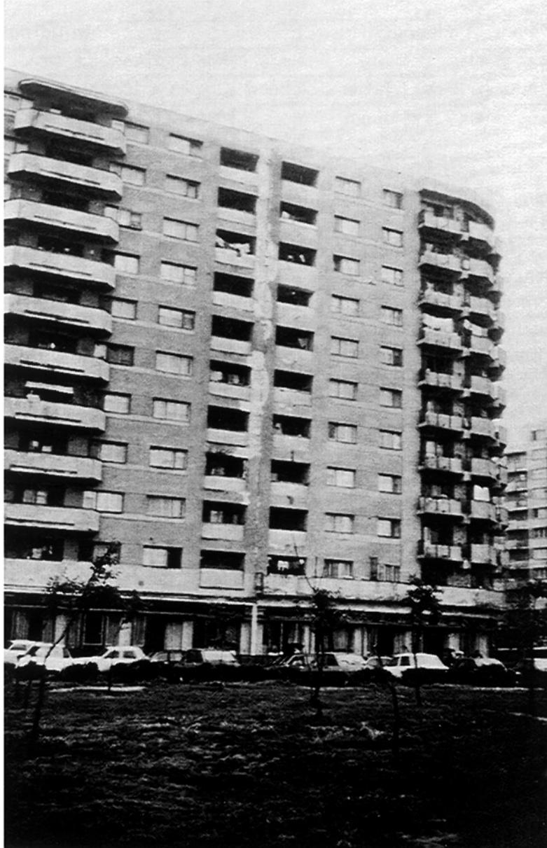
**Plate 1: General view of the apartment building Colentina no. 81, Block 84/I. This is where the two Bucharest fatalities occurred due to the collapse of the plasterboard along the seismic gap, as a result of pounding between the two structural parts of the large complex.**
