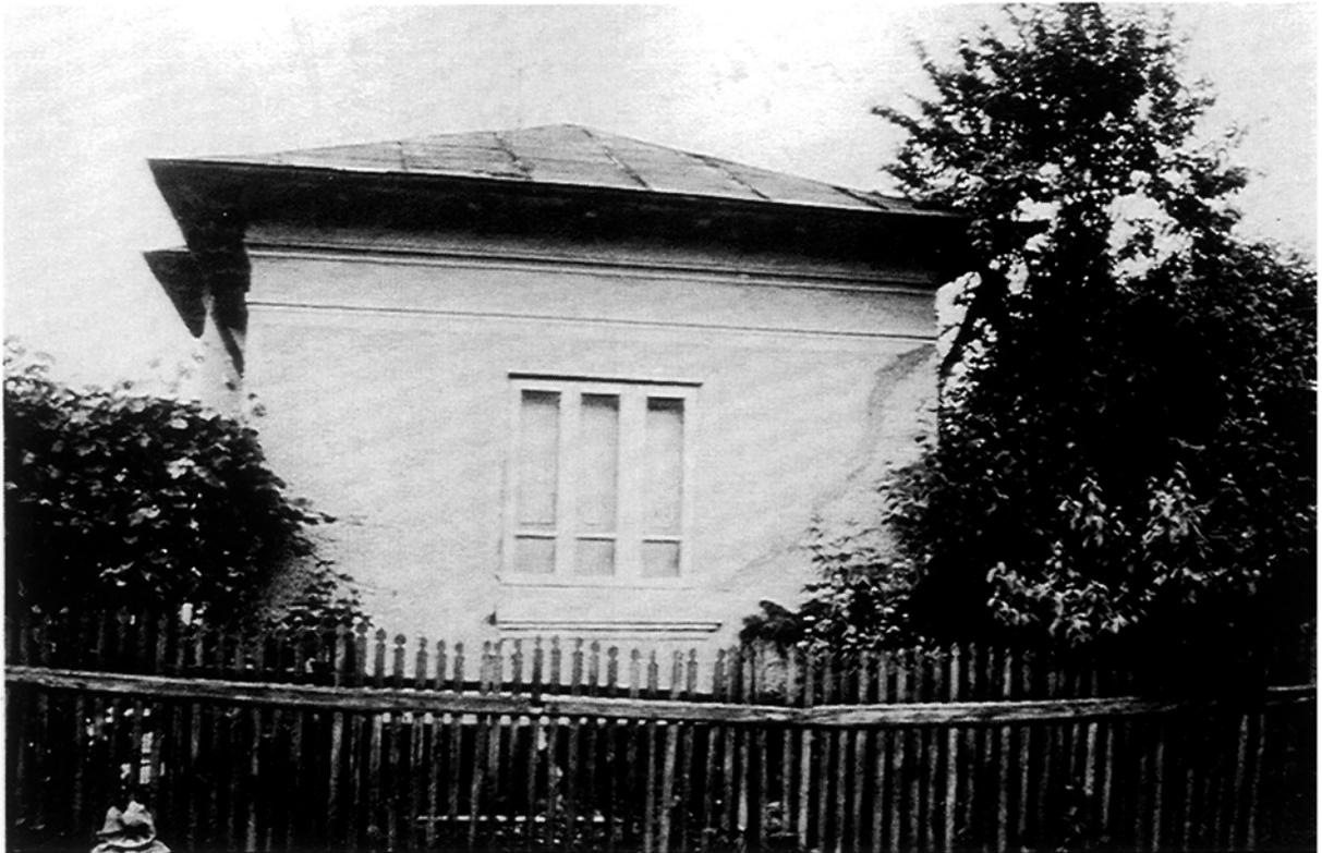
Plate 21: Evidence of repairs after the 1986 earthquake was widespread (Location: Buzau survey).
