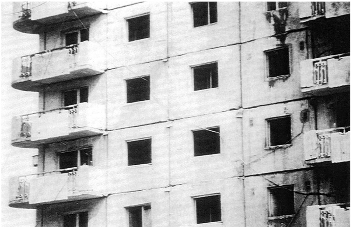
**Plate 17: Detail of connections in an RC large panel building under construction.**
