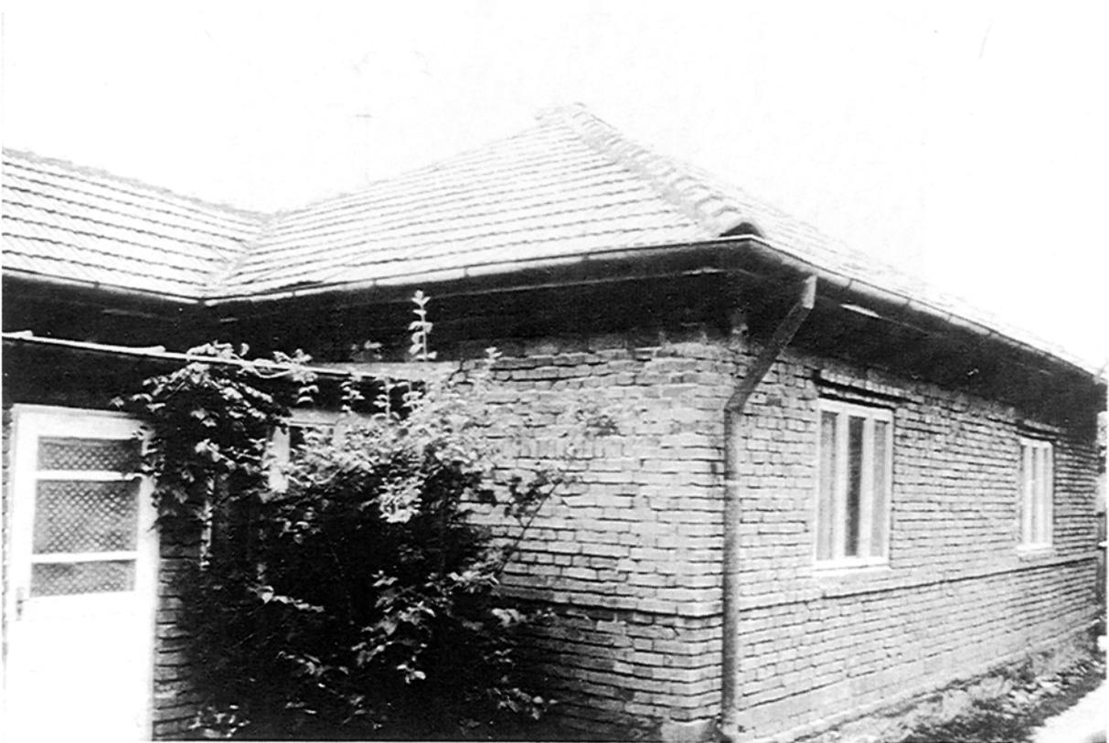
Plate 8: Typical single storey unreinforced brick masonry in cement-lime mortar.
