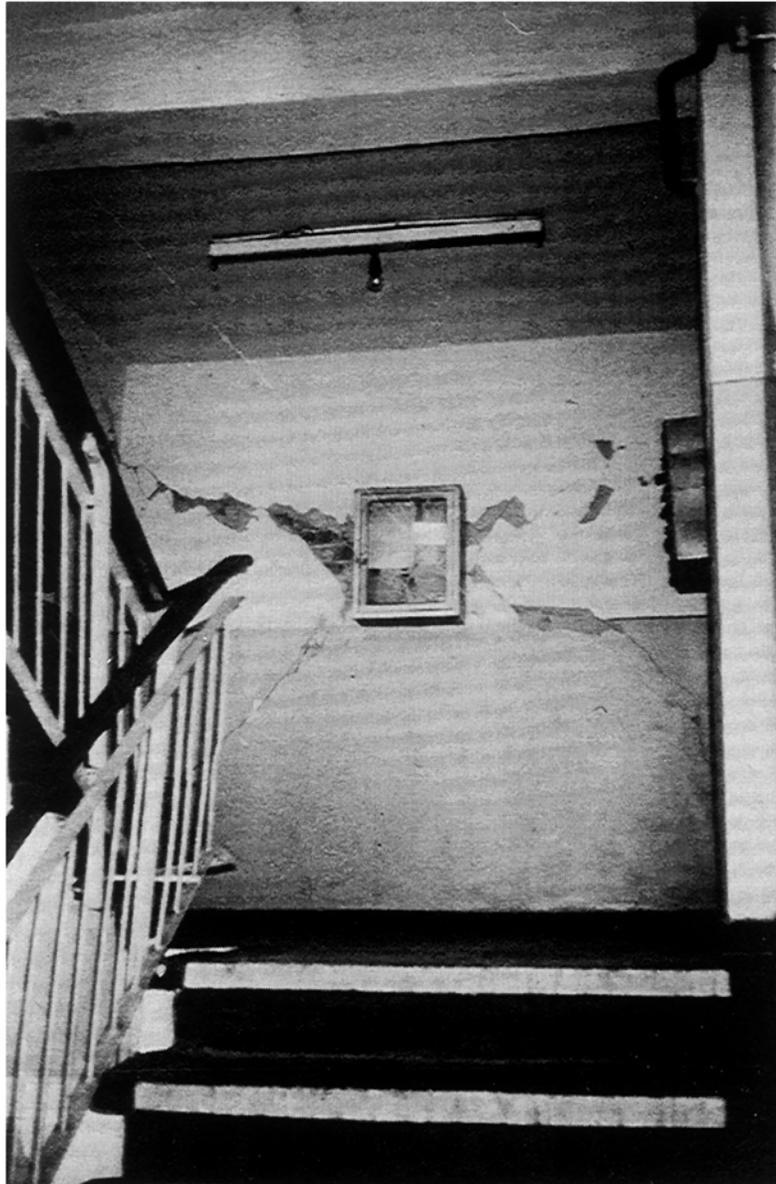
Plate 26: Diagonal cracks in the infill masonry (Location: Buzau survey).
