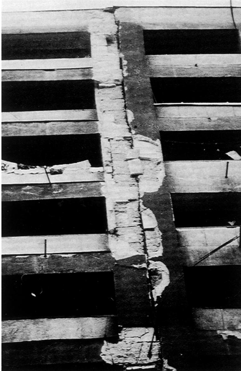
Plate 2: Close view of the collapsed plasterboard along the seismic gap line.
