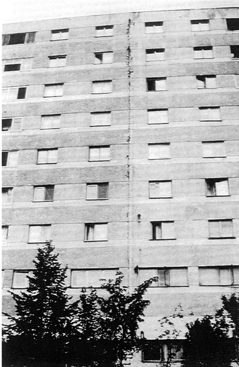
Plate 24: Damage to the expansion joint (Location: Buzau survey).
