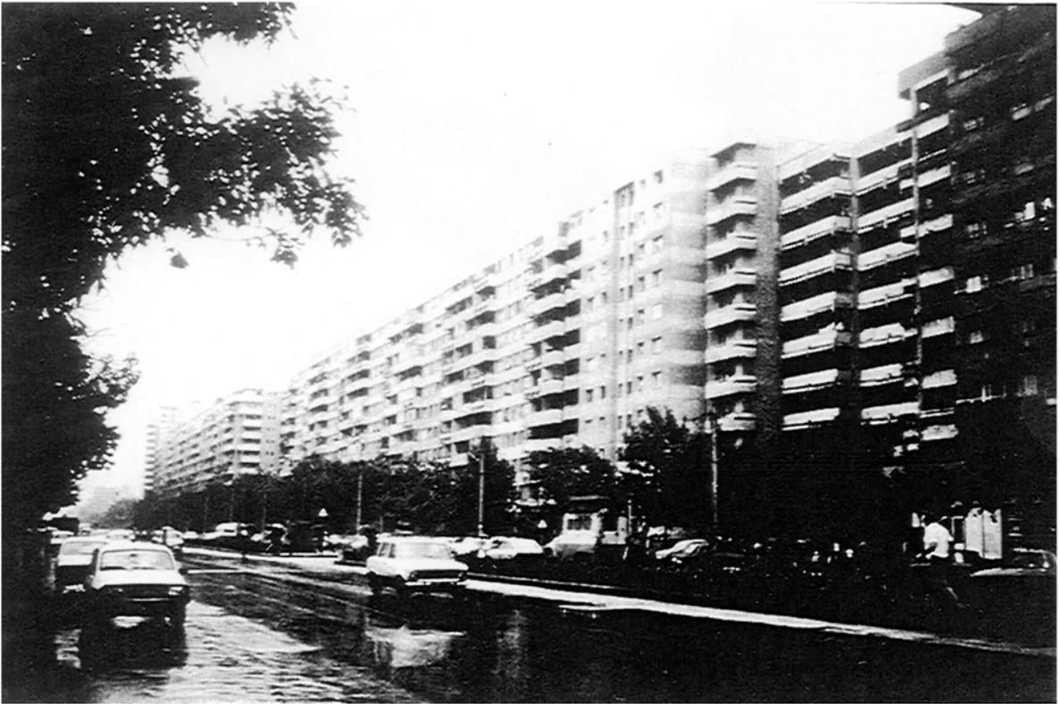
**Plate 16: Typical RC with shear walls large apartment block with several expansion joints and entrances (Location: Bucharest).**
