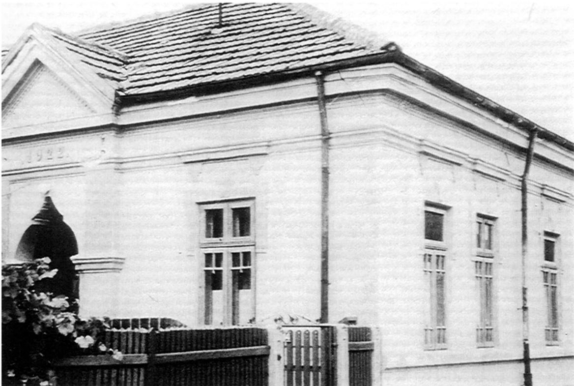
Plate 19: Typical single storey brick masonry building in the Buzau survey.
