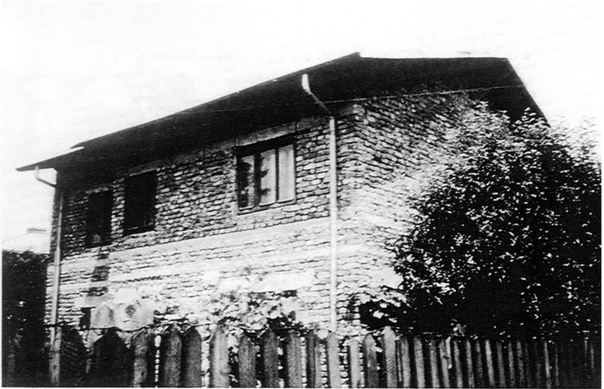
Plate 9: Two storey brick masonry house with RC slab, RC lintels and ring beam in the ground floor.
