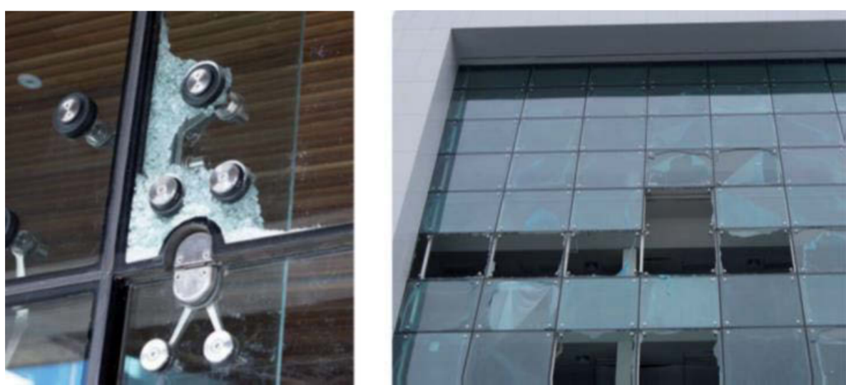
Figure 1: Damage of bolted connected façade elements in 2011 Christchurch earthquake New Zealand (Baird et al., 2012)
