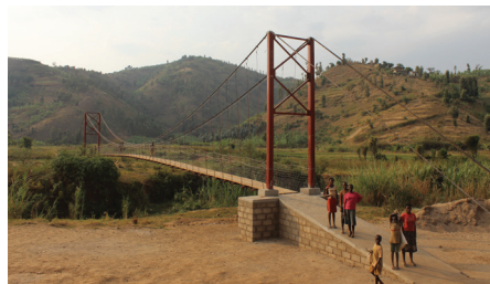
Figure 2 The 50m main span Muregeya Bridge was built with the help of Rwandan engineering students and local support
