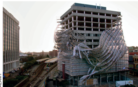
Figure 1 Fanum House scaffold collapse
