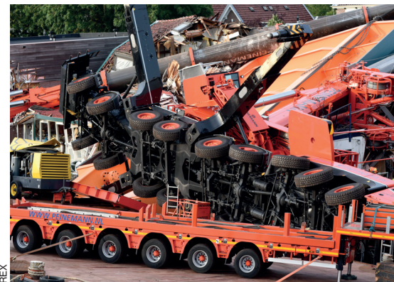
Figure 2 Queen Juliana Bridge crane collapse
