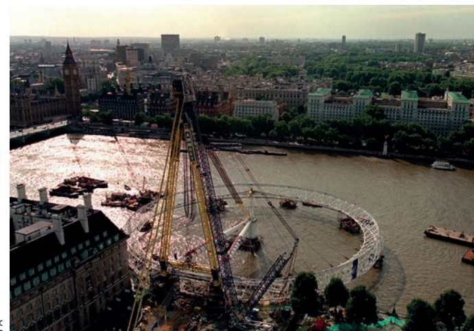
Figure 5 Shear legs used to lift London Eye into position
