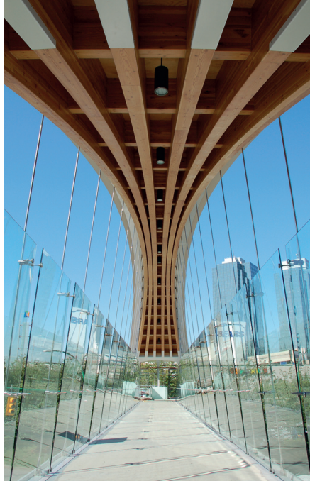
Figure 4 Kingsway Pedestrian Bridge
