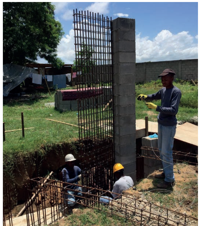
↘ Chapel was erected using local labour
