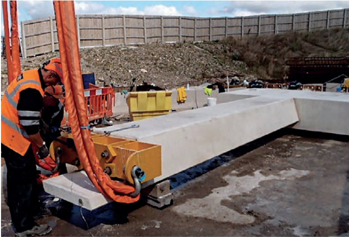
Figure 17 Victoria Dock Road column/ wall structures
