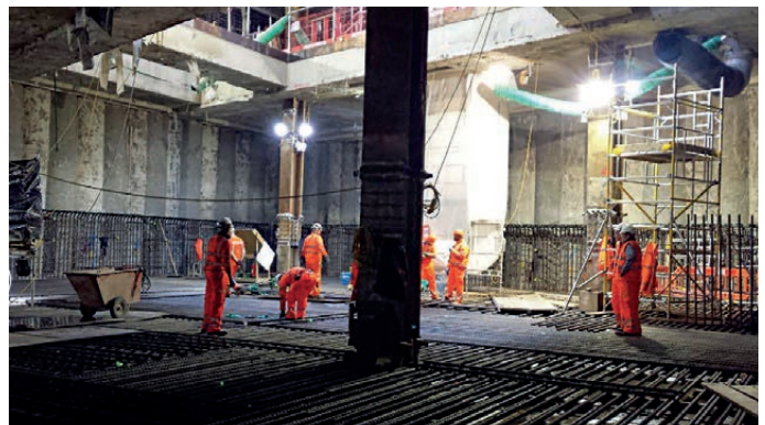
Figure 16 Construction of East Ticket Hall base slab (Level -7) (plunge column exposed)
