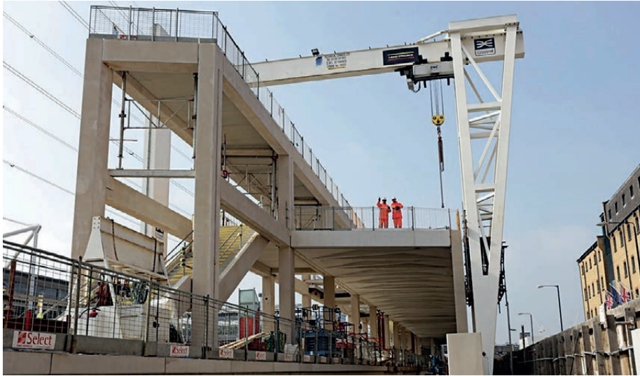
Figure 20 Custom House station used 880 precast units
