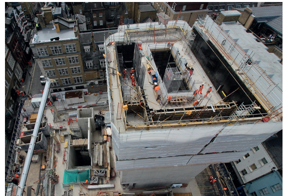
↻ Figure 9 Western Ticket Hall superstructure with climbing formwork
