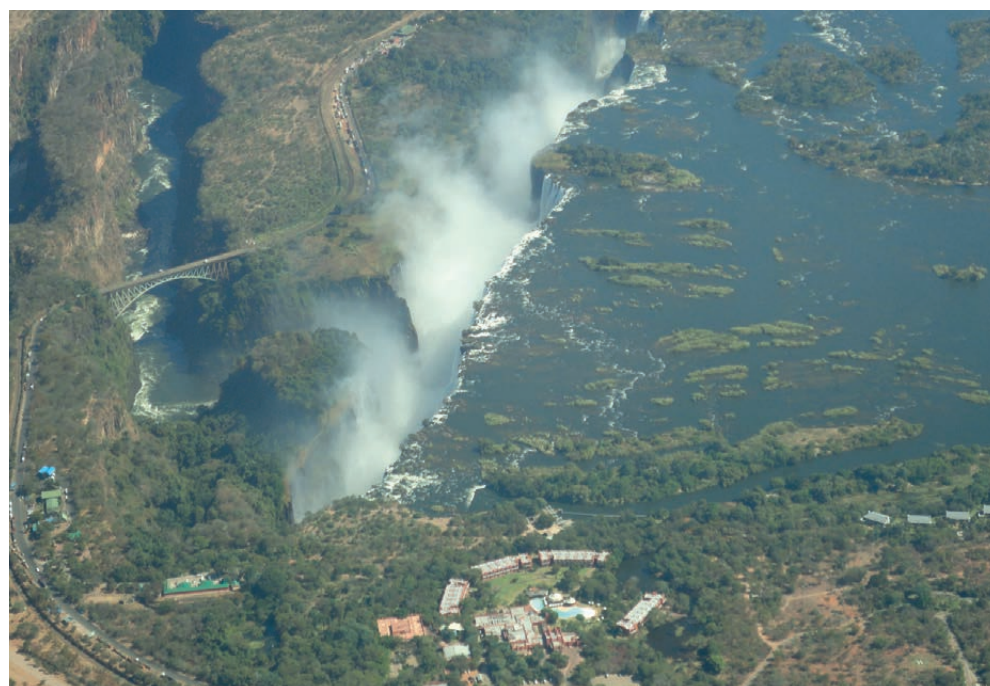
↓ FIGURE 7: Victoria Falls Bridge, Zambia
