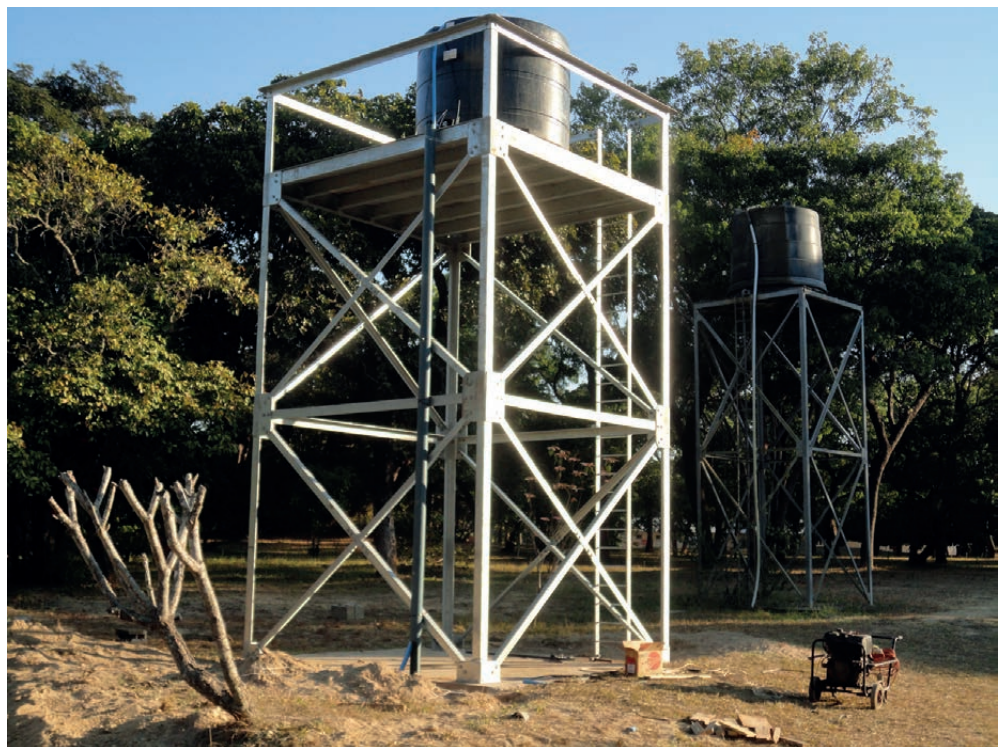
▲ FIGURE 16: Completed water tower, Dupalata
