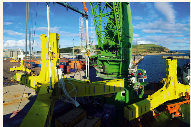
Figure 2 Tripod includes articulated feet with spherical bearings to allow self-levelling and lifting eye for installation
