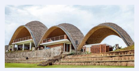
approaches are combined in a permanent structure, with the largest vault spanning 16m with a rise of 8m. The Rwanda Cricket Stadium is a fusion of advanced structural analysis and architectural design with labour-intensive, locally sourced material production offering a much-needed solution to building sustainably in the
