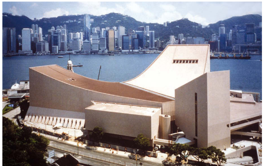
FIGURE 3: Cable and concrete roof for Hong Kong Cultural Centre, 1986
