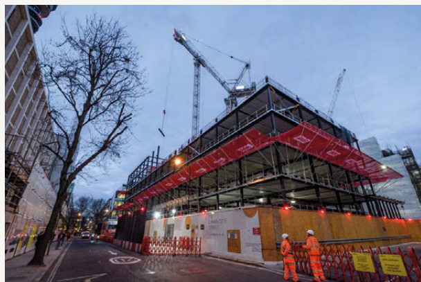
FIGURE 6: Office building with a 90-minute fire resistance period and is provided with intumescent paint pigmented with a dark grey colour
