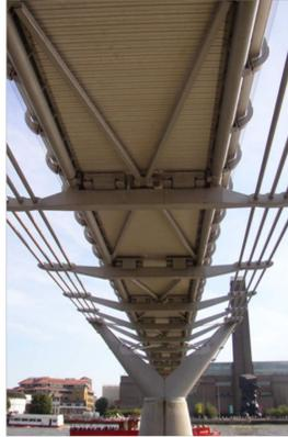
Fig 1 - Millennium Bridge retrofitted with damping devices beneath the deck.
