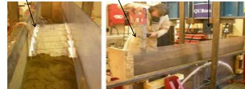
Backfilling the skew FlexiArch
