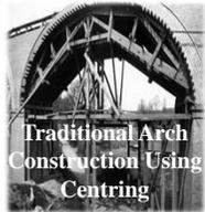
Traditional Arch Construction Using Centring
