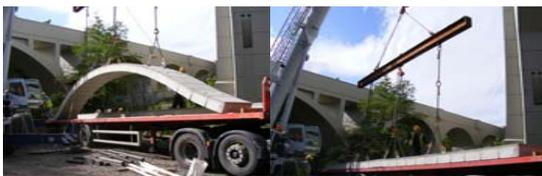
FlexiArch - From flat-pack to arch unit in a matter of seconds
