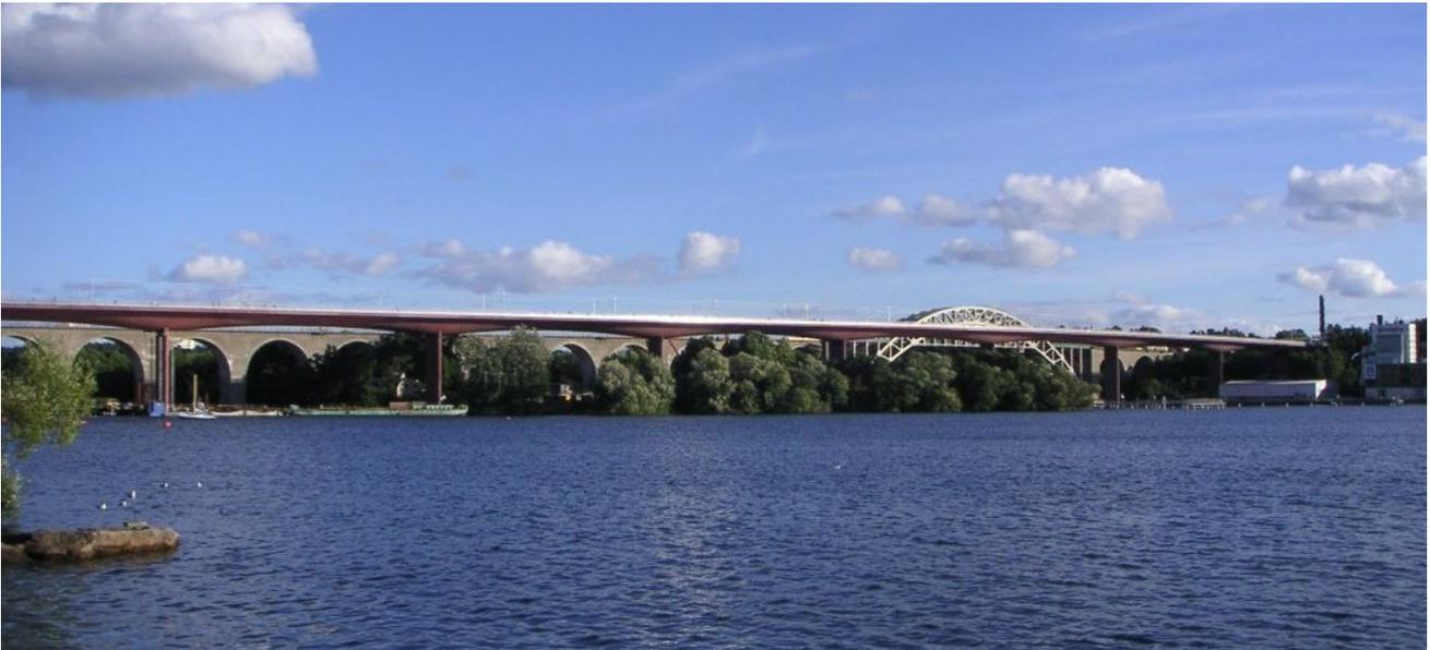
Competition winning design for a new 810m long railway bridge over the Arsta Straits in central Stockholm. The viaduct is a dramatic visual statement with its 3D curved prestressed concrete shell in red concrete rising above the track level which contains much of the rail noise which is a key issue at this site and it naturally provides a 4m wide raised deck to act as the required cycleway. Opened in 2005.
