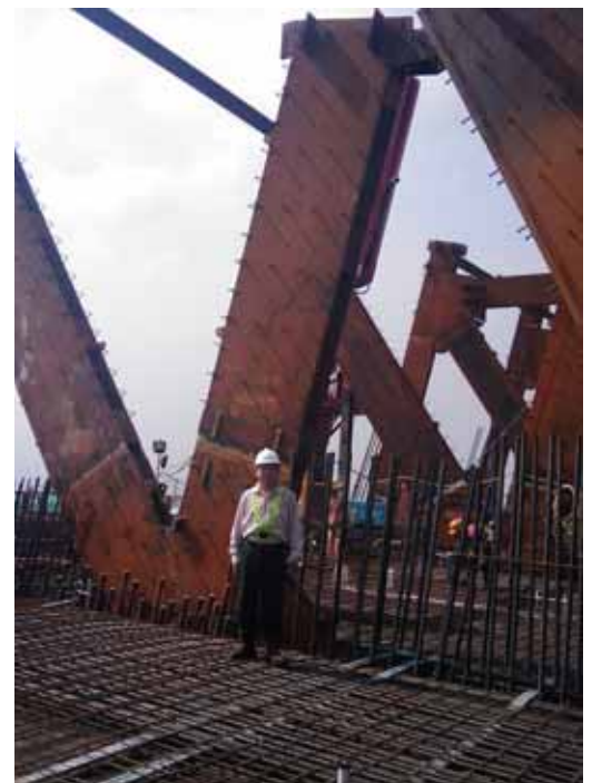
For scaling effect, the size of the 26 th floor transfer truss of MBS Hotel is evident
