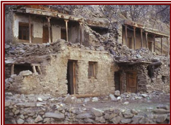
Figure 4: Major epicentral damage of the terraced mountain housing built with random rubble and mud mortars.
