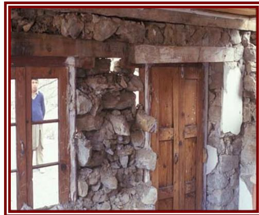
Figure 5: Internal damage to non-load bearing cross walls built in rubble masonry
