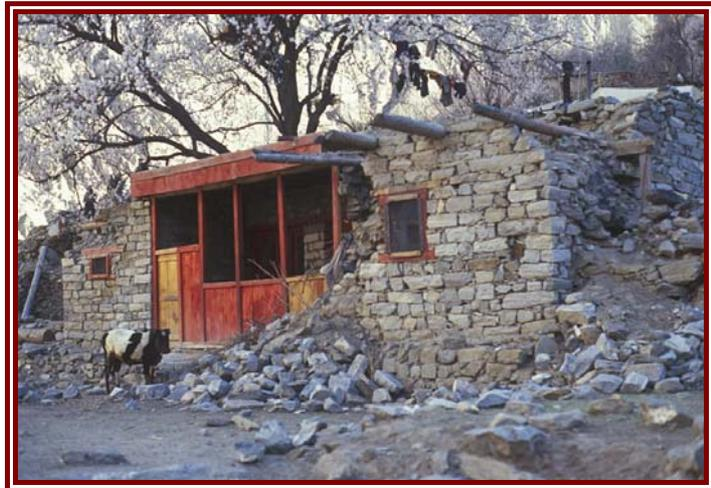
**Figure 6: Load bearing facade survival in new dressed masonry**
