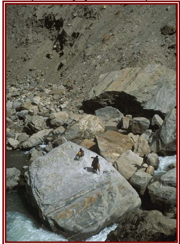
**Figure 3: Breaking up a boulder that had fallen down the mountain side and forming a significant blockage in the river**
