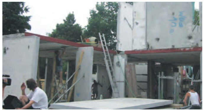
4 Precast panels of the Berlin house
