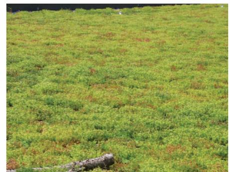
designed accordingly to avoid cold bridging. The growing medium has a tendency to contribute to thermal lag, keeping the building warm at night and reducing heat build up from solar radiation by day.
