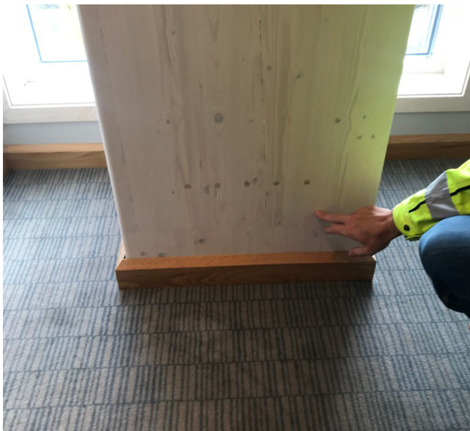
Figure 12: Glulam column on Mjøstårnet. Columns were CNC milled to +/- 1mm tolerance and a flitched steel connection used above floor level to ensure verticality during construction
