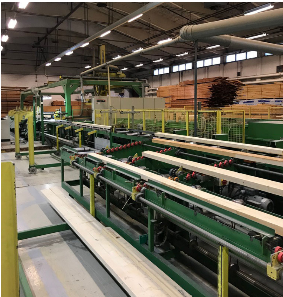
Figure 24: Finger-jointing machinery at Moelven glulam factory, Moelv, Norway
