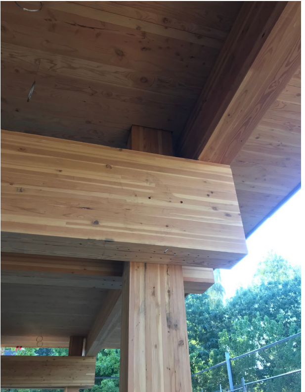
Figure 7: The double-shear connection at the new Adidas HQ in Portland
