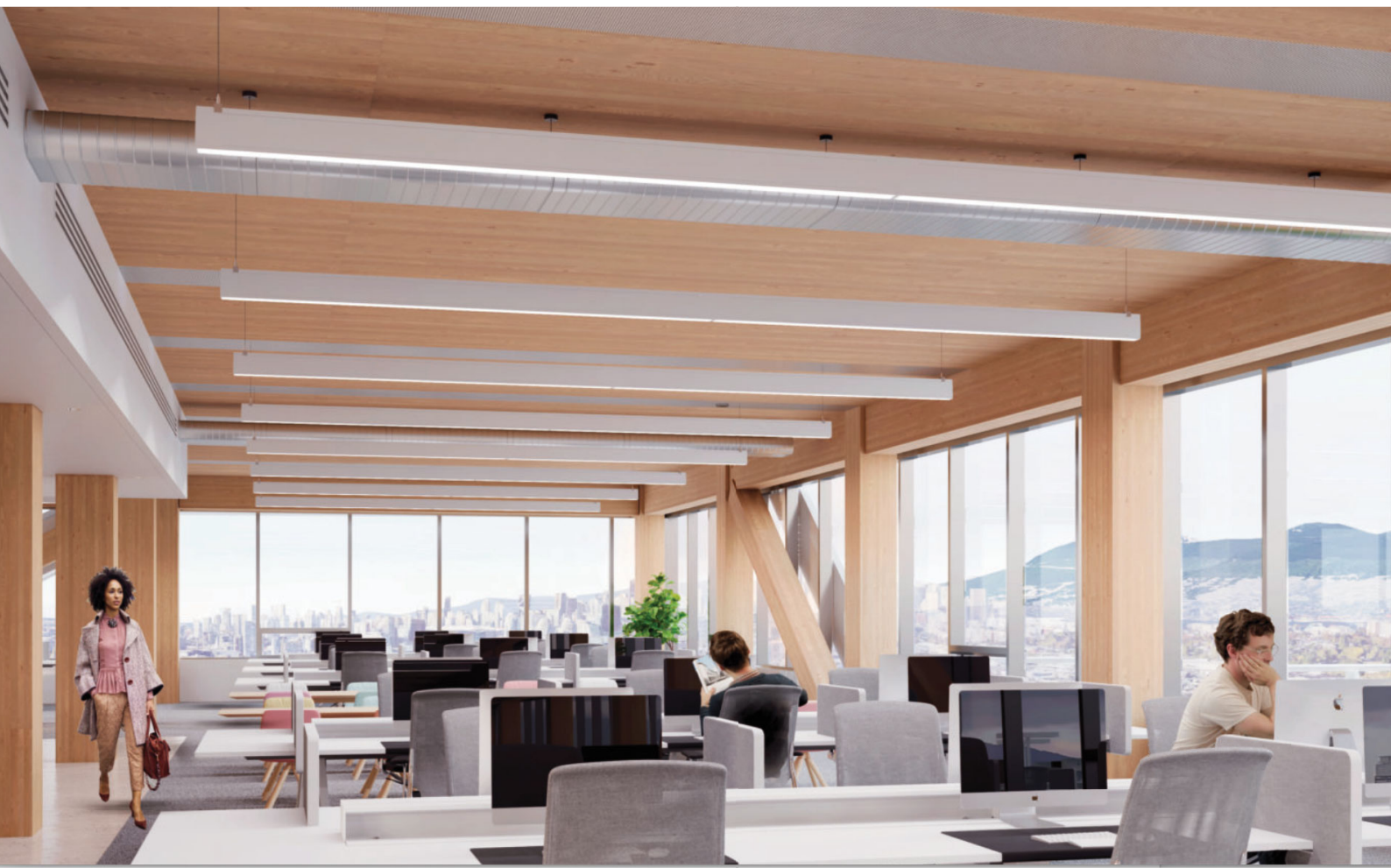
Figure 23: CGI of the flat soffit of Keith Drive, allowing the flexibility of services distribution. Source: Fast & Epp
