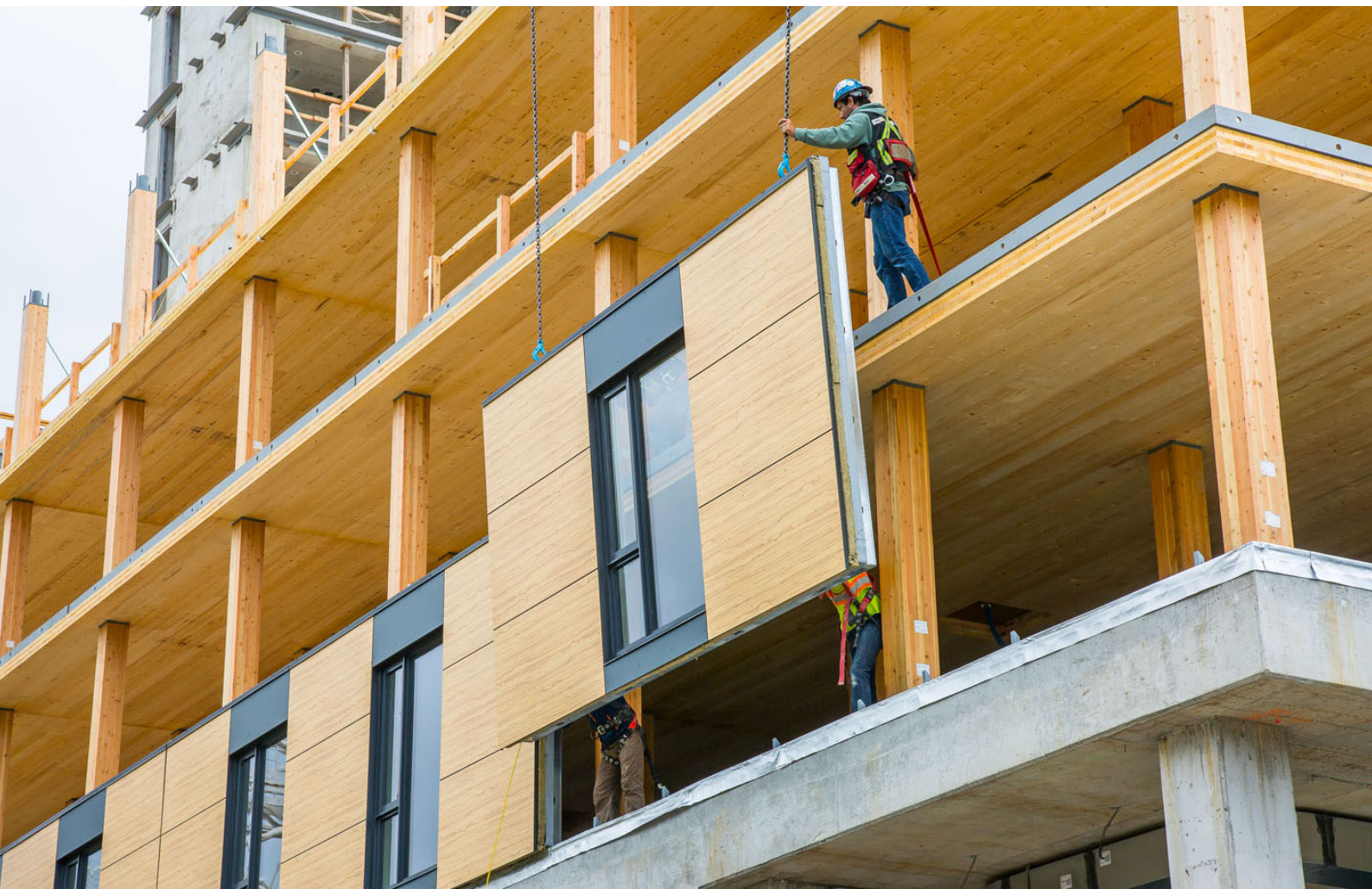
Figure 13: Façade on Brock Commons during construction. Source: Naturally Wood
