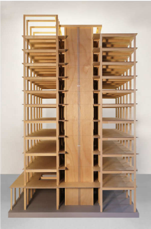
Figure 16: A model of the rocking-wall system on the Framework Building in Portland. Source: Framework Portland
