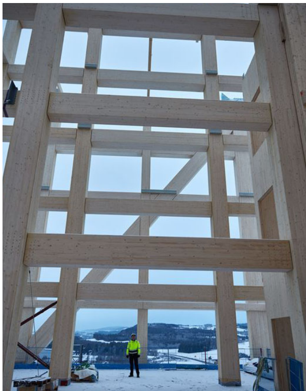
Figure 14: Glulam diagrid on Mjøstårnet during construction. Source: Moelven
