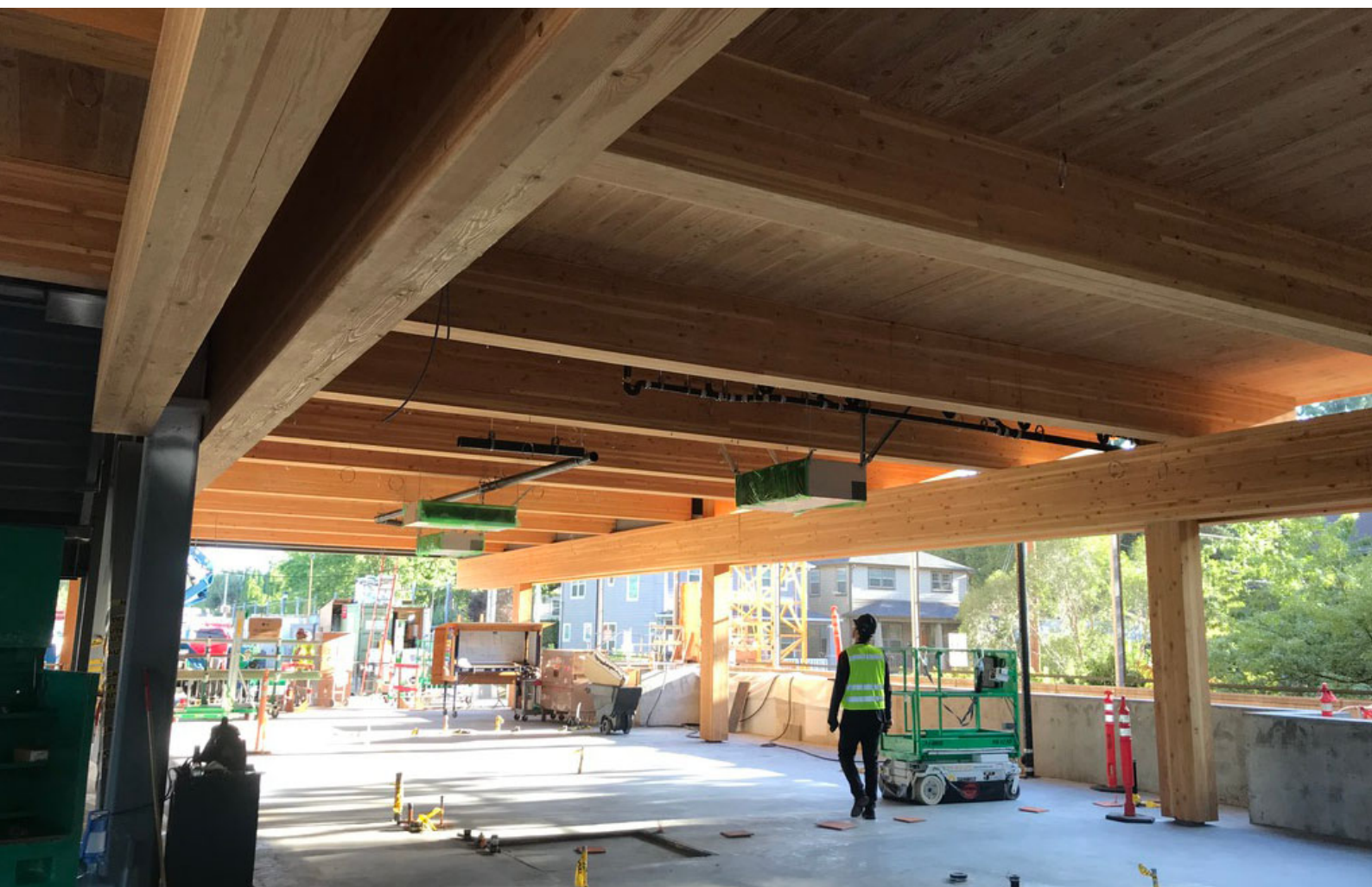
Figure 8: The Adidas HQ typology using two layers of beams for flexibility in internal space and façade arrangement
