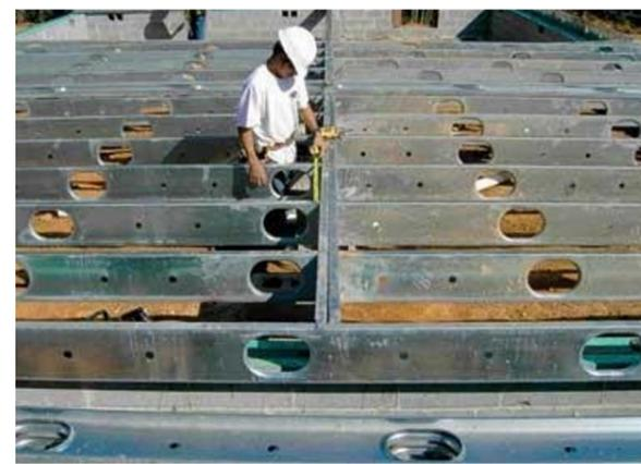
Fig 1 CFS with web openings in flooring and joist
