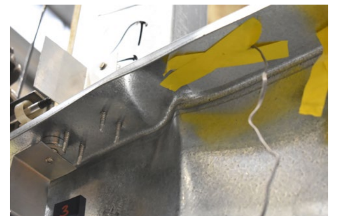
Fig 2 Distortional buckling at joist flange and web
