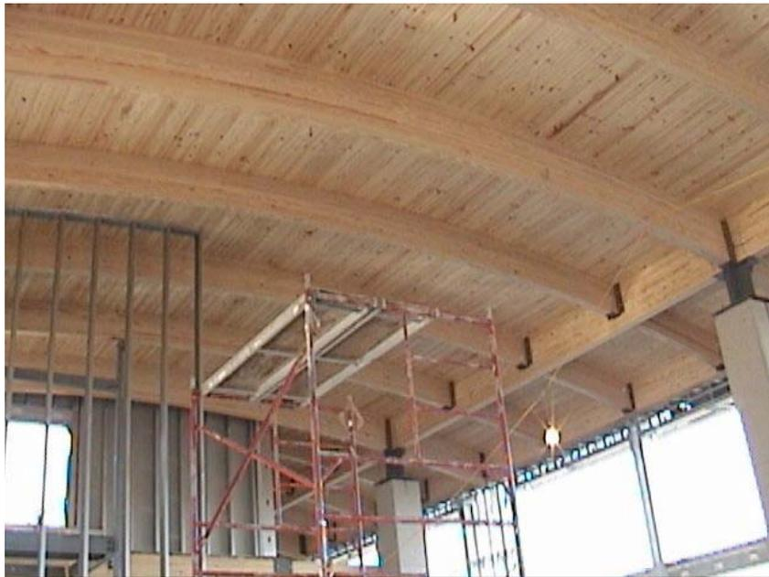
Figure 11. FSC certified wood installed at Missouri DNR
