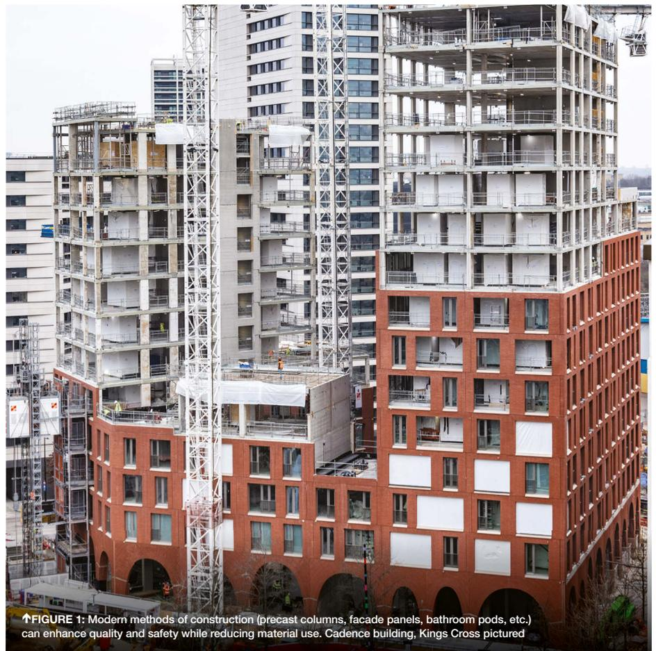
↑FIGURE 1: Modern methods of construction (precast columns, facade panels, bathroom pods, etc.) can enhance quality and safety while reducing material use. Cadence building, Kings Cross pictured
