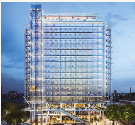
↓FIGURE 2: Paddington Square development, incorporating Farrat TBF structural thermal breaks to isolate feature lift shafts and canopies in fire-protected facade zones
