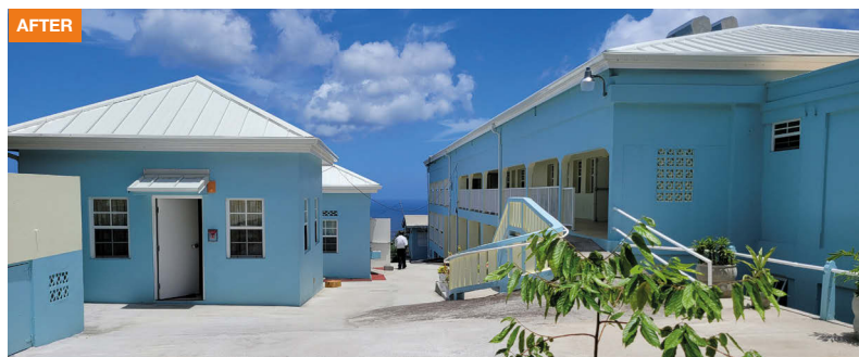
↑FIGURE 4: Smart retrofit of home for elderly in Richmond, Grenada
